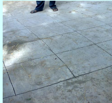
Figure 5 Panel concrete pavement in a village in West Bengal
