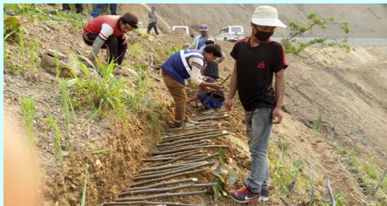
Before: Laying of cuttings in C-Z road
