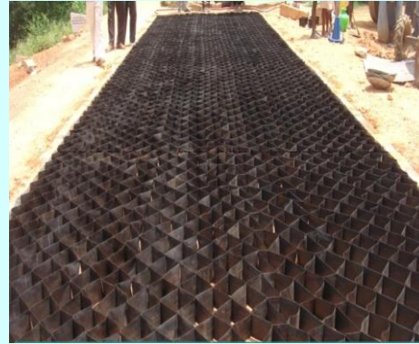
Fig. 6 A view of stretched cell placed over compacted GSB layer
