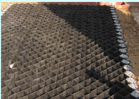
Figure 1 Formwork of cells of recycled plastic.
