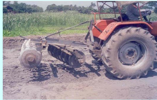
Fig.1. In-situ mixing by using rotavator Fig.2. In-situ mixing by Agricultural Disc Harrow
