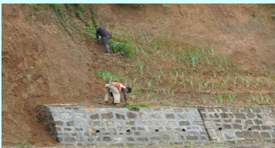
Plate No. 9: Grass slip plantation in between brush layers in C-Z road, Mizoram
