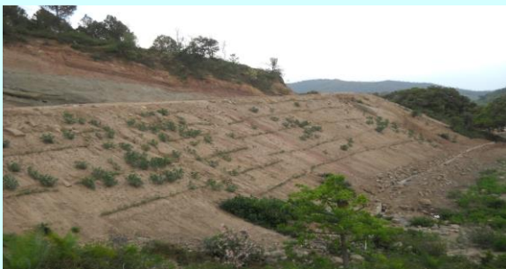
Before: Brush layers with palisades and fascine
