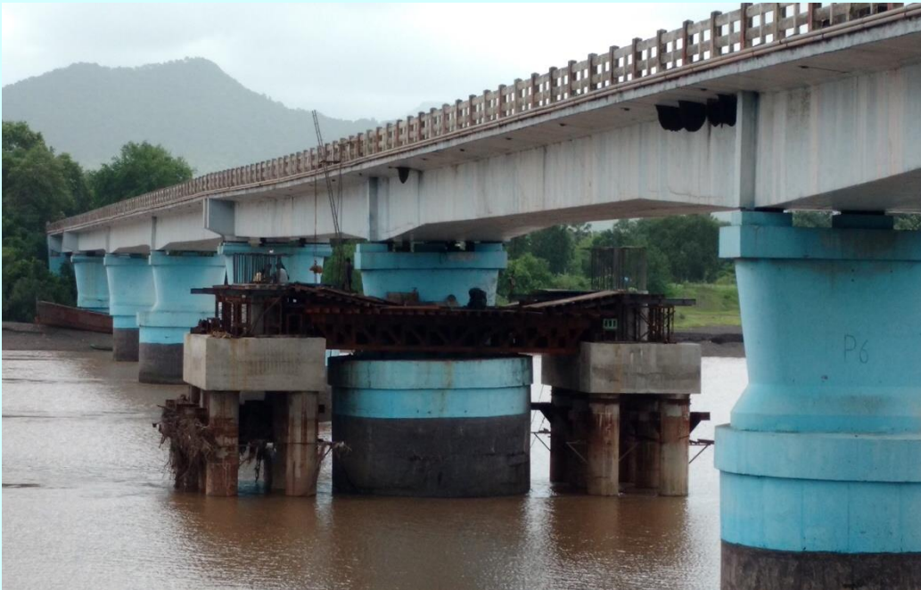
Form work for Portal Beam
