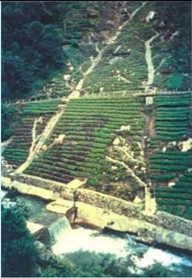
Figure 13: Landslide at Left Bank of Charnawati Valley
