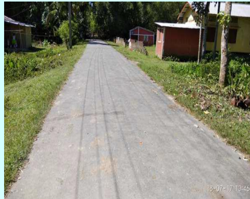
Fig12 Cold Mix Road after Five years
