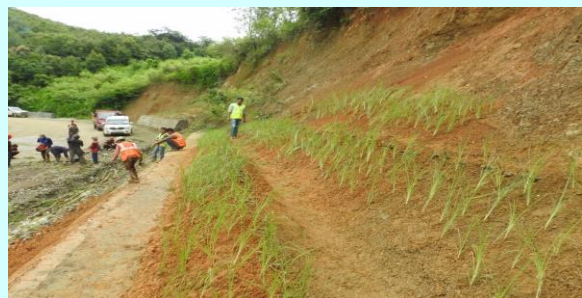
Plate No. 9: Grass slip plantation in between brush layers in C-Z road, Mizoram
