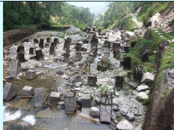
Figure 21: Concrete Armor Blocks After 28 Years
