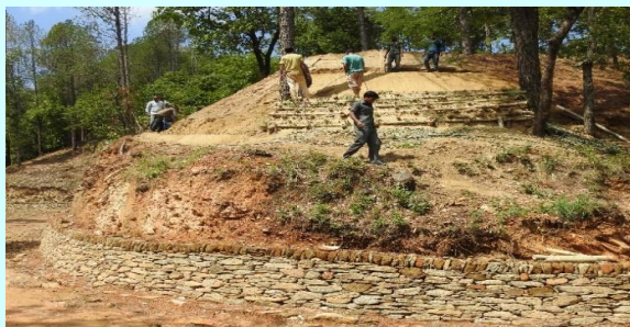
Before: Bamboo crib wall construction
