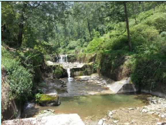
Figure 20: Gabion Check Dams Have Remained Intact After 28 Years
