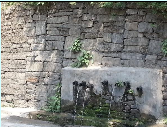
Figure 26: Horizontal Drains Draining Effectively at km 69
