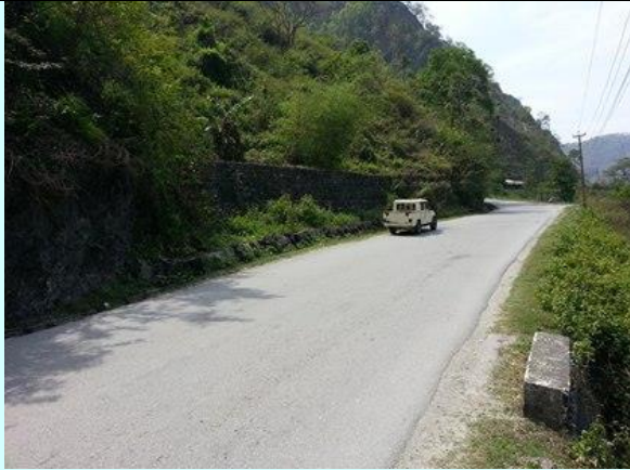
Figure 34: Pavement Condition Intact on Embankment Supported by Soil Nail Wall at km 17
