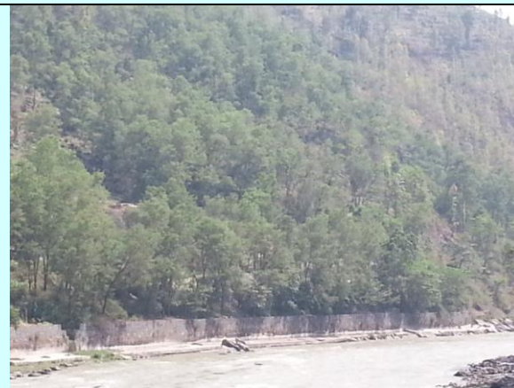
Figure 27: Landslide Converted into Thick Forest. River Training Intact at km 69
