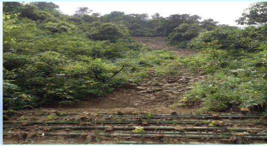
Before: Bamboo crib wall with brush layers, Plate No. 4: Soil bioengineering in Gorkha, Nepal
