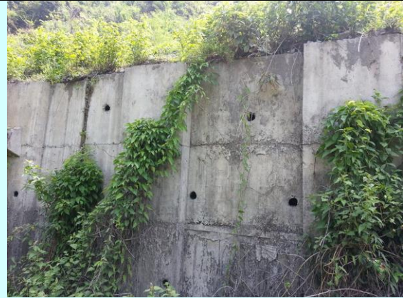
Figure 35: Soil Nail Wall at km 17 Intact
