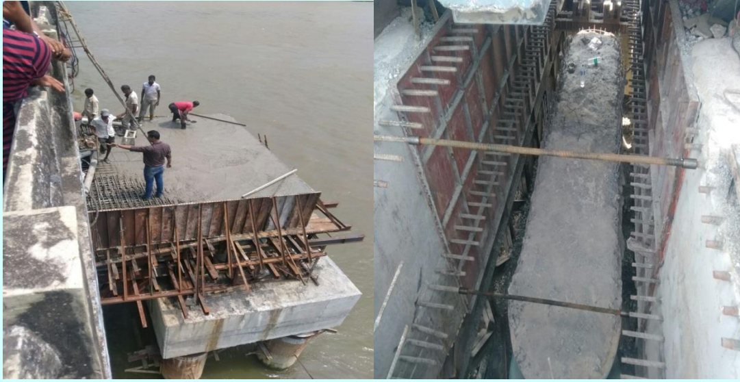
Casting of portal beam
