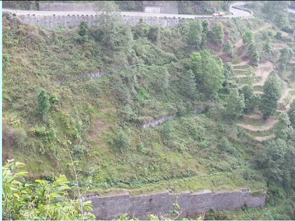
Figure 30: Gabion Toe Wall and Three Tiers of Soil Nail Walls at TN10A
