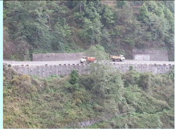
Figure 31: Soil Nailed Wall at Road Edge is Intact at TN10A
