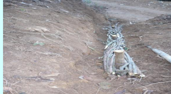
Before: fascines being laid as bundle on rill
