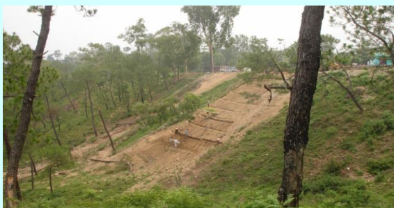
Before: Bamboo crib wall and brush layering techniques
