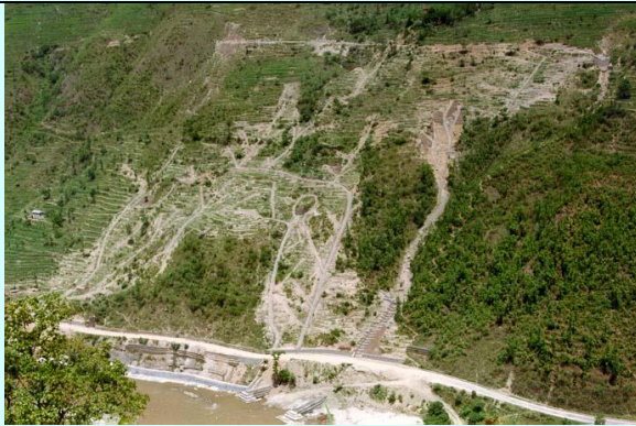
Figure 24: Network of French Drains at km 69
