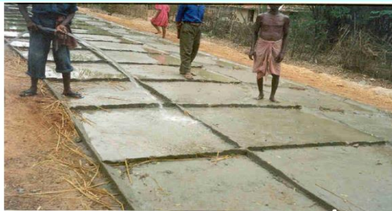
Fig. 7. Curing of concrete
