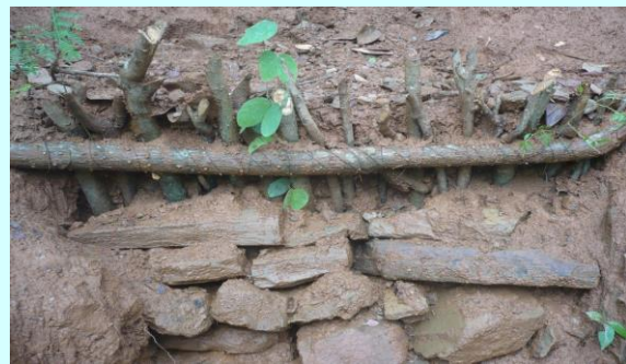
Plate No. 8: Establishment of Palisades in Gorkha for gully stabilization after the earthquake in Nepal
