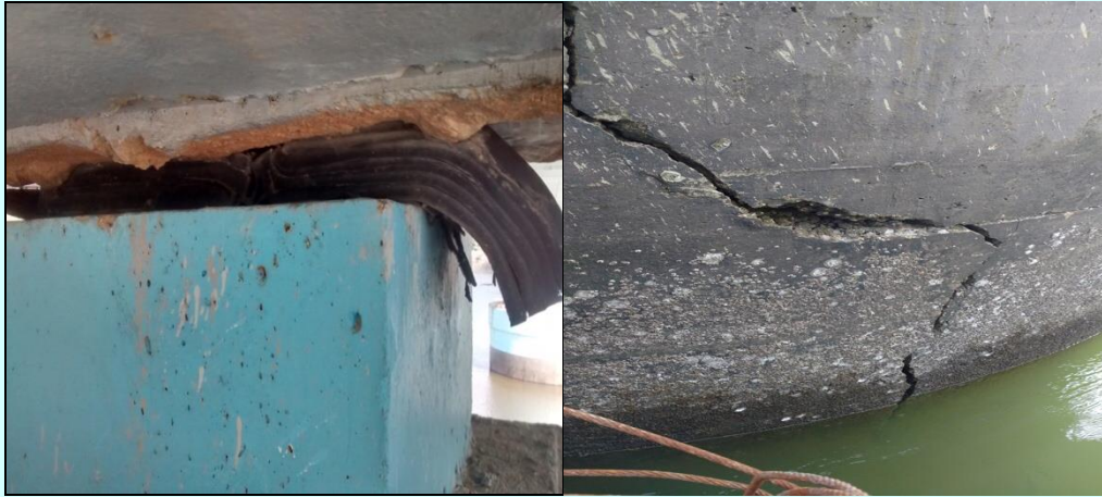
Dislocated Neoprene pad Bearing Crack observed in well
