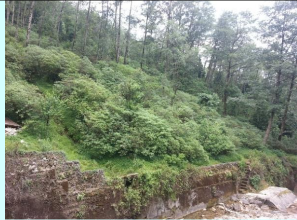
Figure 19: Stabilized Slide Remains Intact After 28 Years
