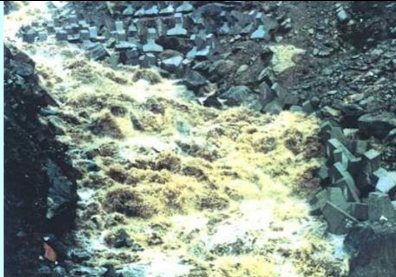
Figure 14: Extensive Use of Flexible Concrete Armored Blocks for Bed Protection
