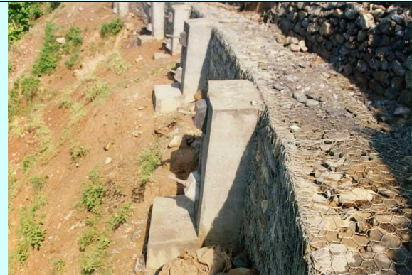
Figure 25: Gabion Wall Supported by Anchored RCC Slices at km 70
