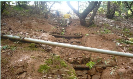
Plate No. 8: Establishment of Palisades in Gorkha for gully stabilization after the earthquake in Nepal
