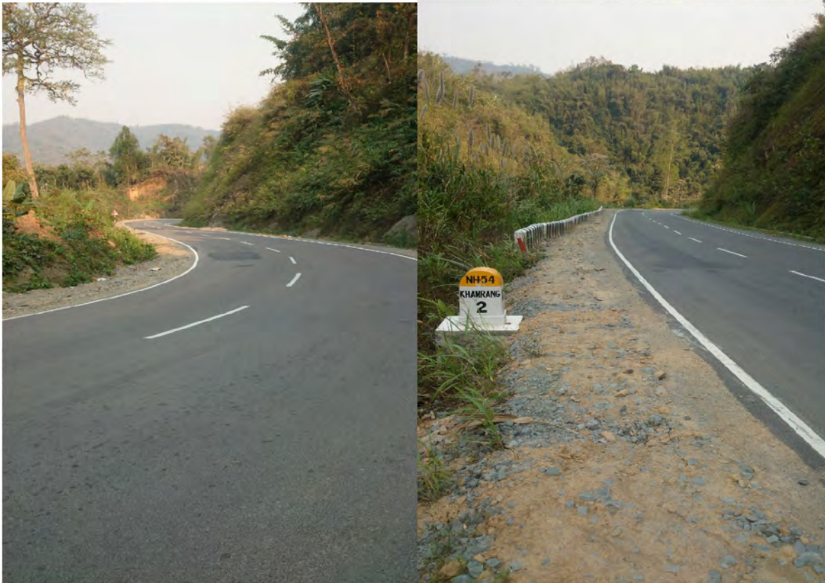
2-laning of NH-54 from km 118/00 to km 133/00 under SARDP-NE : Phase 'A' Package 1/54 (Kawnpui to New Khamrang)
