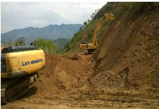
Hill Cutting in progress at @ Ch.18+400
