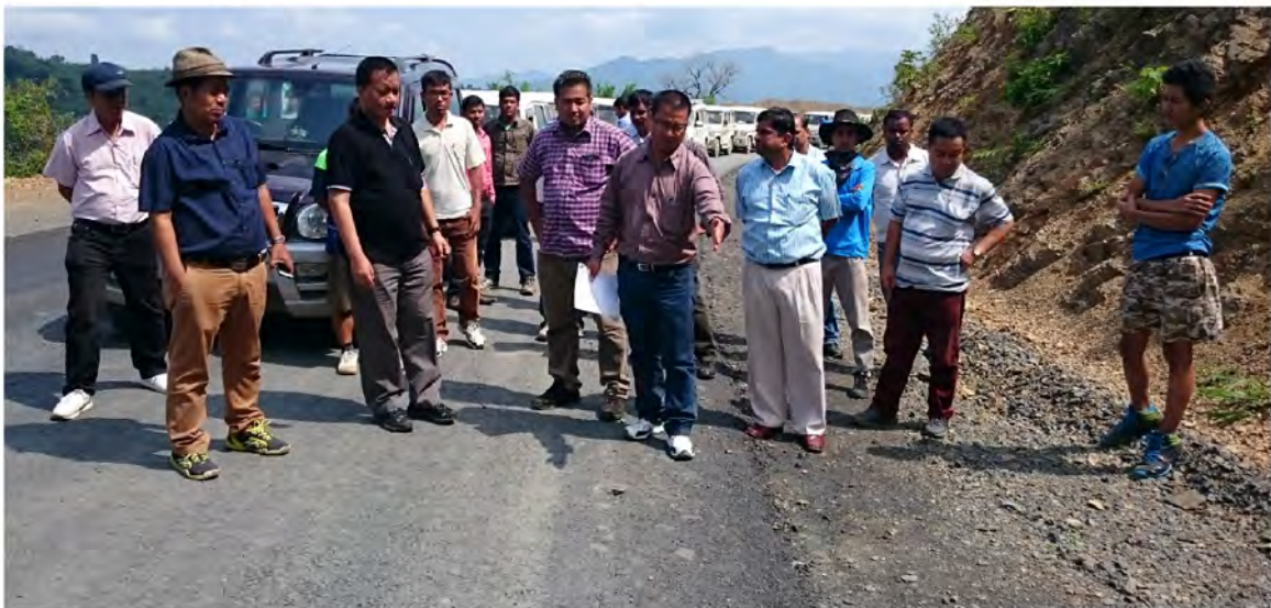
Contractors of Multi Modal Road & Officials having inspection of on-going works
