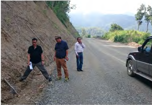
E-in-C assisted by SE, MMPC, having closely Inspection of Road & Side Drain at Multi Modal Road
