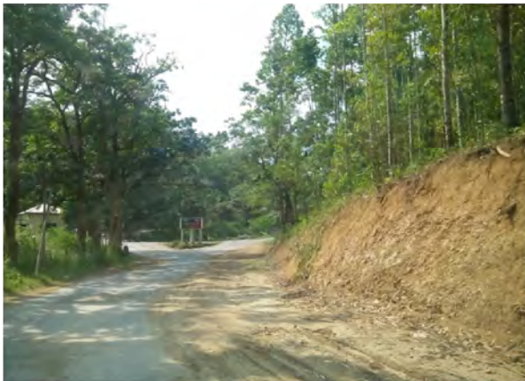
Ch:15+200kmp (Serchhip-WB Road Junction)
