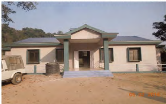
Name of Works : Construction of Police Station at Tlabung
