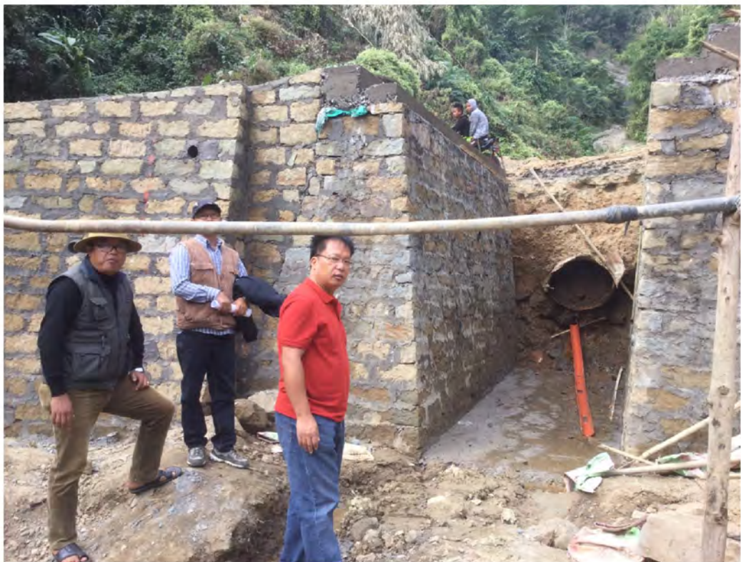
EE, NH Division-III inspecting the Site
