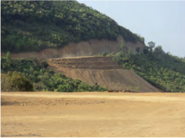
Crib wall construction for minimizing soil erosion
