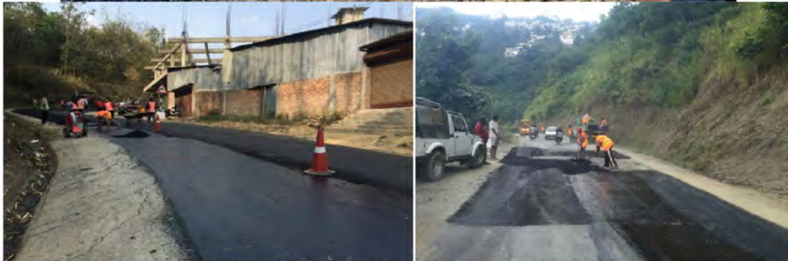
Improvement of Riding Quality on Aizawl Bypass Road 0.0 Kmp to 5.00 Kmp (Resurfacing in patches) & Improvement of Riding Quality on Aizawl Bypass Road 5.00 Kmp to 7.00 Kmp (Resurfacing in patches)
