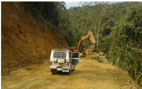
Formation Cutting Ch:18+800kmp of Part-II
