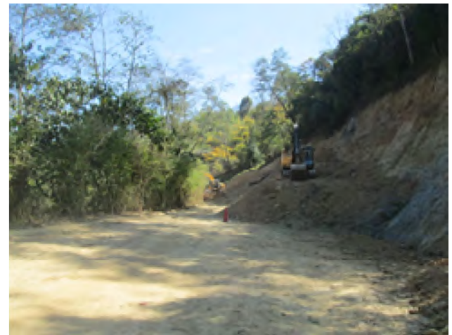
Formation cutting in progress at Km0+200, C – Z Road
