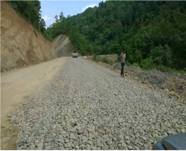
WBM Ist is in progress at Ch 1.610 to 1.700 RHS
