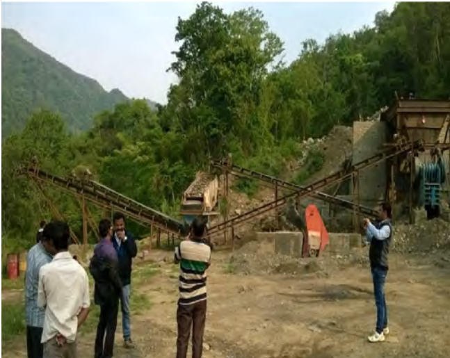
Crusher Plant @Ch 5+600 LHS
