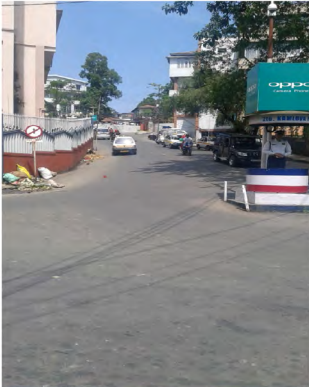
Resurfacing in Patches of Zodin to Sikulpuikawn via Khatlakawn & Resurfacing of Kulikawn - Silaimual Road
