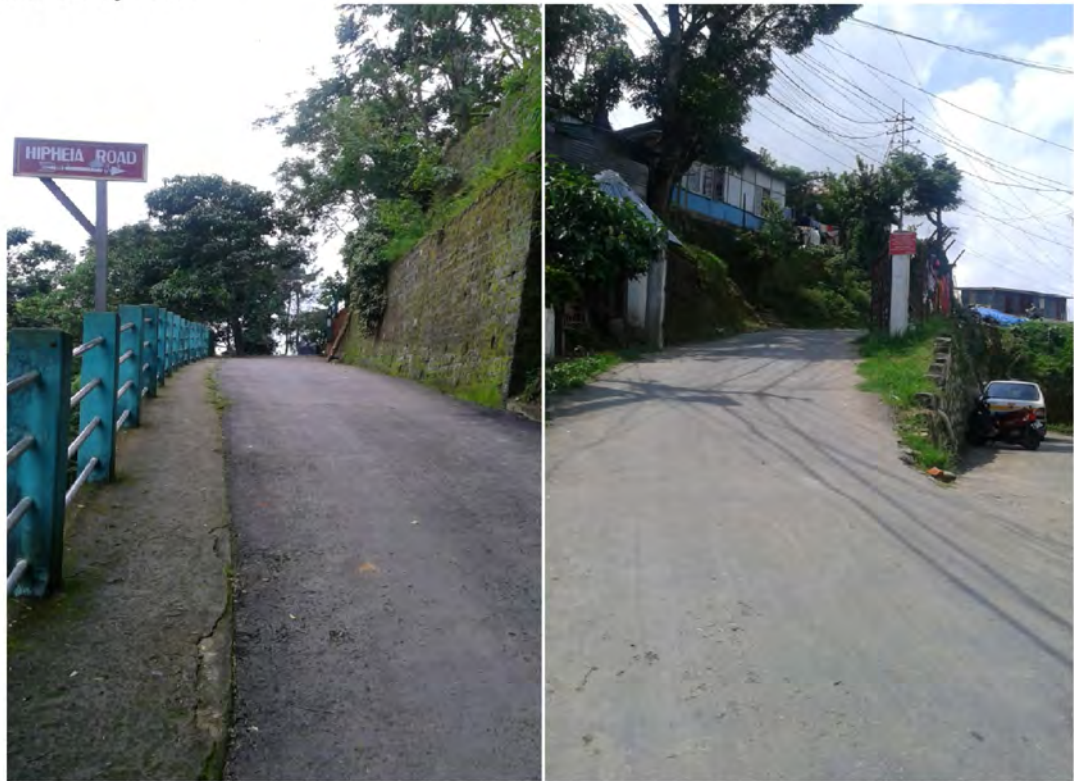
Pavement of Pu Hipheia Road at Dinthar (New Pavement). Patch Repair of Bungkawn to CID Complex Road
