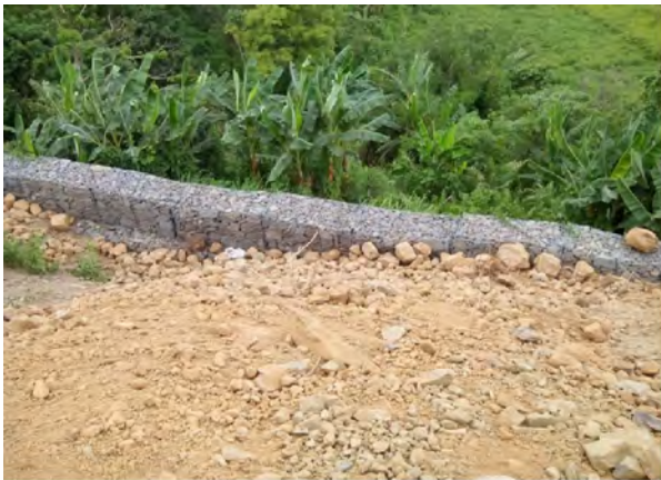
Gabion Wall at Ch: 12+500kmp of Part-I
