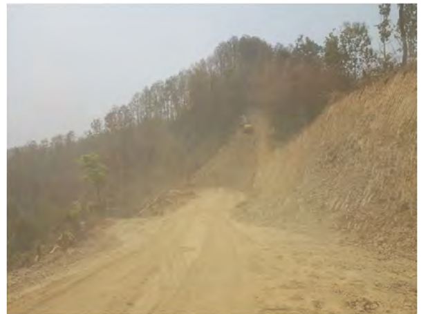
Hill Cutting in progress at @ Ch.12+200
