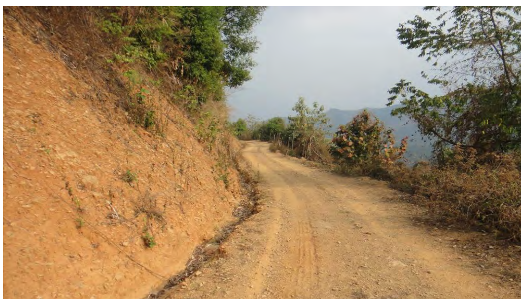
Formation Cutting of Mimbung - R. Tuivai Road NLCPR
