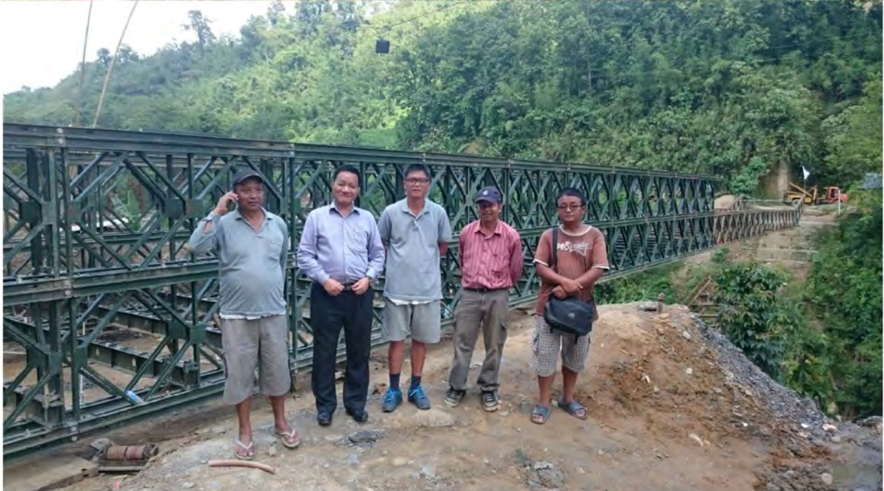
E-in-C is Inspecting Erection of Tlawng Bridge at Sihhmui.
