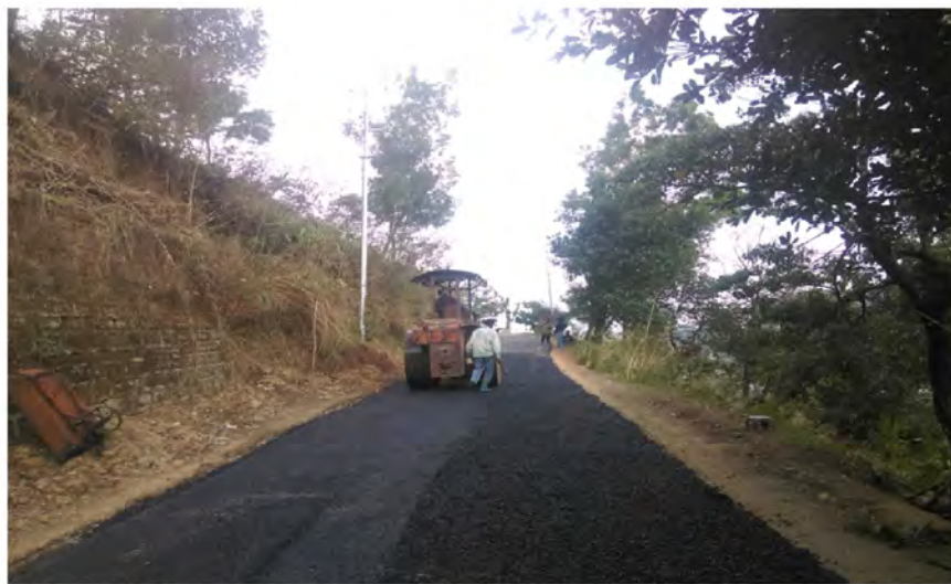
Strengthening and Resurfacing of Amed Veng to Bethlehem Vengthlang
