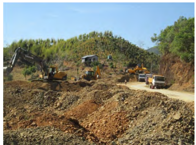
Formation Cutting at Km 7+500, C – Z Road
