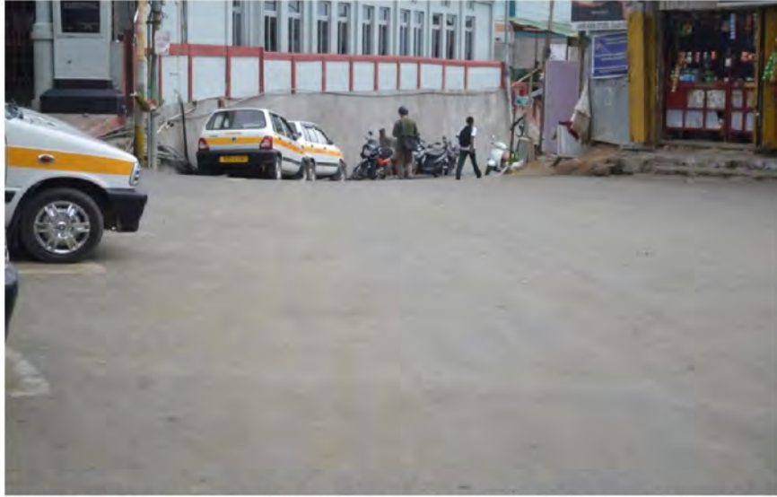
Patch Repair to MHNH road PH-II (from Kanan Biak In to Dawrpui Vengthar) -1
