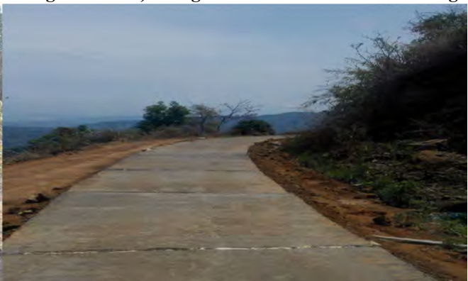
Black Topping at Lungpho-Hmunzawl Road & Cement Concrete Pavement at Chhawrtui-Vanchengpui Road
