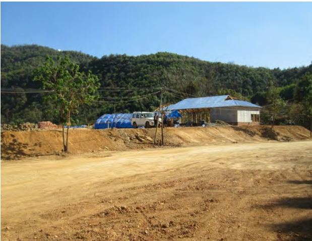
View showing Contractor's Site Lab at Km 14+000, C – Z Road
