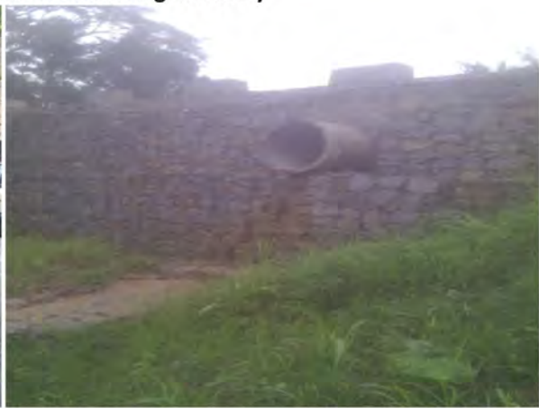
Hume Pipe culvert with Gabion wall on Tuirial Airfield
