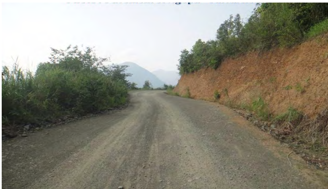
Laying of WBM at Ngopa-Tuivai Road under NEC
