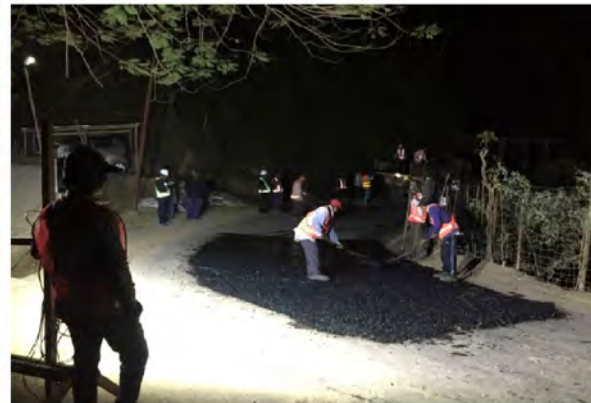
Resurfacing of Sikulpuikawn to Kulikawn & Resurfacing of 3rd MAP internal Road (Bad Patches)
