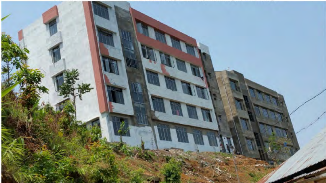
Buildings of MCON Block - I and Block – II at Falkawn
