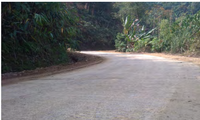
Rigid Pavement (Cement Concrete) Phullen-Phuaibuang – PMGSY
