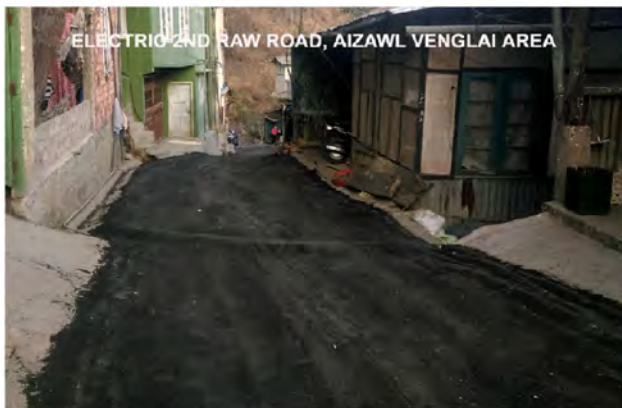
Patch Repair and Seal Coating of Electric Second Raw Road & Patch Repair and Seal Coating of Sihpui to Ramhlun Vengthar
