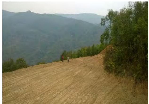
Hill cutting in progress at @ Ch. 18+200 to 18+360
