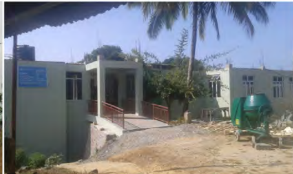
Govt. Kolasib College Main Building
