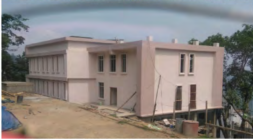
Govt. Zirtiri Residential Science College Library Building at Durtlang
