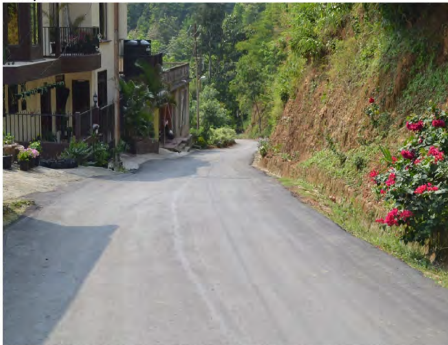
Patch Repair to Building Project to Govt. Complex road-2
