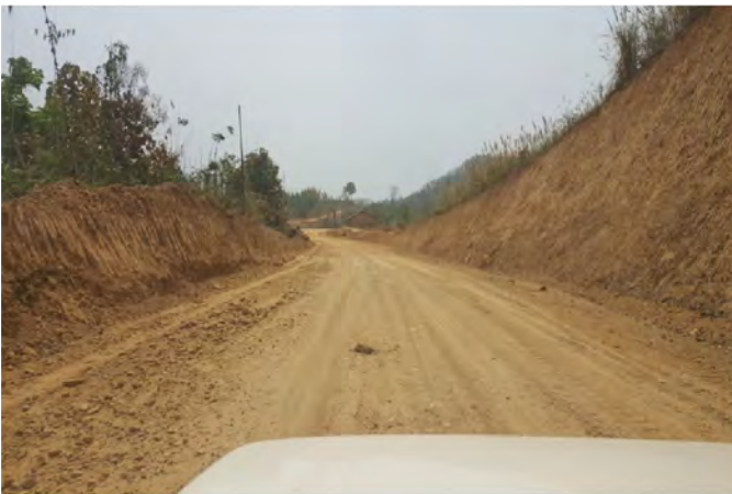
Hill Cutting in progress at @ Ch.11+650
