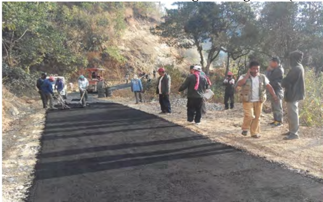
Black Topping at Lungpho-Hmunzawl Road & Cement Concrete Pavement at Chhawrtui-Vanchengpui Road
