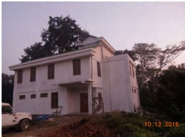
Name of Works : Construction of Police Station at Borapansury
