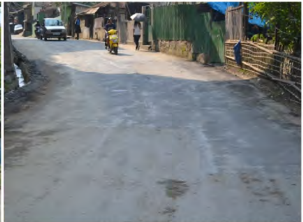
Patch Repair to Vaivakawn to MZU
