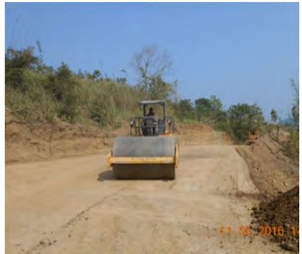
Embankment work in Progress at Km 9+800
