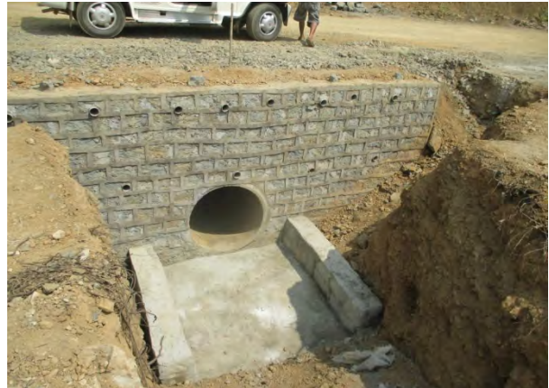
Cross Drainage at Ch:7+102kmp of Part-I
