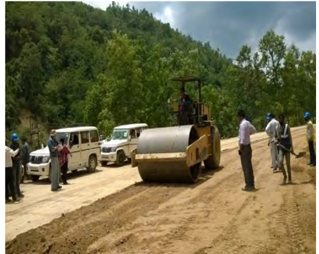
CTS work is in progress @ Ch. 1.990 to 2.040 LHS
