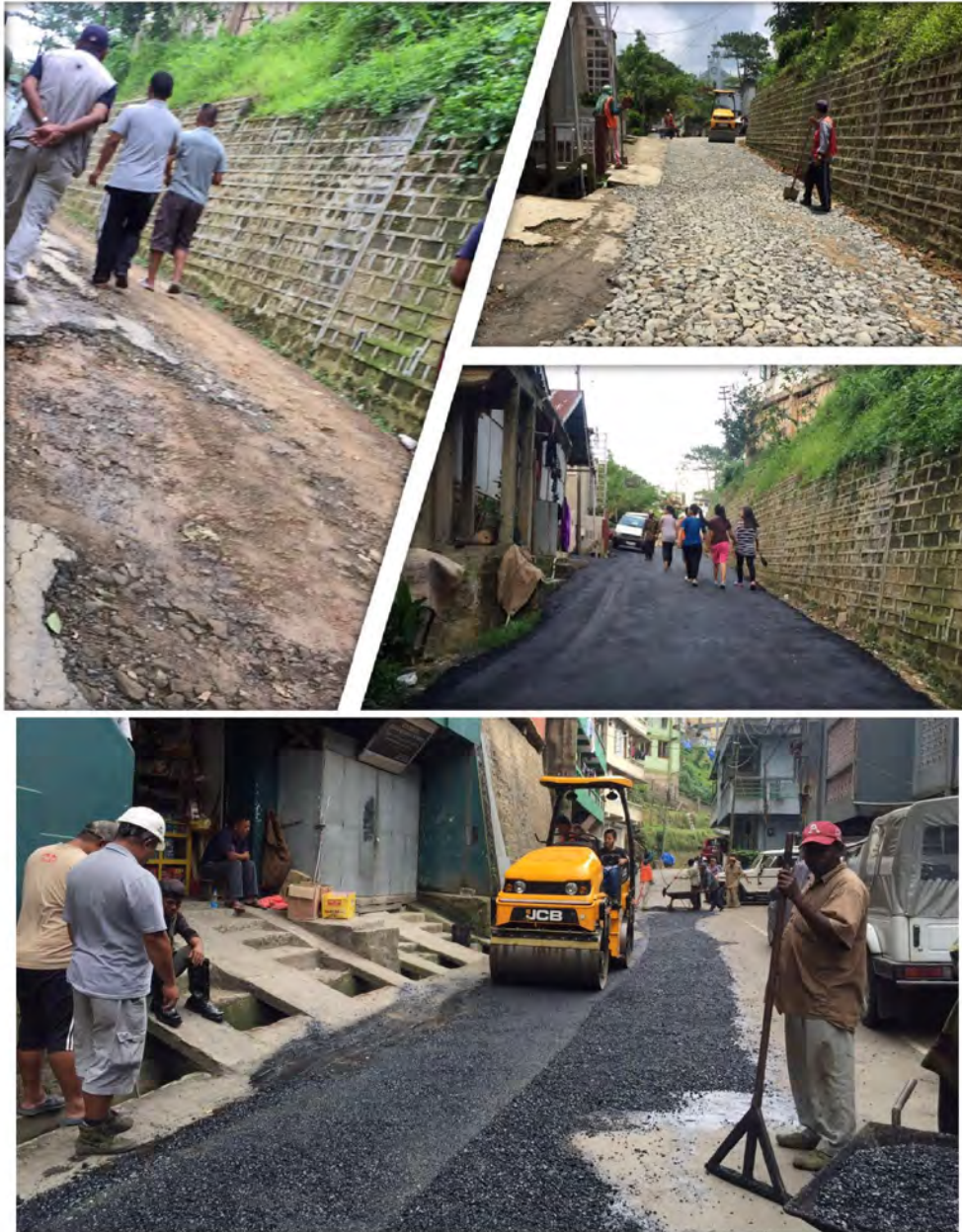
Road repaired works within Aizawl
