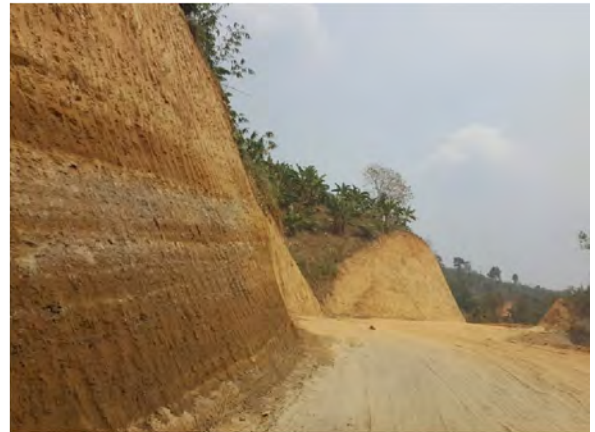
Hill Cutting in progress at @ Ch.22+420
