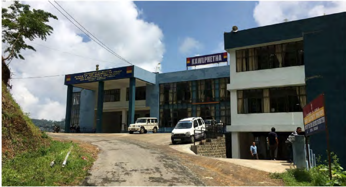
Engineer-in-Chief Office, Power & Electricity Department at New Secretariat Complex
