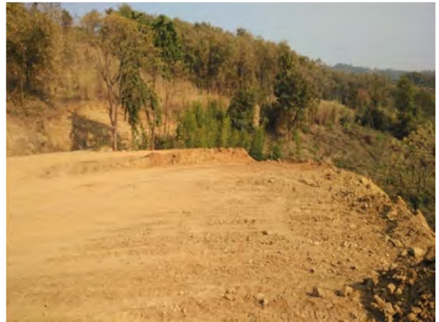
Dumping site @ Ch 17+200
