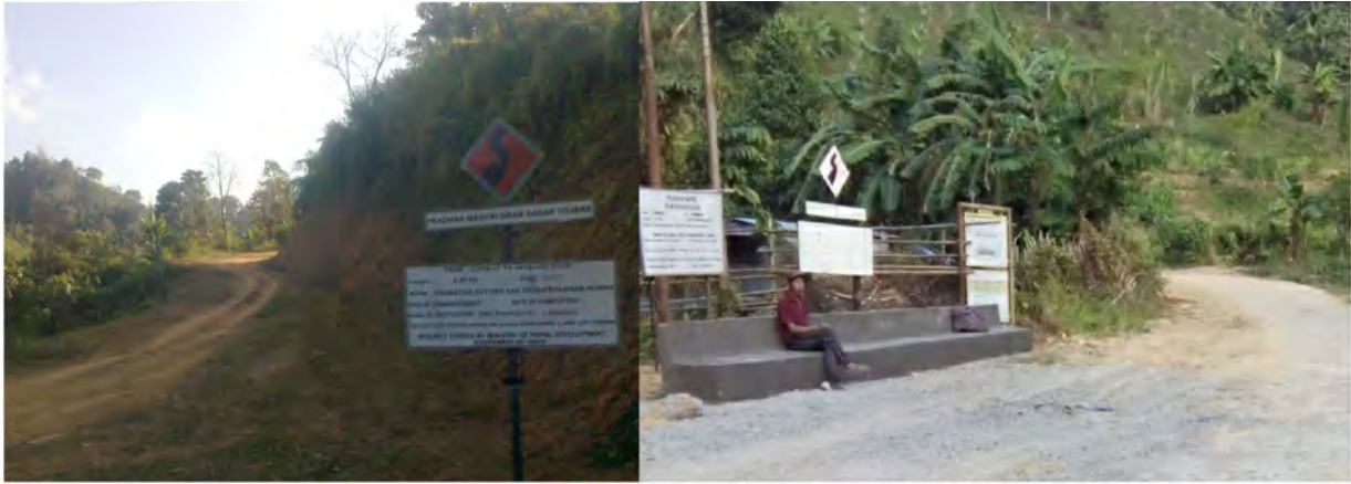
Ch. At 0.000 Kmp Construction of Zohmun to Palsang Road (Sh: Formation Cutting Works & Drainage Works)
