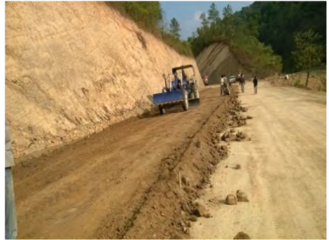
CTS grading in progress @ Km 1+610 to 1+700 LHS
