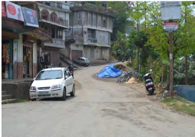
Patch Repair to Ramrikawn to Sakawrtuichhun Road-1 Road-2
