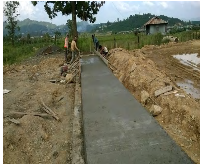
Slab casting is in progress at @ Ch 2.760 for irrigation
