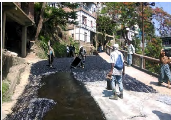
Patch Repair and Seal Coating of Electric Second Raw Road & Patch Repair and Seal Coating of Sihpui to Ramhlun Vengthar
