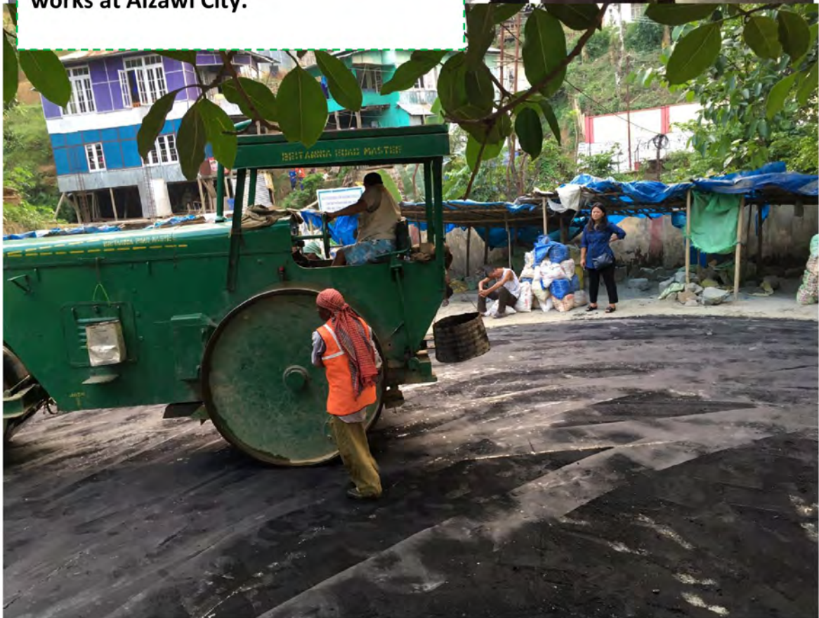
EE & SDO are inspecting pavement works at Aizawl City.
