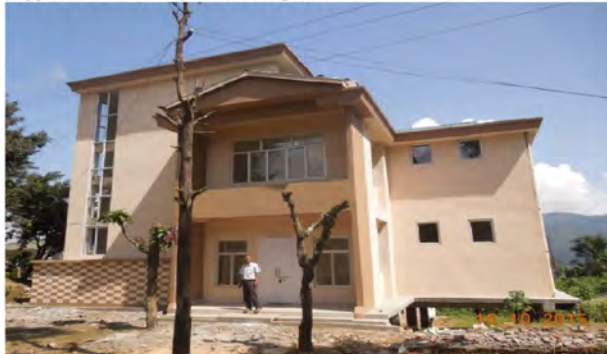
Name of Works : Construction of SDO NH Office at Hnahthial
