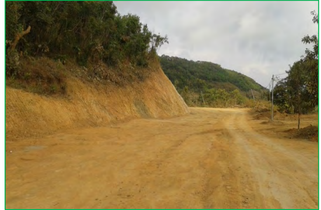
Another Finished View of Formation Cutting @ Km 13+ 200, C – Z Road
