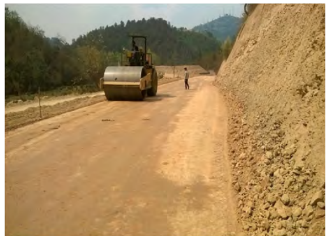
Subgrade preparation @ Ch 1.600 to 1+720 LHS
