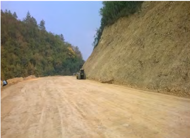
Rolling in progress for embankment @ Ch 0+880 to 1+040
