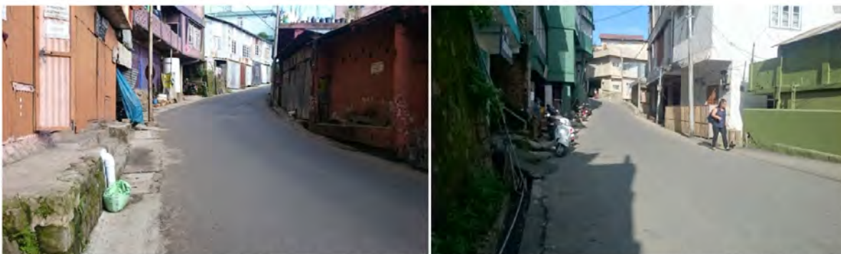
Geometrical Improvement of Mission Veng to Mission Vengthlang road near Pi Rosiami's House & Geometrical Improvement of Mission Veng-Mission Vengthlang Road below Pu J.Lalsangzuala's House
