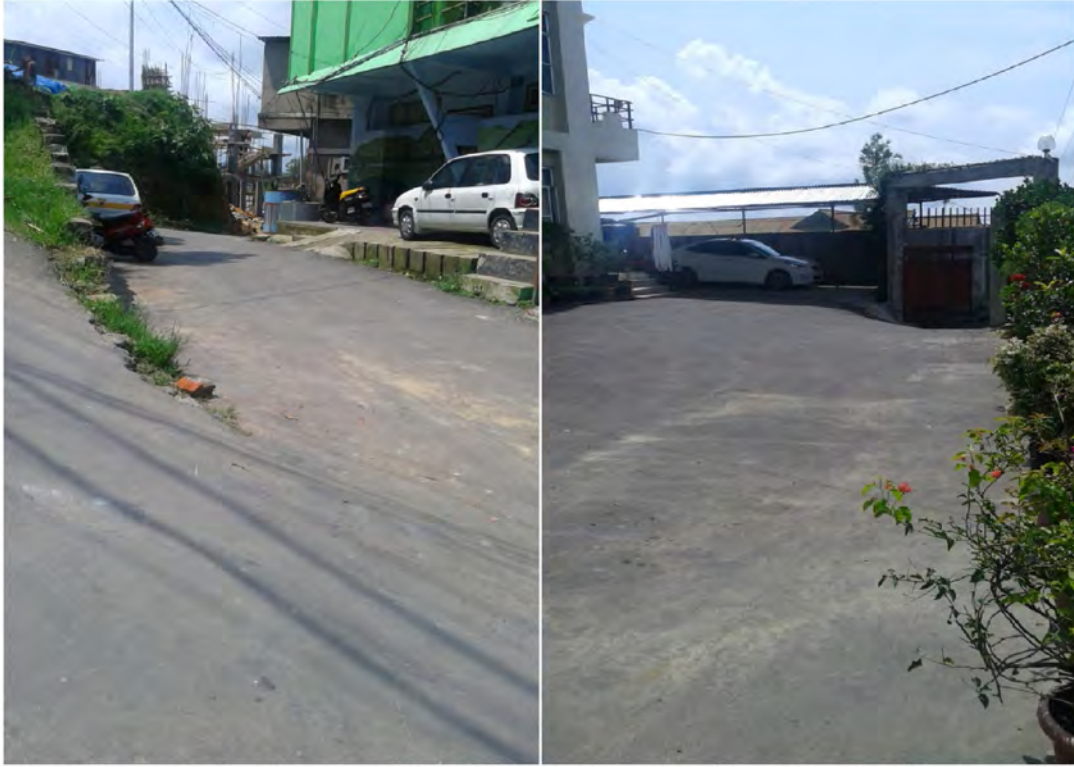
Improvement of Riding Quality of Bungkawn Y.M.A Road. Improvement of Riding Quality of Courtyard 2nos. Of VIP Bungalow at Shivaji Tillah
