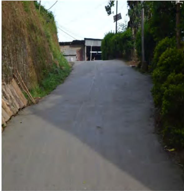
Patch Repair to Chanmari Central Road-2
