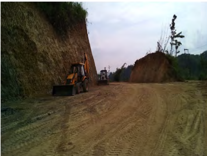
Hill Cutting in progress at @ Ch.15+500
