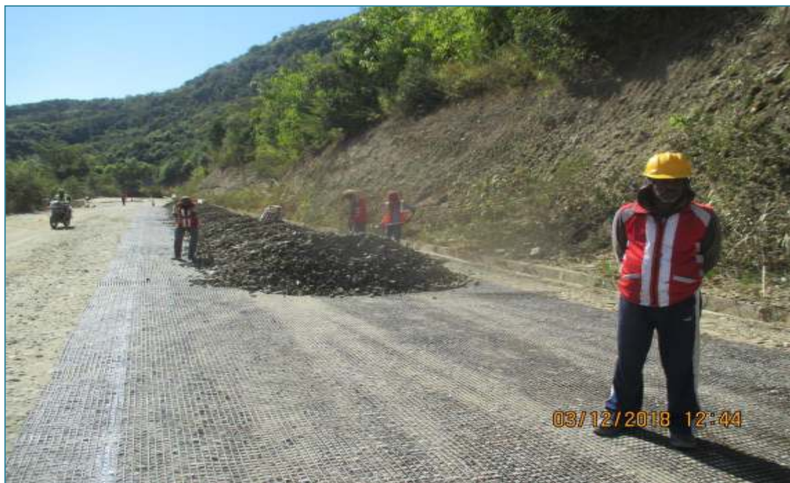
CH. 13+400, LAYING OF GEOGRID AND WBM II
