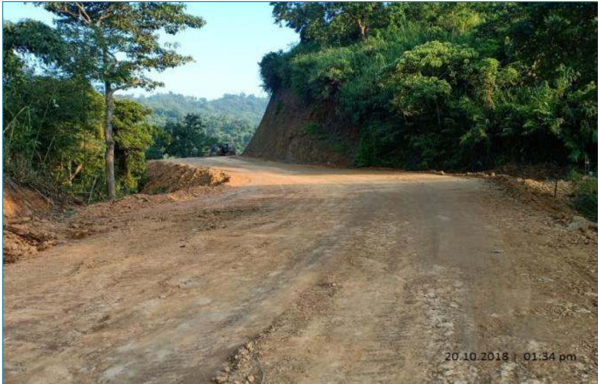
Ch 4+400, Sub Grade Preparation
