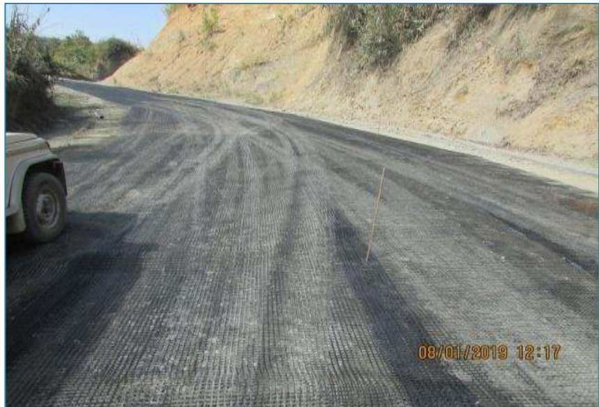
CH. 1+400 B.H.S, GEO-GRID LAYING BEFORE W.B.M 2 ND LAYER SPREADING
