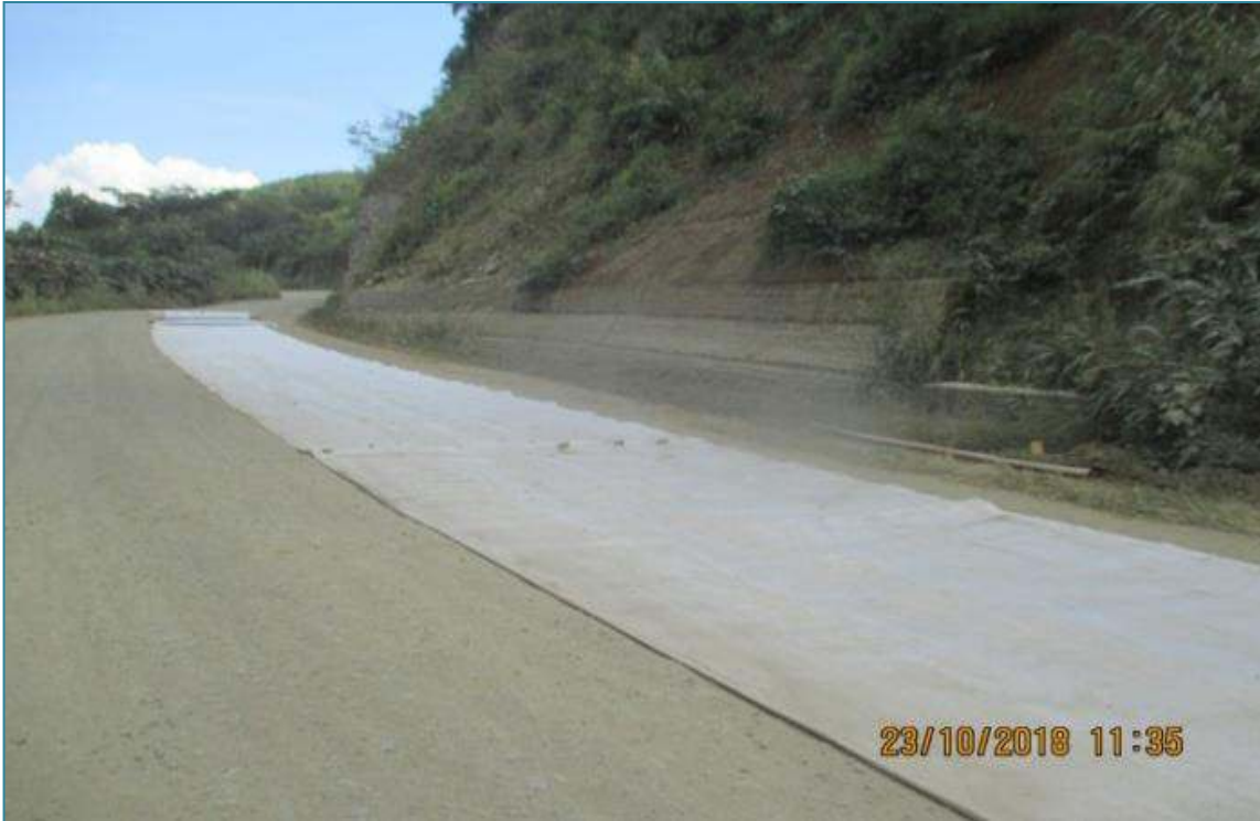
Ch. 10+830, Laying of geotextile
