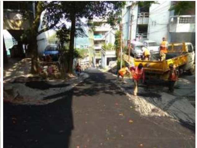
(8) Patch Repair of Zarkawt to Babutlang Approach to Govt.Quater's. Length : 450.00
