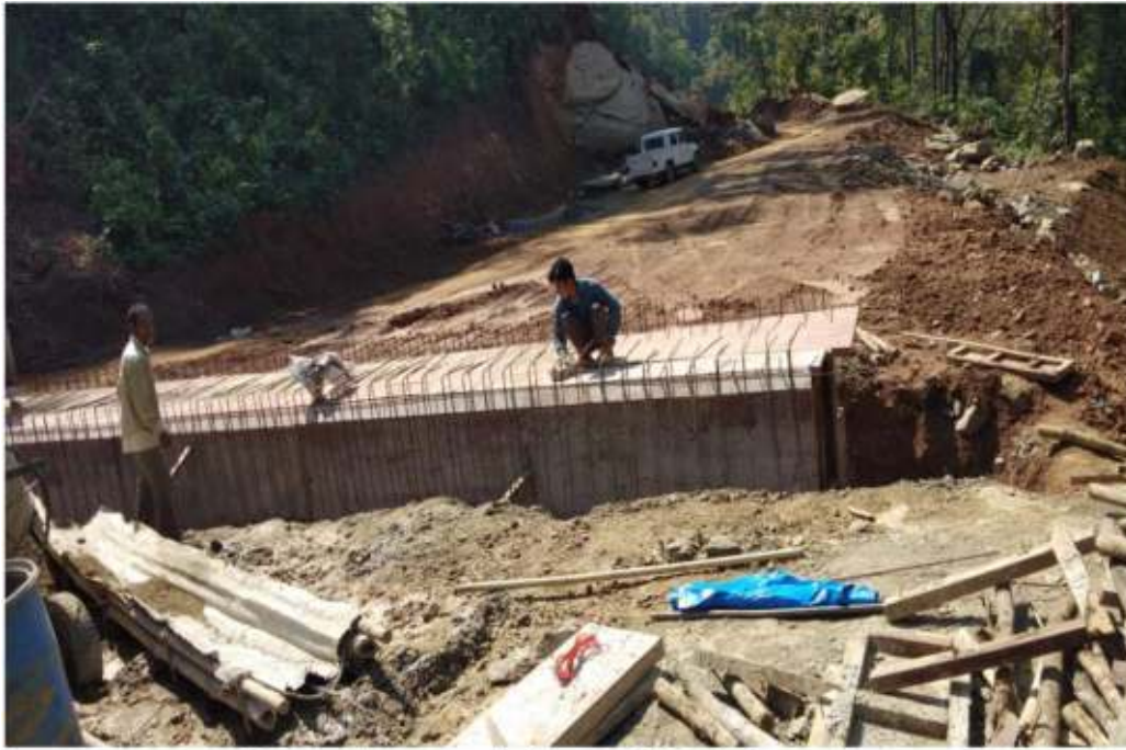
Box culvert at chainage 58.16 Kmp
