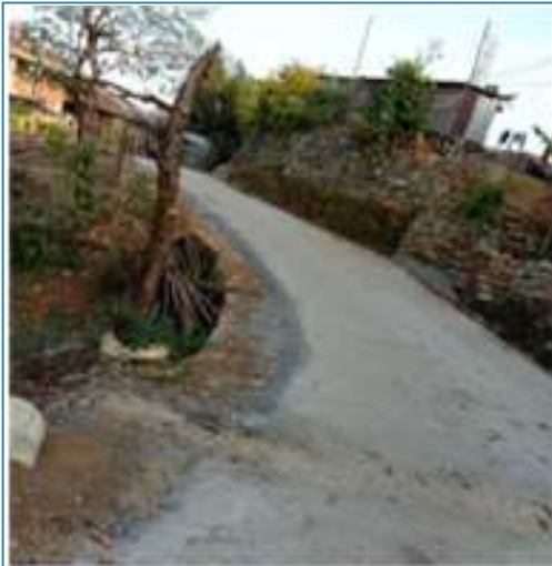
Cell Filled Concrete at Hmuifang Village
