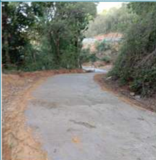
Cell Filled Concrete at Hmuifang - Chawilung Road
