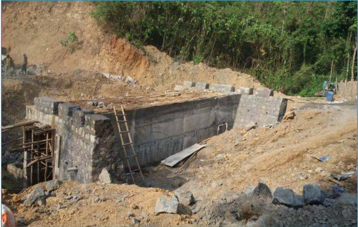
Ch 3+700 Box Culvert Construction
