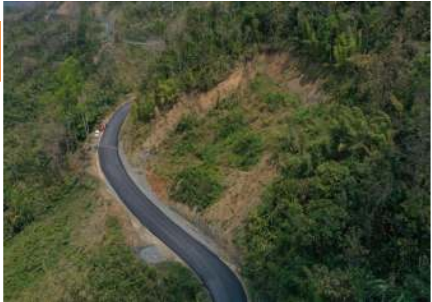
NH44A 44.150 kmp sinking Area
