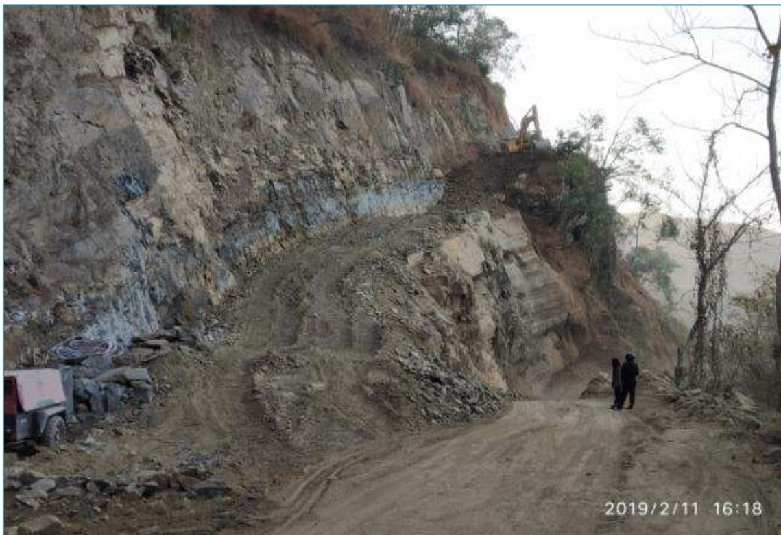
Ch. 14+900 FORMATION CUTTING IN PROGRESS
