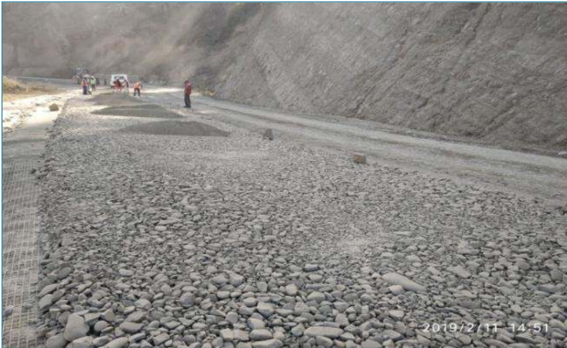
Ch 12+000, LAYING OF WBM II
