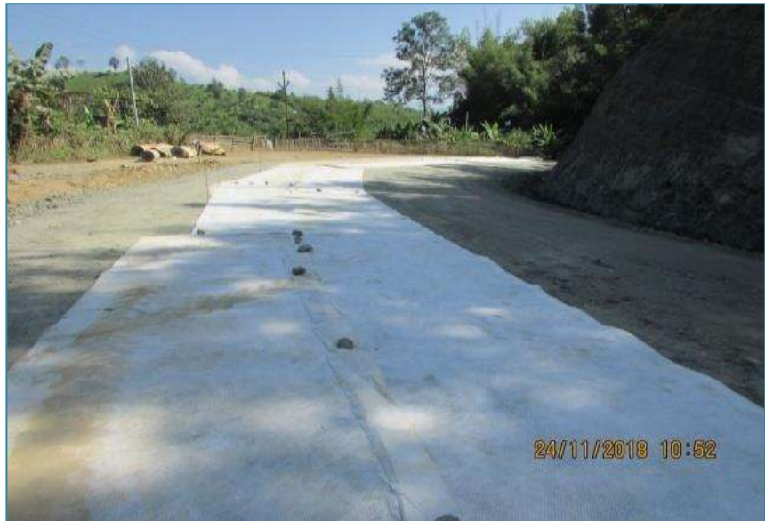
CH 0+100 R.H.S GEO GRID LAYING WORK DONE FOR W.B.M 1ST LAYER SPREADING
