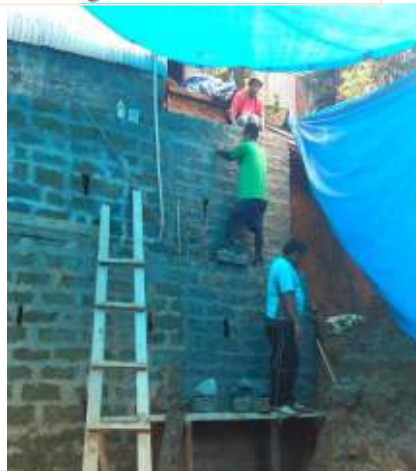
(3) Construction of B/Wall on Elim Road at Chhinga Veng. Length : 13.00
