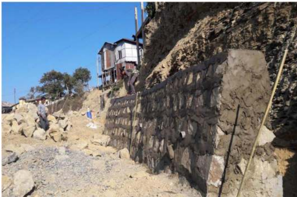
Breast wall at Chainage 59.42 Kmp
