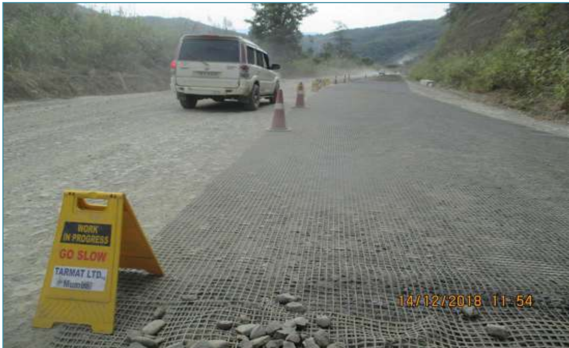
CH. 13+000, LAYING OF GEOGRID
