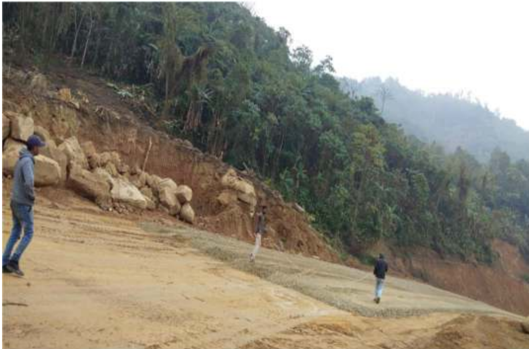
GSB laying at chainage 53.30 Kmp
