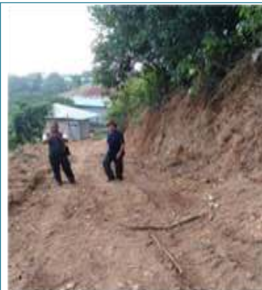
Construction of Internal Roads at Darlung Village (Internal Road between Lallula Hall & Vengchhak Charkawn within Darlung Village)
