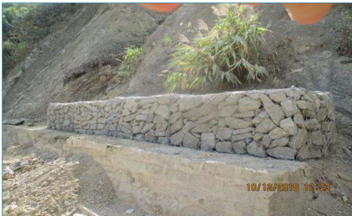
CH 9+530 TO 9+550 RHS, GABION WALL CONSTRUCTION
