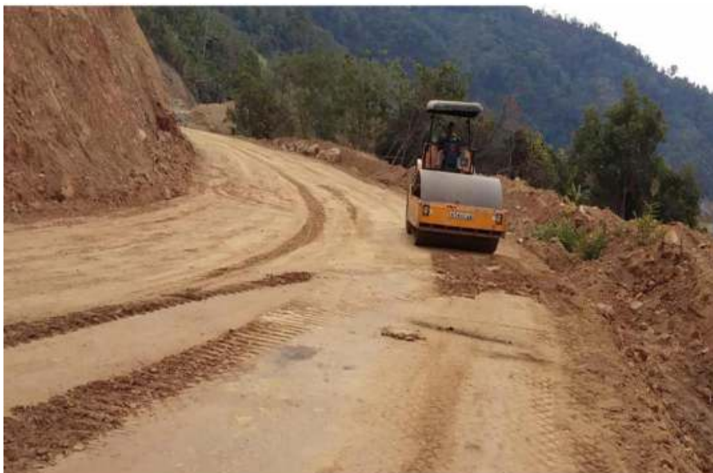
Finished formation cutting at chainage 54.50kmp
