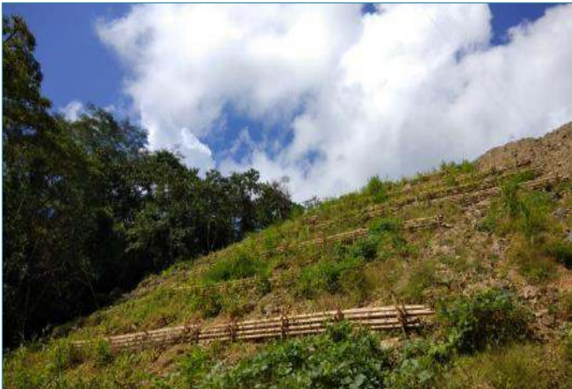
CH. 3+660 RHS BIOENGINEERING WORK DONE FOR PROTECTING THE DISPOSAL SITE
