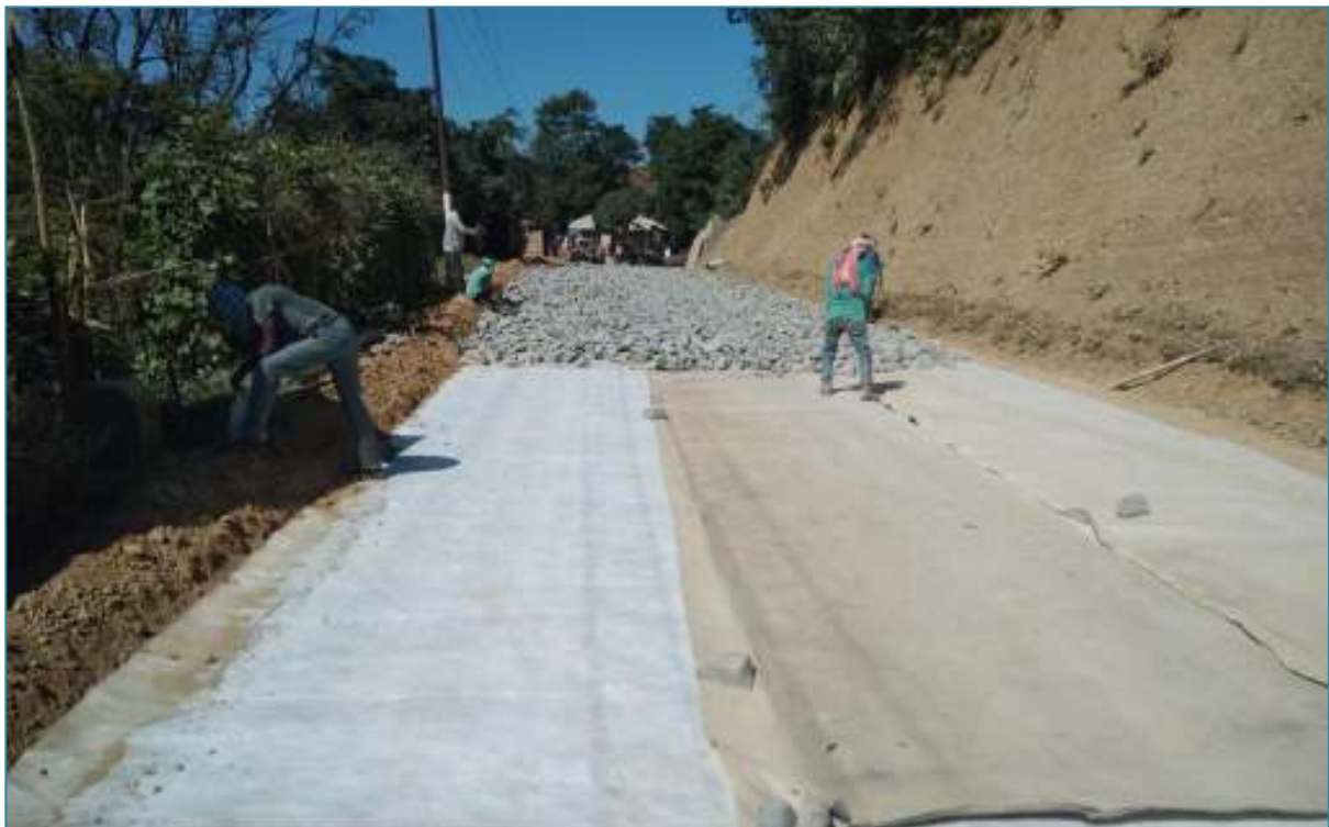
Serchhip – Buarpui Road: Geo-composite layer
