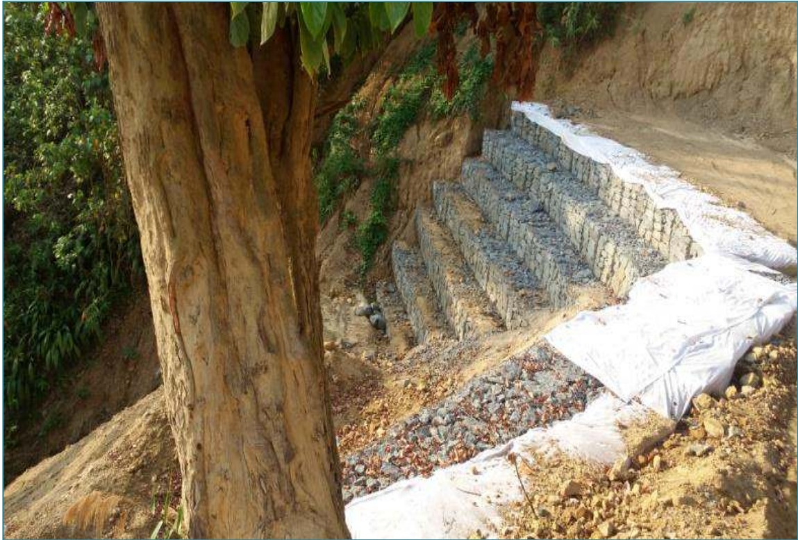
Ch 5+375 GABION SLOPE PROTECTION WORKS
