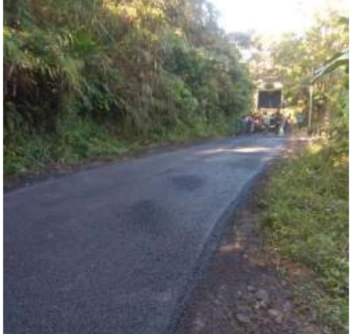
Lawngtlai DC's Office - resurfacing
