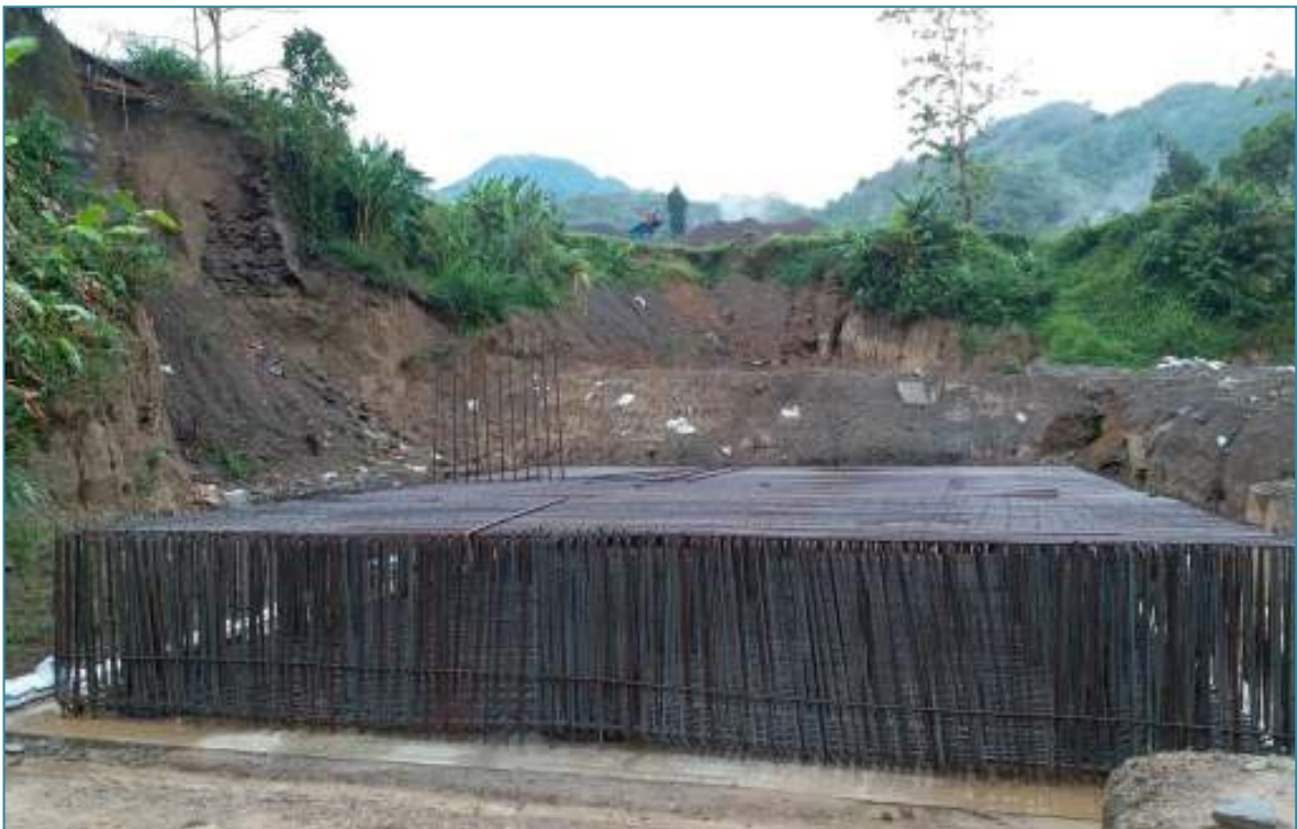
Serchhip – Buarpui Road: Pile cap reinforcement at Tlawng
