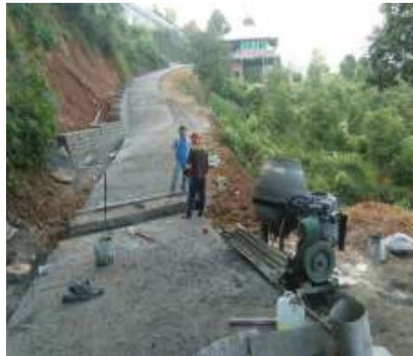
Concrete Pavement for approach road to Bawngkawn 'S' Cemetery at Durtlang Ramthar Total Length = 600.00M.
