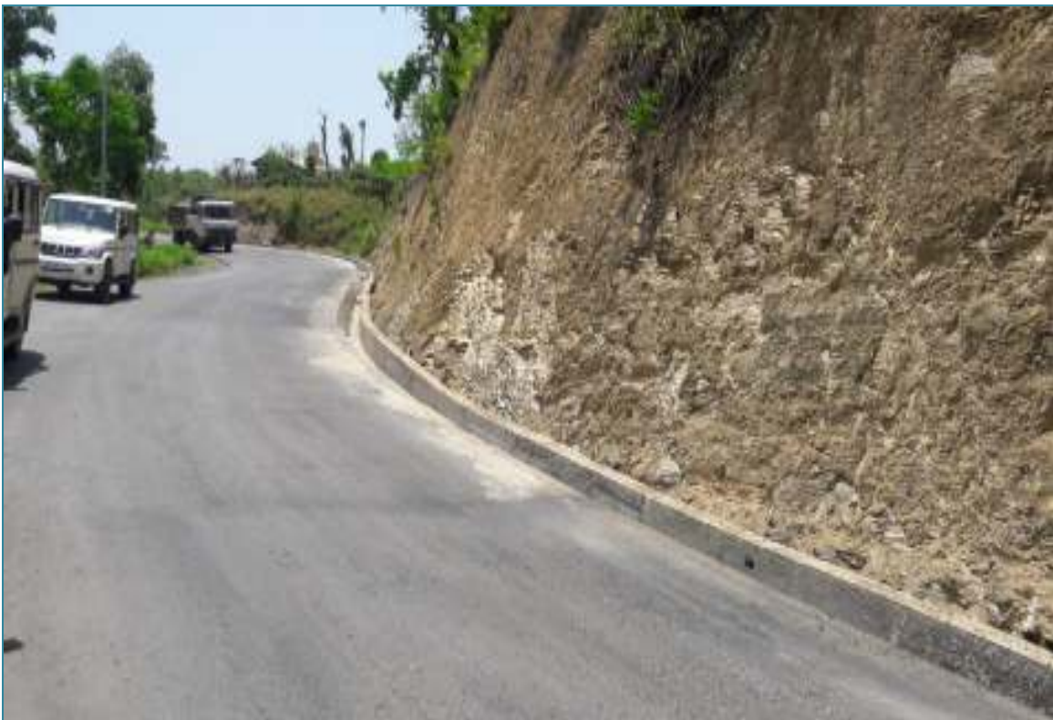
Serchhip – Buarpui Road: Construction of Side Drain
