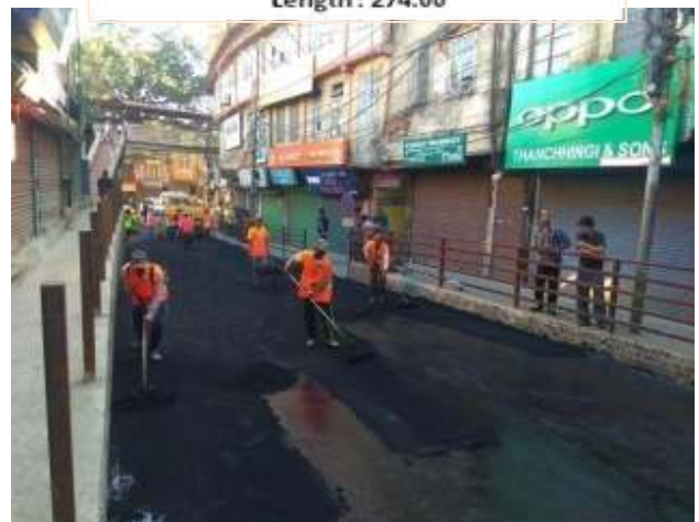
(6) Patch Repair and Sela Coating of Bazar Bungkawm to Millenium Centre Length : 420.00
