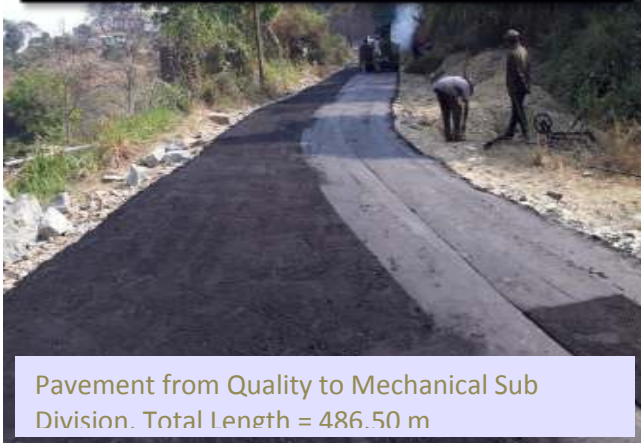
SI No. 25. Patch repair & Seal coating of NH-54 to Sericulture Complex at Zemabawk
