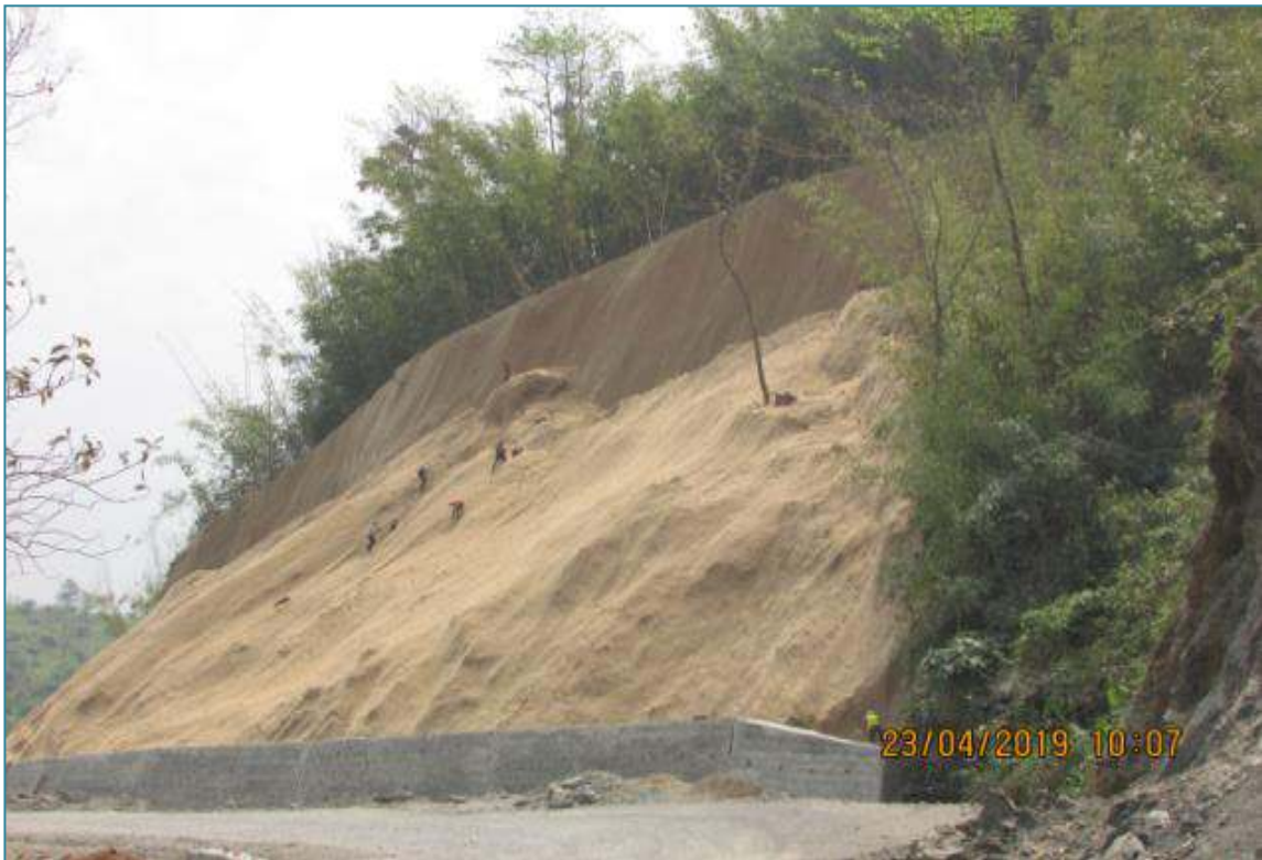
CH 0+110 TO 0+190(RHS), JUTE NETTING COVERING OVER CUT (LAND SLIDE) SURFACE
