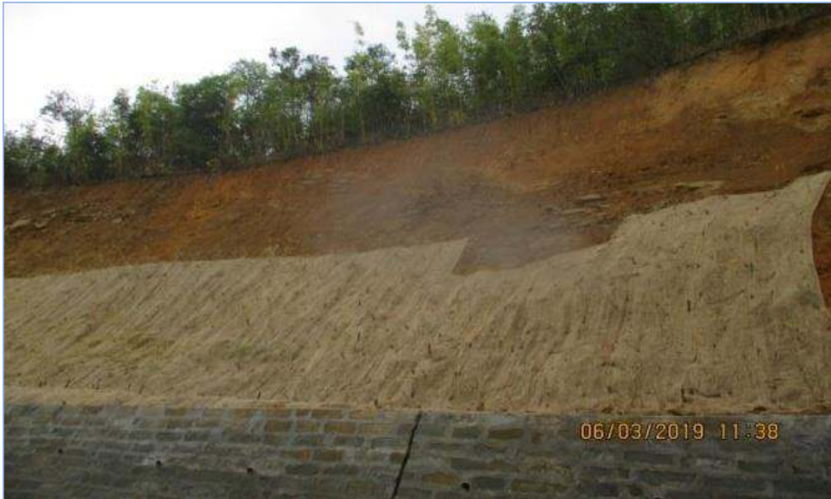
12+550 TO 12+580 RHS, SLOPE STABILISATION BY JUTE NETTING
