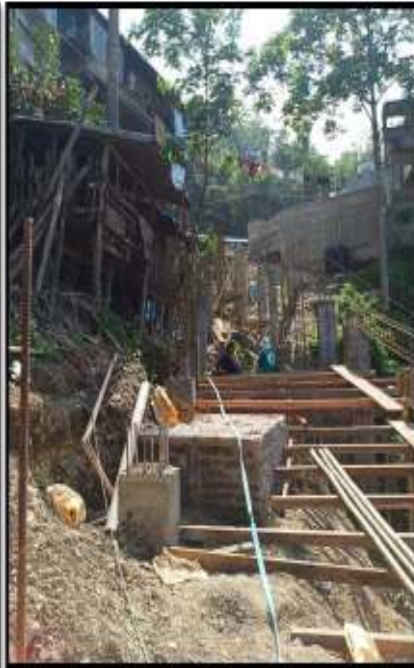
SI No. 12. RCC Balcony on approach road to Old Lunglei Road
