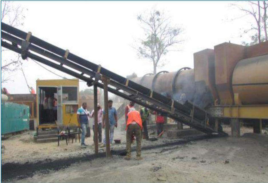
CH 1+800 (CRUSHER & PLANT SITE) HOT MIX PLANT IN FUNCTION
