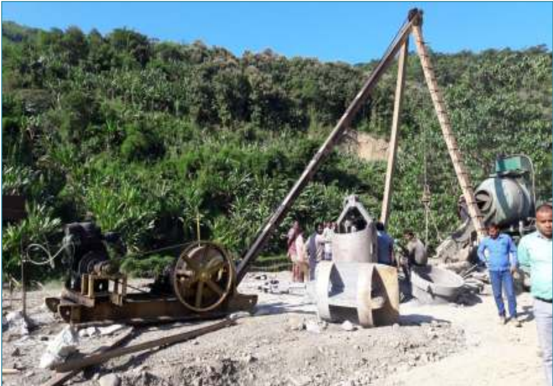
Serchhip – Buarpui Road: Test Pile casting at Mat Bridge site
