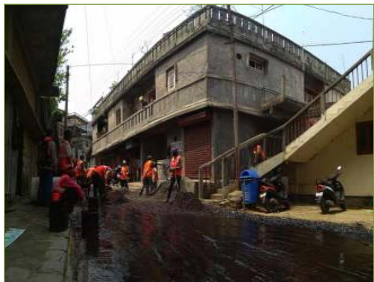
Re-Surfcing of Industry Peng to ramhlun Vengthar Road. Length : 1250.00
