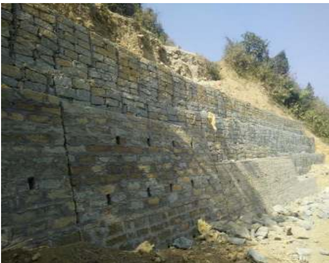
Construction of Masonry Retaining Wall and Gabion structure R/Wall on approach road to Assam Rifles Complex at Zokhawsang at Ch: 0.230kmp. Length 40.00 Rm.
