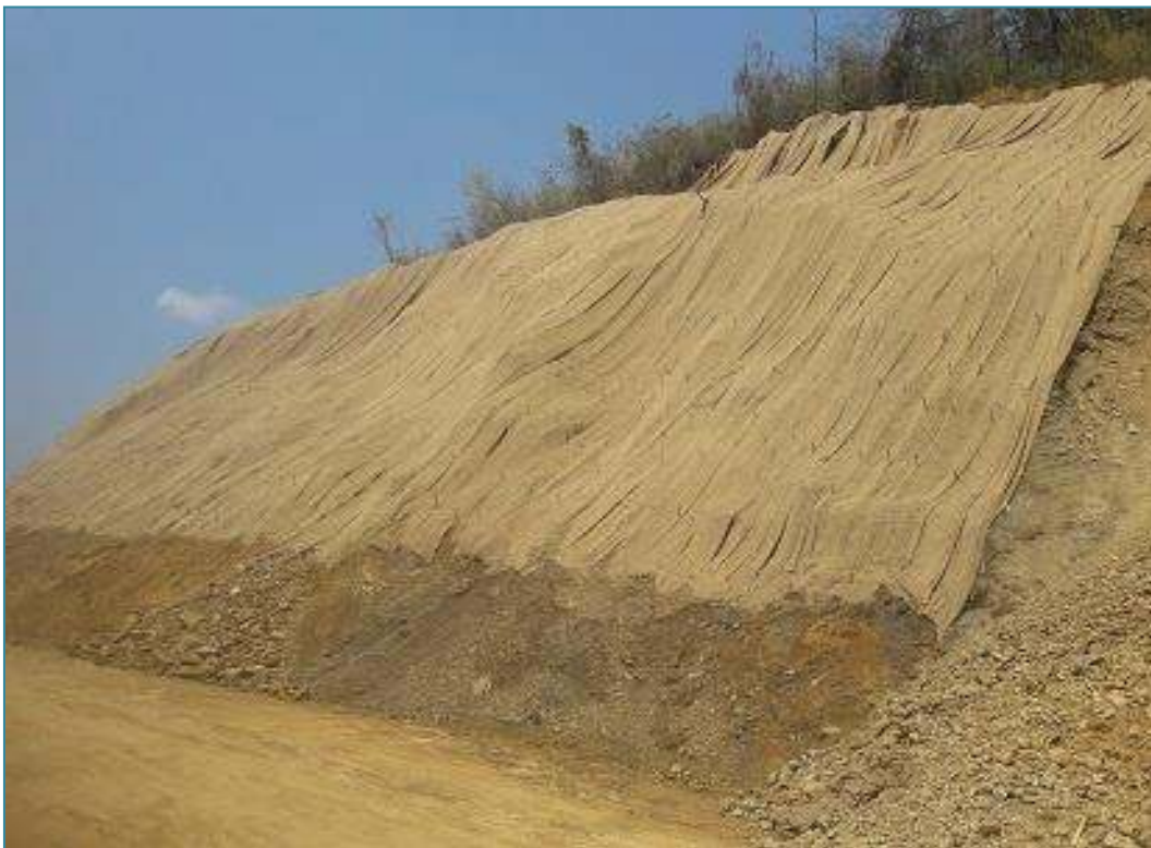
Ch 5+260 to 5+360, JUTE NETTING
