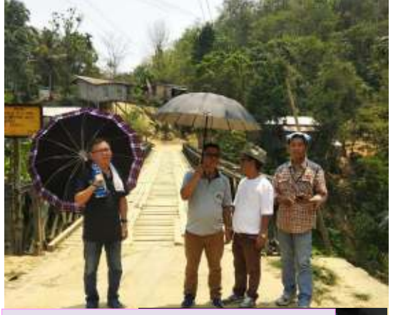
SE inspected Bailey Bridge R. Sazek
