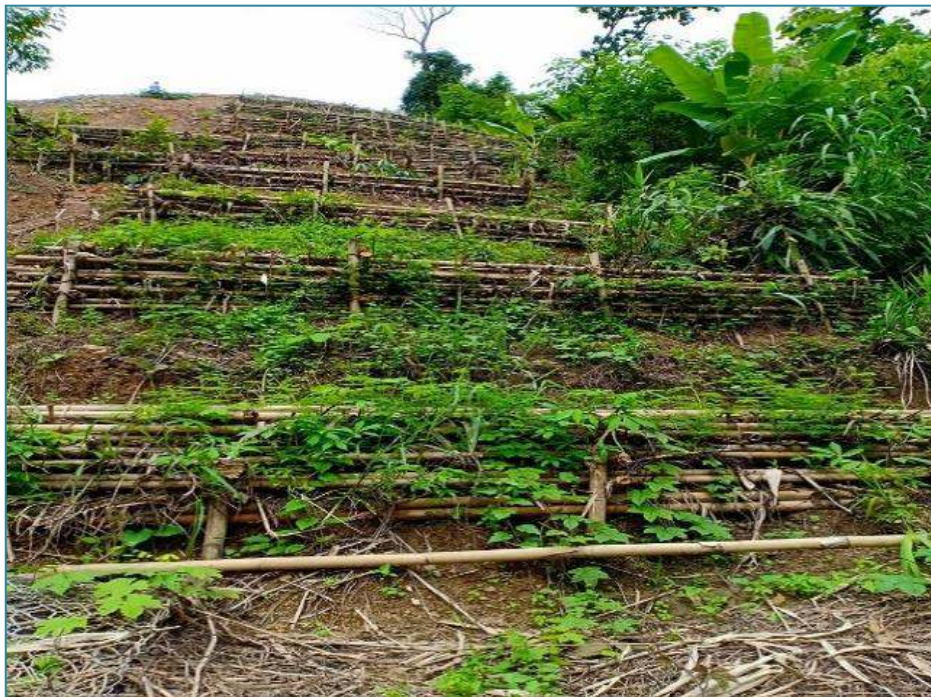
Ch 1+910 to 1+970, BIO ENGINEERING PRACTICE
