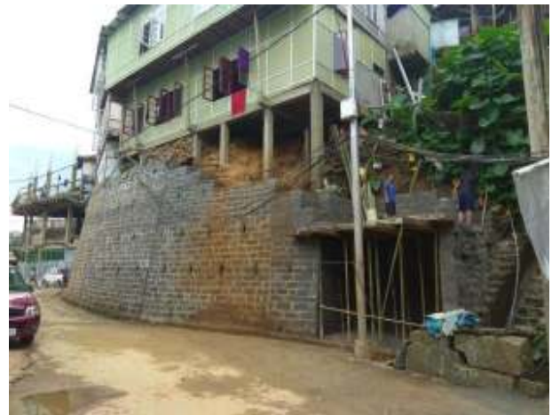
(2) Construction of B/Wall Below Pu Lalthantluanga's House on Armed Veng to Electric Veng Cemetery at Chhinga Veng Length : 18.00
