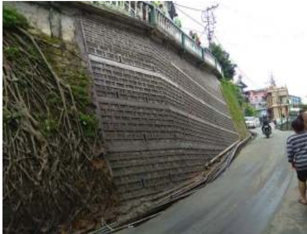
(1) Re Construction of R/Wall on Approach Road to Chief Minister Bungalow from Zarkawt. Length : 14.50
