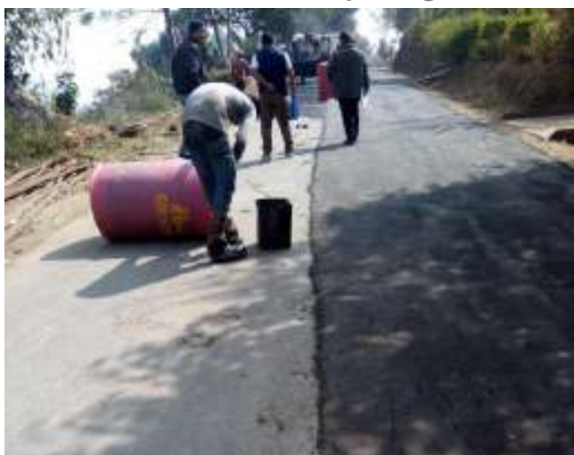
CEO and his team inspecting Mamit Town on 30.1.2019.
