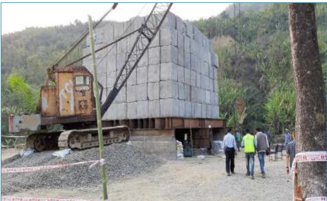
Serchhip – Buarpui Road: Initial Pile Load Test at R. Mat
