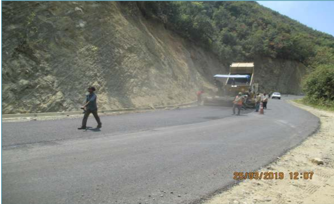
CH. 9+900, LAYING OF DBM
