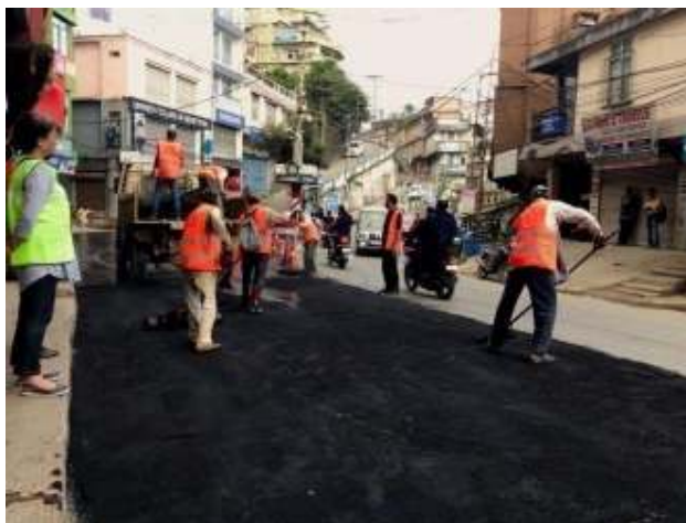
(5) Patch Repair and Seal Coating of Chanmari to Bazar Bungkawm via Zarkawt. Length : 1500.00
