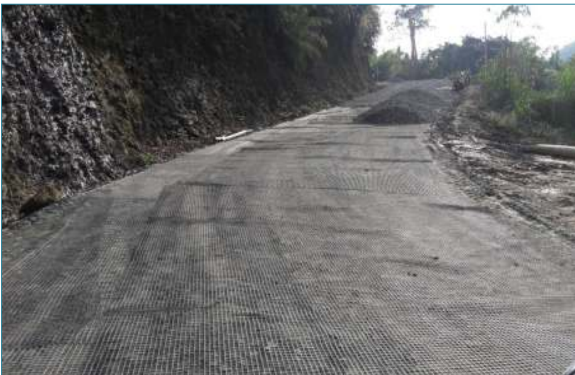
Serchhip – Buarpui Road: Geo-grid layer Pictures of Serchhip – Buarpui Road, contd.2
