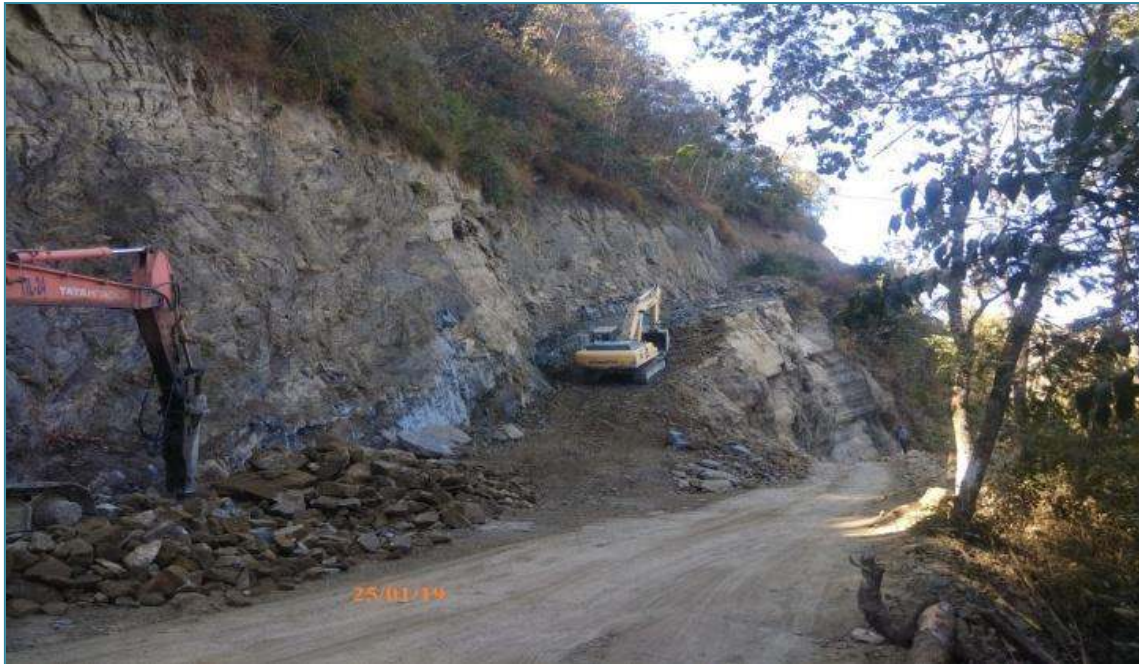
Ch. 15+000 RHS Excavation in Progress
