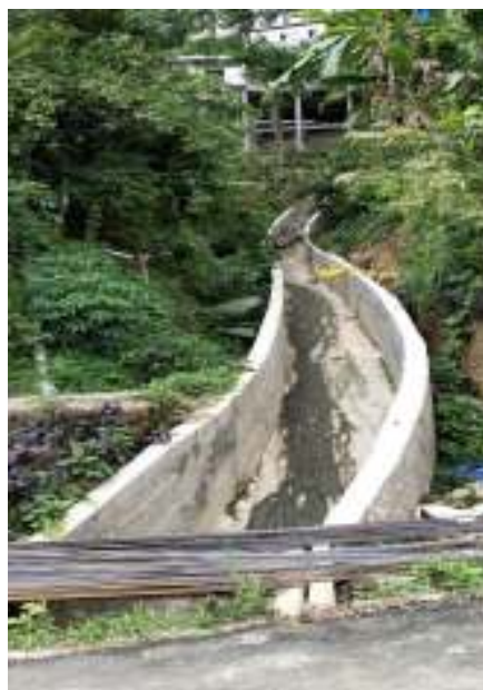
14.Construction of Drain to Potect Dawrpui Cemetry at Chhinga Veng, Length= 214Rm
