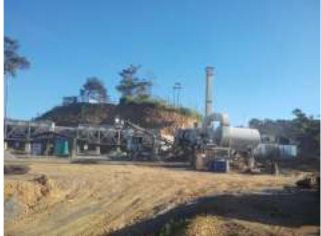
12. 65.100 - 44A13. 66.400 - 44A Mamit Plant
