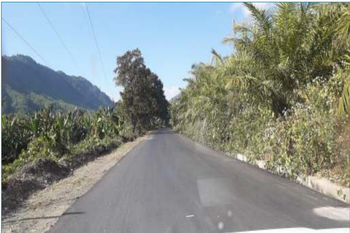
Serchhip – Buarpui Road: Completed BC layer
