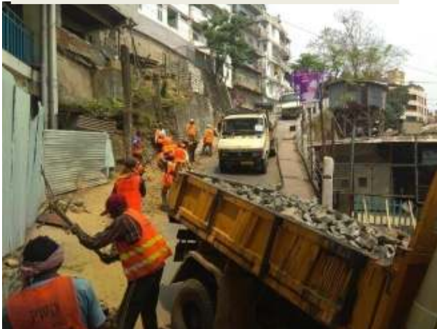
26. Resurfacing of Bazar Bungkawn to saron Veng road , Length = 650Rm
