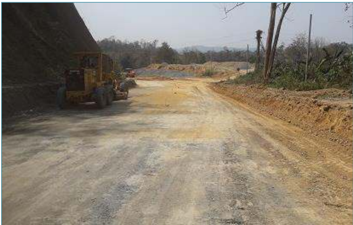
Ch 5+400 to 5+600, Sub Grade Preparation
