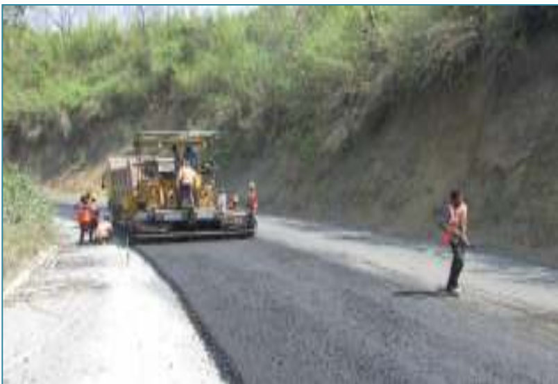
CH 1+500 TO 1+700(RHS) LAYING OF D B M
