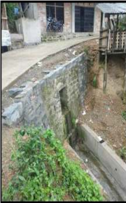
SI No. 11. Rigid Pavement Kailiana Road
