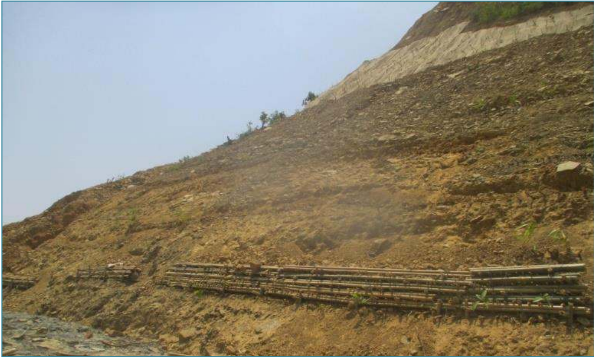
CH. 1+100 RHS, BAMBOO CRIB WALL
