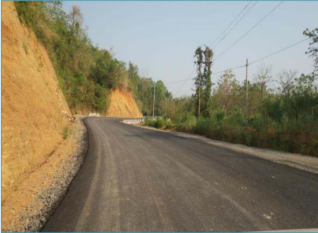
Ch 4+500, LAYING OF DBM
