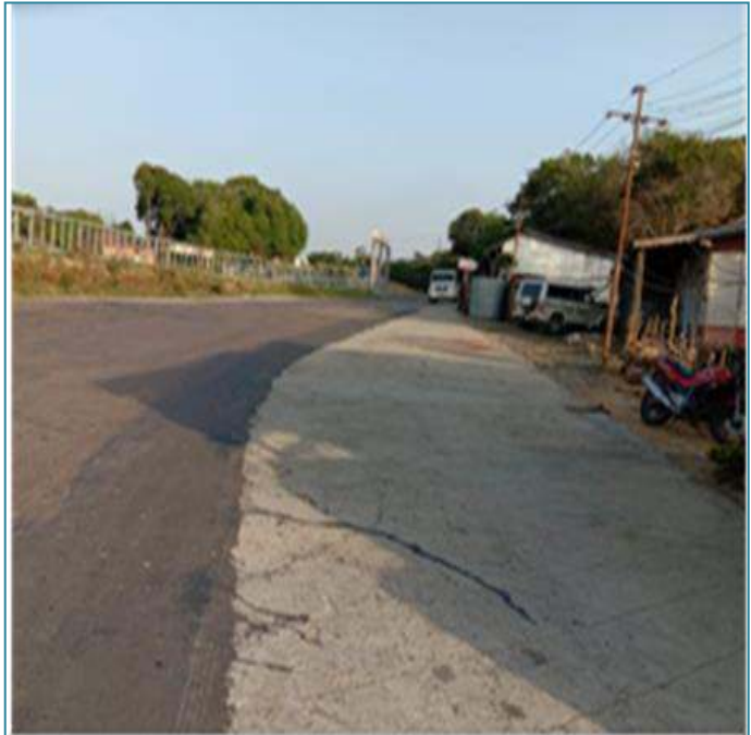
Cell Filled Concrete at Hmuifang Village
