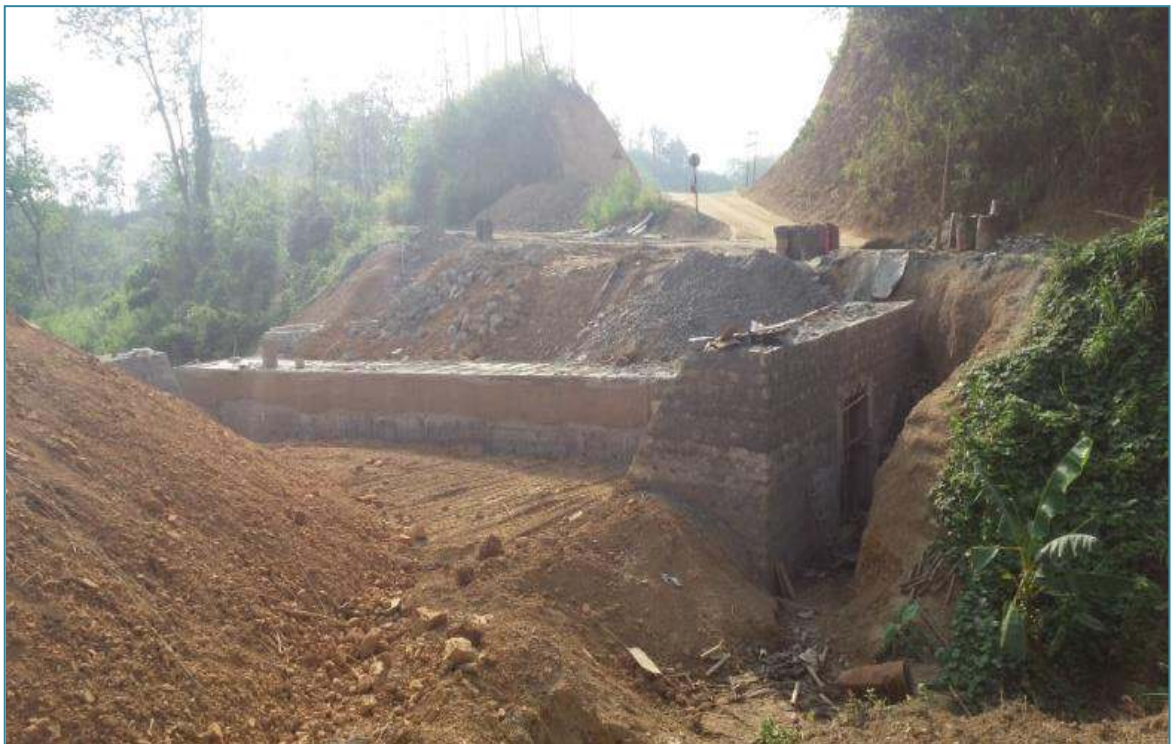
Ch 3+370 Box Culvert Construction
