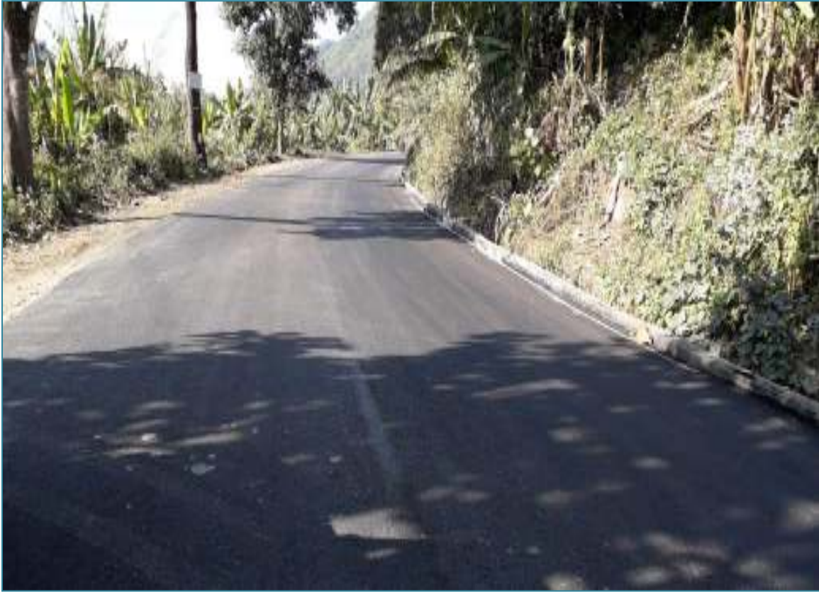
Serchhip – Buarpui Road: Completed DBM layer
