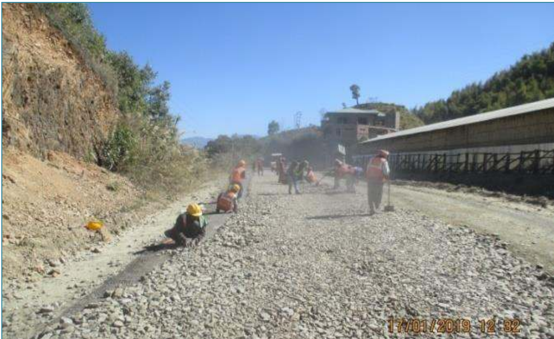
Ch. 10+550, laying of WBM II
