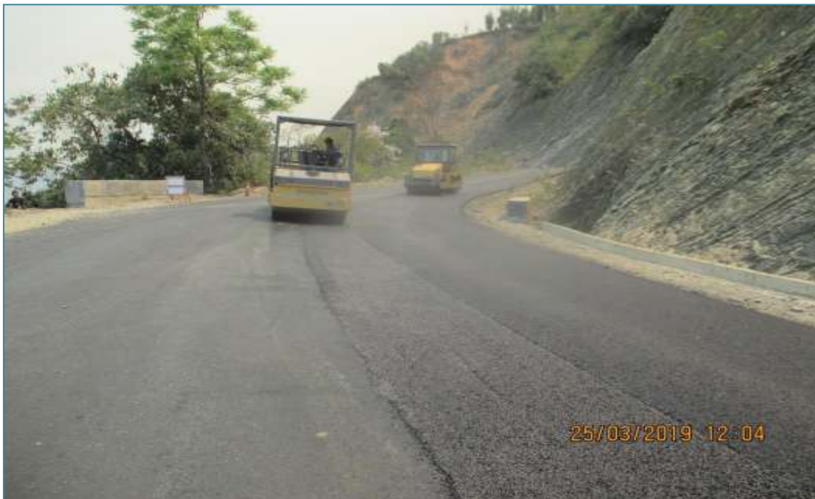
CH. 9+920, LAYING OF DBM
