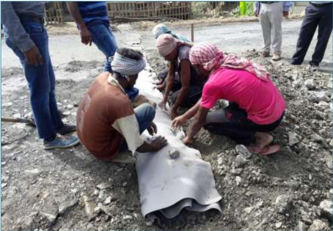
Serchhip – Buarpui Road: Non-Woven Geo-textile sub-surface drainage
