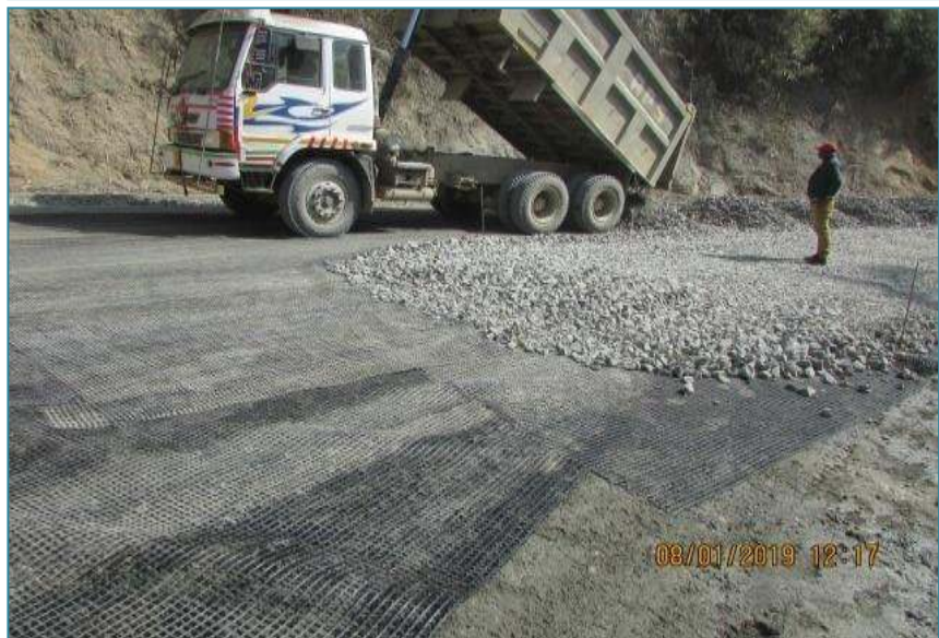
CH 1+500 TO 1+590 BHS, W.B.M 2 ND LAYER SPREADING WORK IN PROGRESS.
