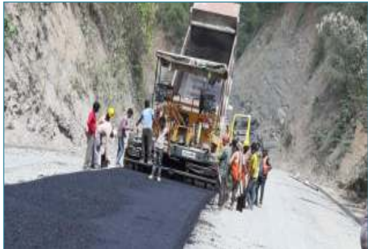
CH 1+300, (LHS) DBM LAYING IN PROGRESS
