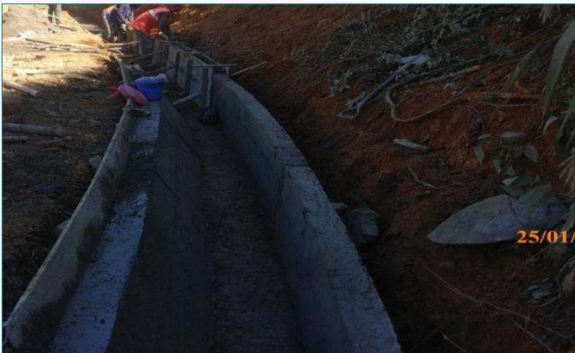
CH. 11+910 TO 11+940 RHS, CONSTRUCTION OF SIDE DRAINS
