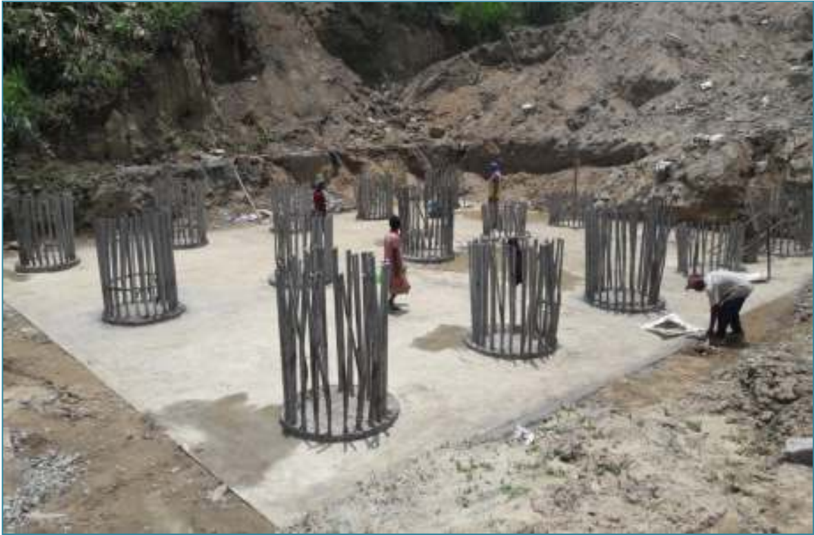
Serchhip – Buarpui Road: Pile Foundation for Major Bridge over R. Tlawng
