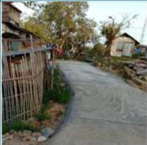
Cell Filled Concrete at Hmuifang Village
