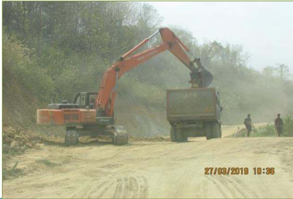
CH 30+700 TO 30+760 BHS EXCAVATION IN PROGRESS
