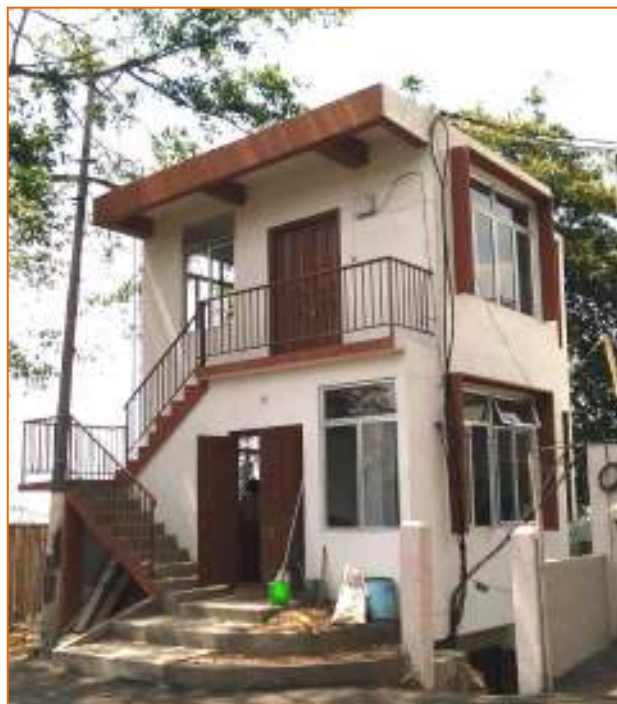
NAME OF WORK : CONSTRUCTION OF OPERATOR DUTY ROOM AT CHIEF SECRETARY COMPLEX. A/A AMOUNT : Rs. 30.00 LAKH PHYSICAL ACHIEVEMENT : WORK COMPLETED DATE OF COMPLETION :10.01.2019
