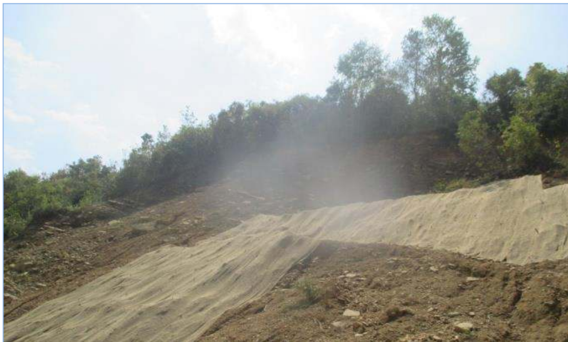
CH. 0+050 RHS, SLOPE STABILISATION BY JUTE NETTING
