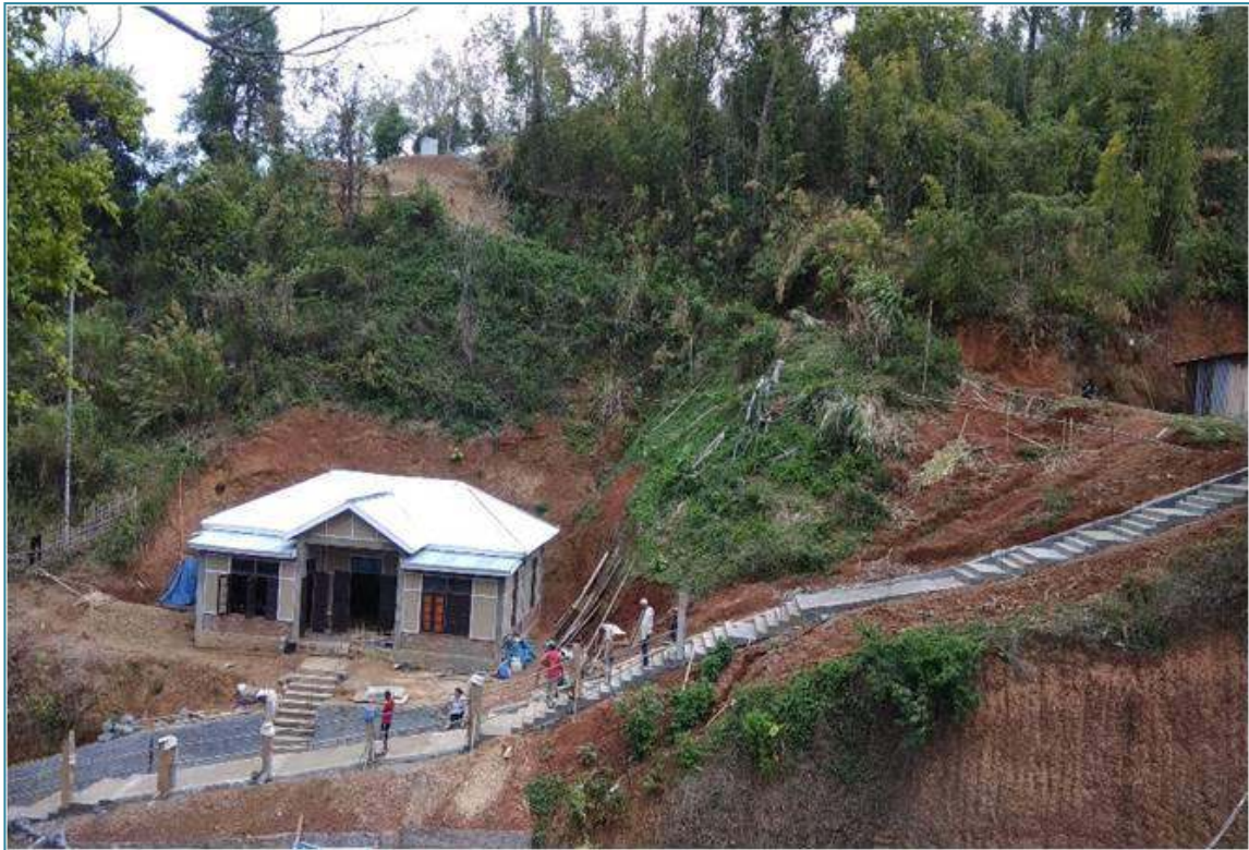
Construction of Concrete step to Church at Rangte village
