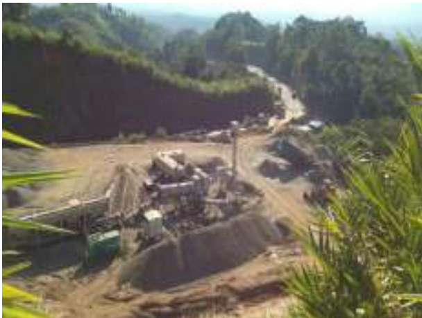
19. 103.35 - 44A Tuidam Plant
