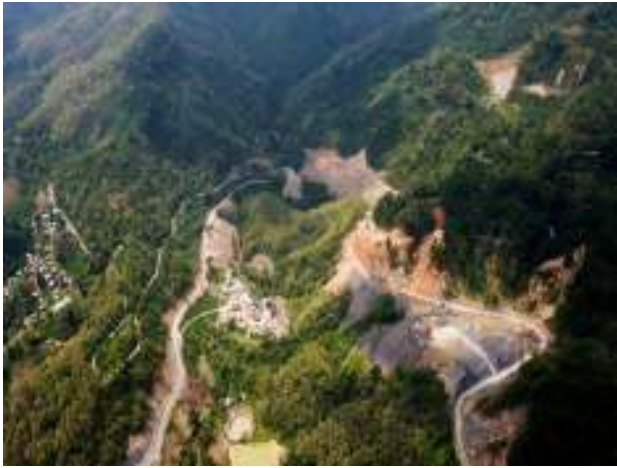
8. 47.300 - 44A Dapchhuah, W.Phaileng Junction, Daplui Bridge Site, Dampui Diversion Inlet.
