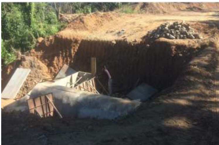
HP Culvert at chainage 53.28 Kmp
