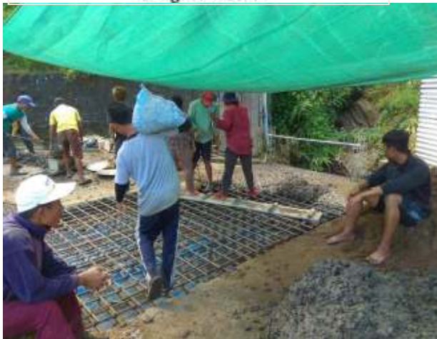
(9) Re-Construction of Collapsed RCC Slab Armed Veng South to Bethlehem Venghlang. Length : 1.00
