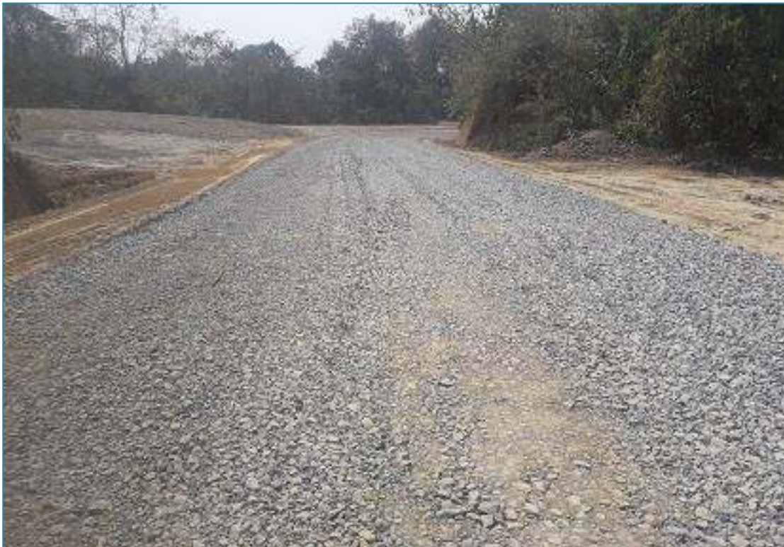
Ch 7+970 to 8+200, Laying of WBM grade 1
