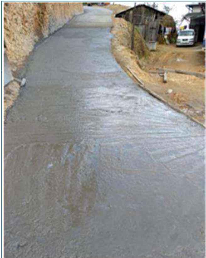
Improvement of Aibawk - Darlung Road (32.00 km) including approach road to Cemetery and supply godown at Darlung
