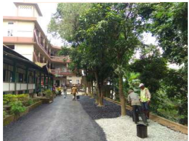
(4) Resurfacing of Approach Road to Govt. Mizo Higher Secondary School at MC Donald Hill. Length : 274.00
