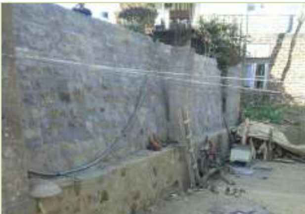
Construction of R/Wall on Durtlang Lower Lane road at Ch: 1.670kmp. Total Length = 10.00M.
