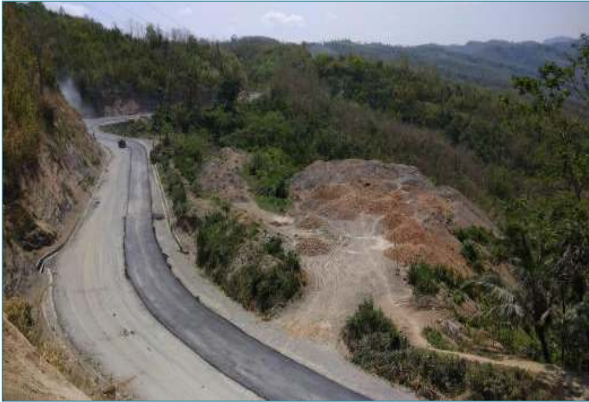
CH 0+470 RHS, DBM LAID
