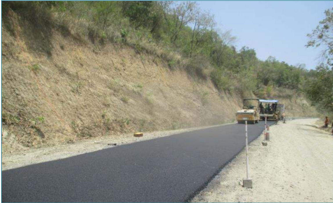
CH. 6+500-6+540, LAYING OF DBM
