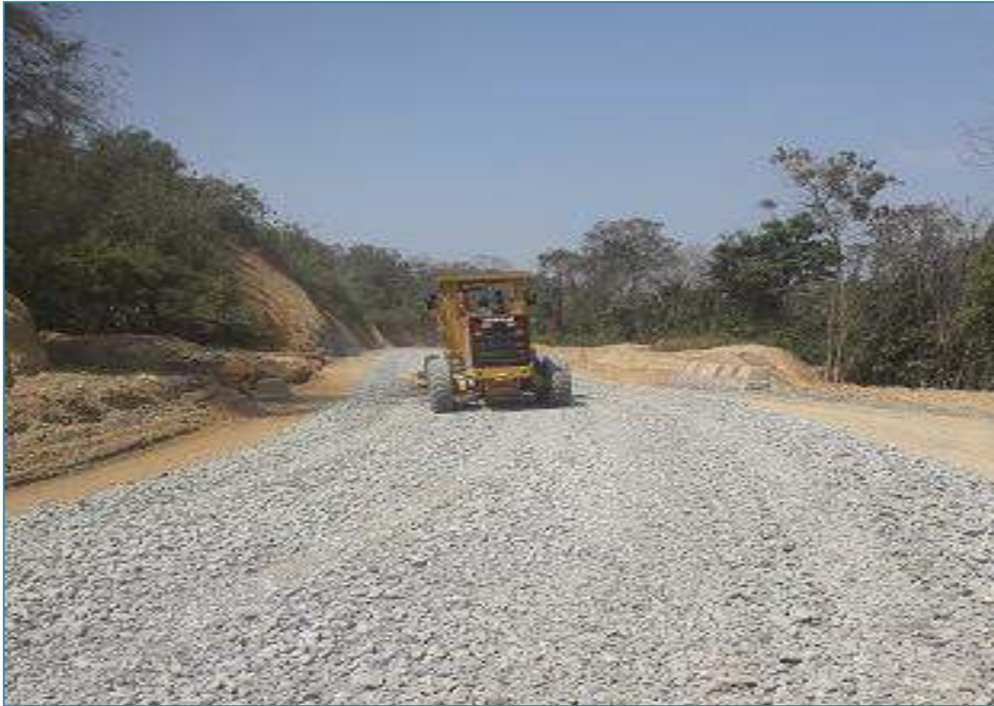
Ch 7+800 to 7+920, Laying of WBM grade 1
