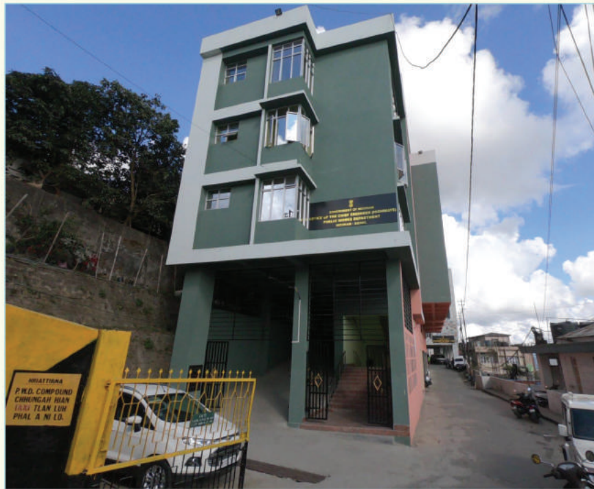
Office Building of CE Highways, Tuikhuatlang
