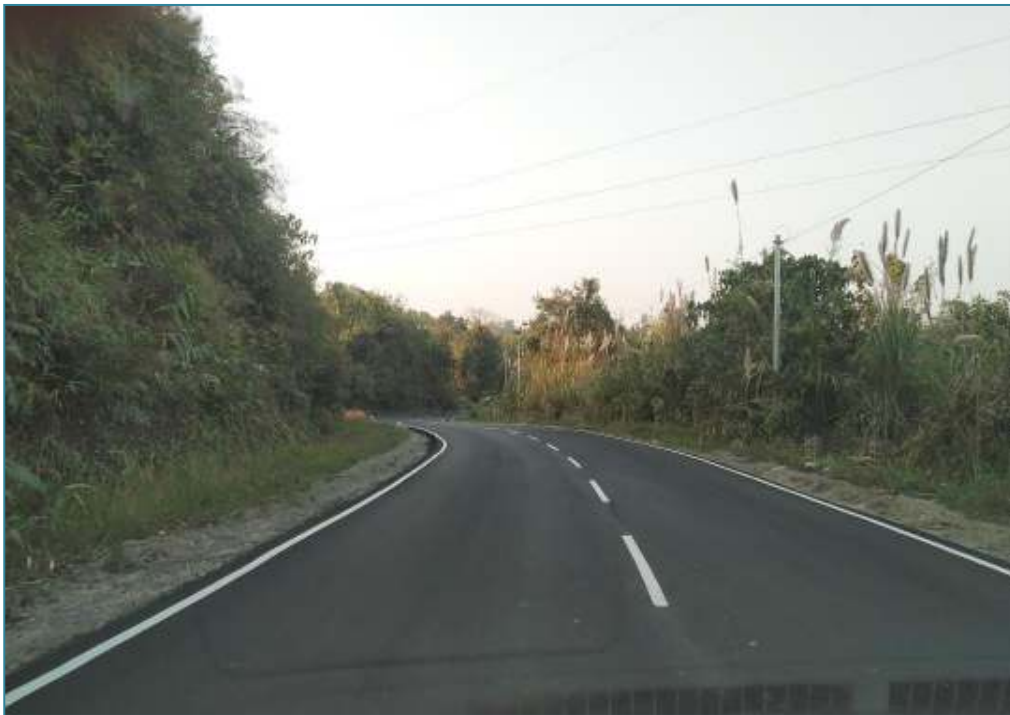
IRQP Works on NH-154
