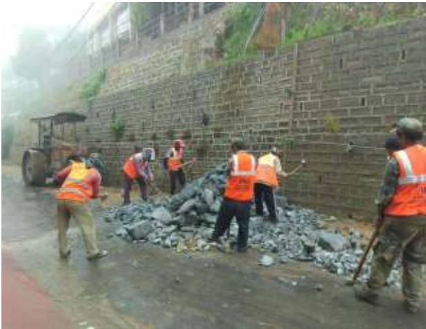
(7) Patch Repair of Approach Road to S.E NHC-II Office PWD at Ramhlun Venglai. Length : 431.00
