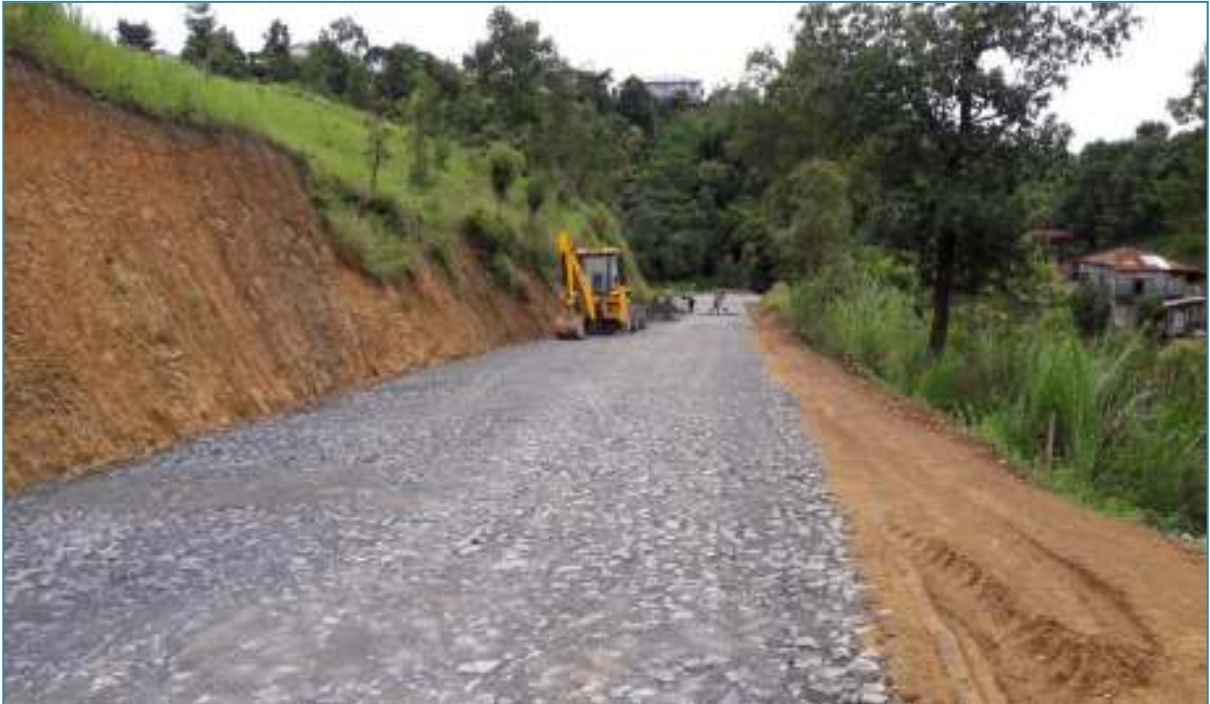
Serchhip – Buarpui Road: WBM Grade-I
