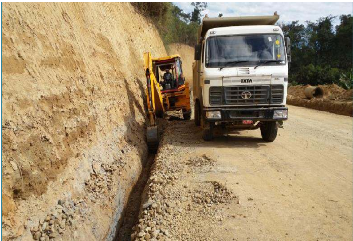
Ch 9+200 ROAD SIDE DRAIN – EXCAVATION IN PROGRESS
