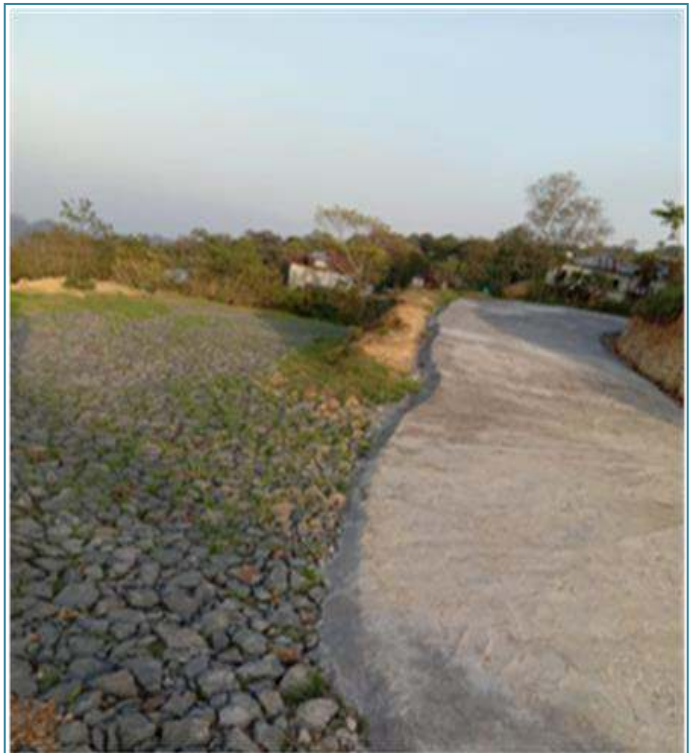
Cell Filled Concrete at Hmuifang Village
