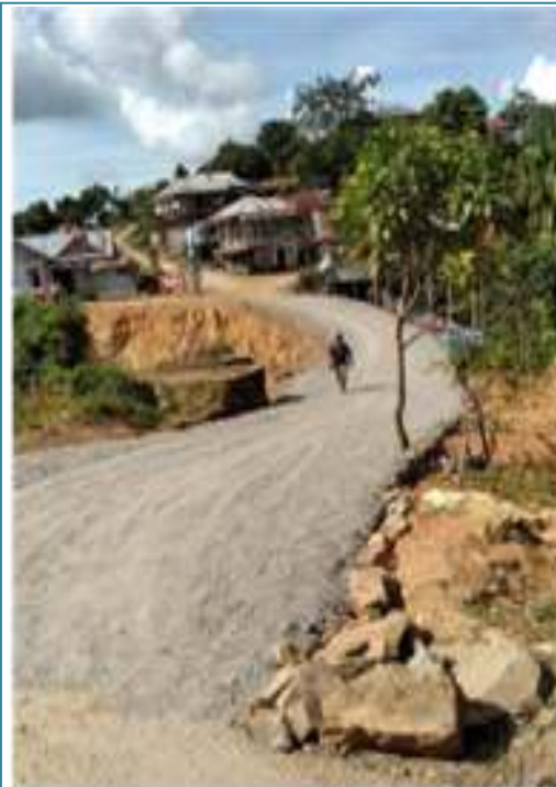
Temporary Restoration of Collapsed road Formation within Darlung Village at Junction Point of Aibawk - Darlung Road
