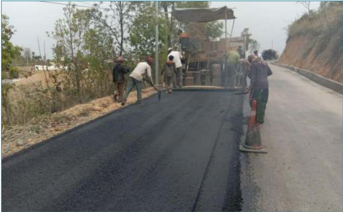
Serchhip – Buarpui Road: Construction of BC in progress
