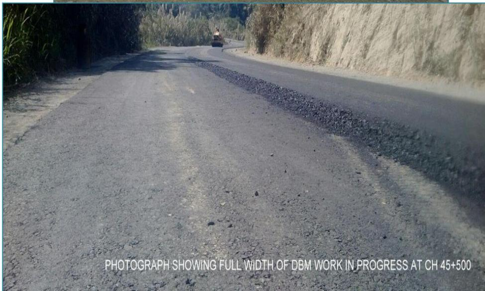
PHOTOGRAPH SHOWING FULL WIDTH OF DBM WORK IN PROGRESS AT CH 45+500
