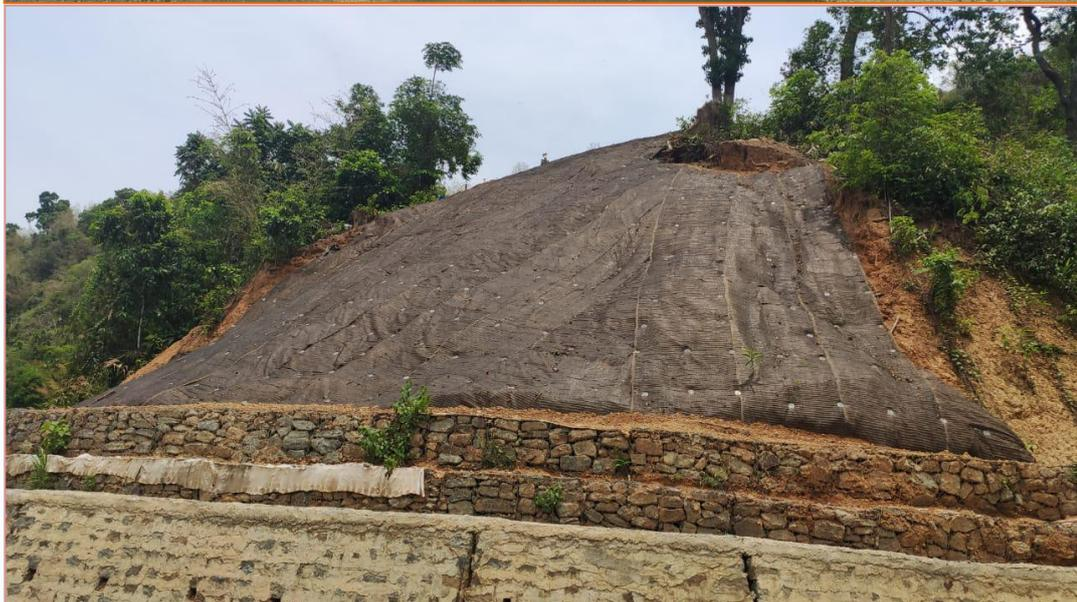
**CH 0+650 : Slope stabilization with Terra-lock, anchor and erosion control**
