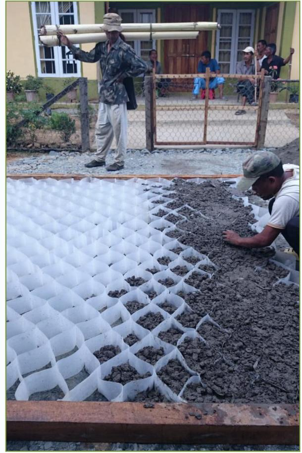
**Execution of Cell Filled Concrete Pavement on S. Vanlaiphai to Muallianpui Road**
