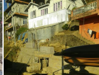
Pavement of BSNL to BRTF road with RCC Slab Culvert at Ch: at 6.615kmp Durtlang Total Length = 617.20 M
