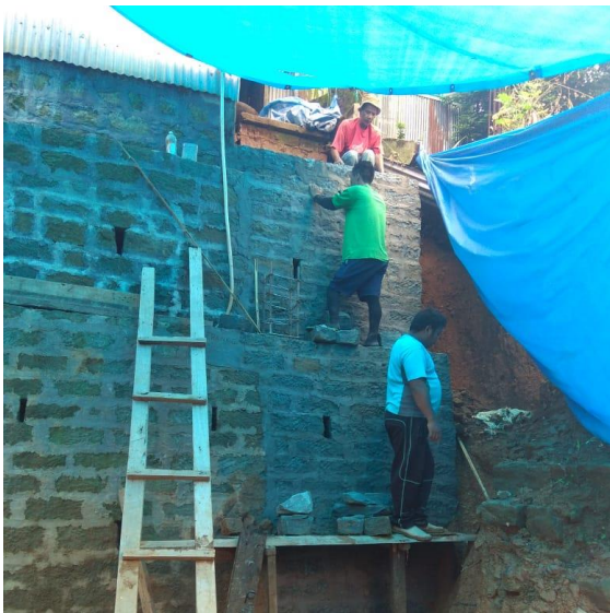
(3) Construction of B/Wall on Elim Road at Chhinga Veng. Length : 13.00
