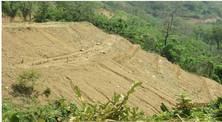
CH 5+650 (DUMPING AREA) RHS --- Bio- Engineering Demonstration for Slope Protection (Bamboo Crip
