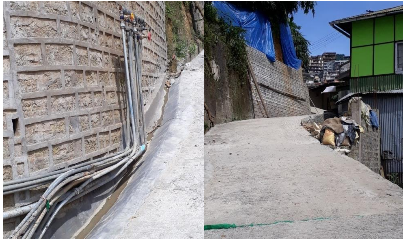
Construction of Jeepable Road from Khatla South Church to Khatla East at Aizawl.
