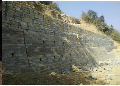
Construction of Masonry Retaining Wall and Gabion structure R/Wall on approach road to Assam Rifles Complex at Zokhawsang at Ch: 0.230kmp. Length 40.00 Rm.
