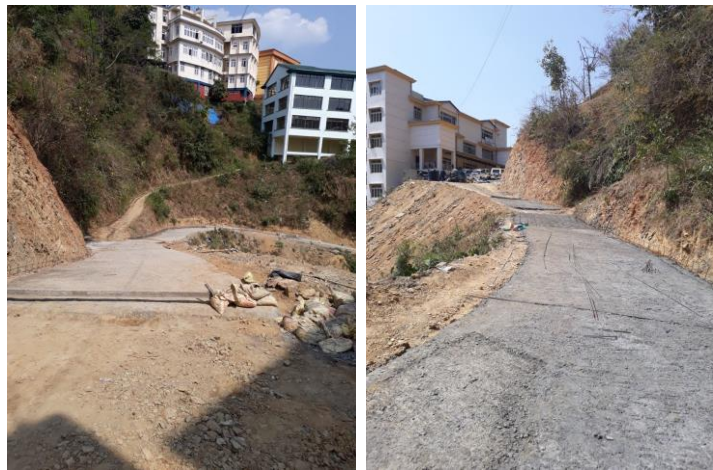
Concrete Pavement from Bungkawm Vengthar to District Revenue Office, New Secretariat Complex.
