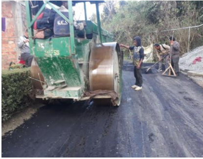
Resurfacing of approach road to Synod Hospital upto Gate Total Length = 1000.00M.
