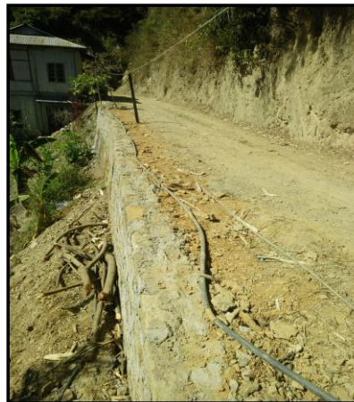
Construction of R/Wall near Pu Zahnuna's house on approach road to Theihai Huan at Thuampui.
