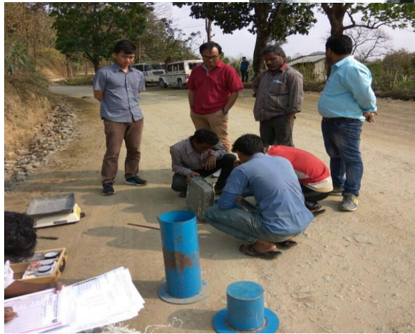
Checking of Granular Sub-Base (GSB) density at Ch.8+000, Part-I
