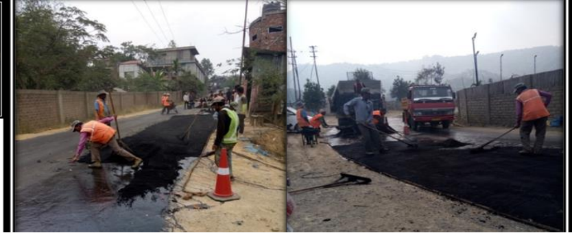
Repair of Potholes with Full Seal Coat on Aizawl Bypass Road at Ch 0.00-2.00 kmp.
