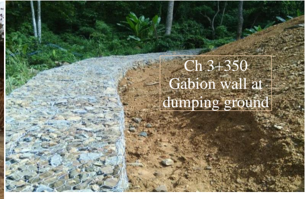
Bank Protection with Gabion structure
