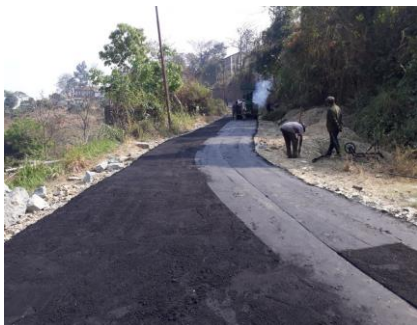
Pavement from Quality to Mechanical Sub Division, Total Length = 486.50 m
