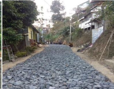
Pavement of BSNL to BRTF road with RCC Slab Culvert at Ch: 6.615kmp at Durtlang Total Length = 617.20 M
