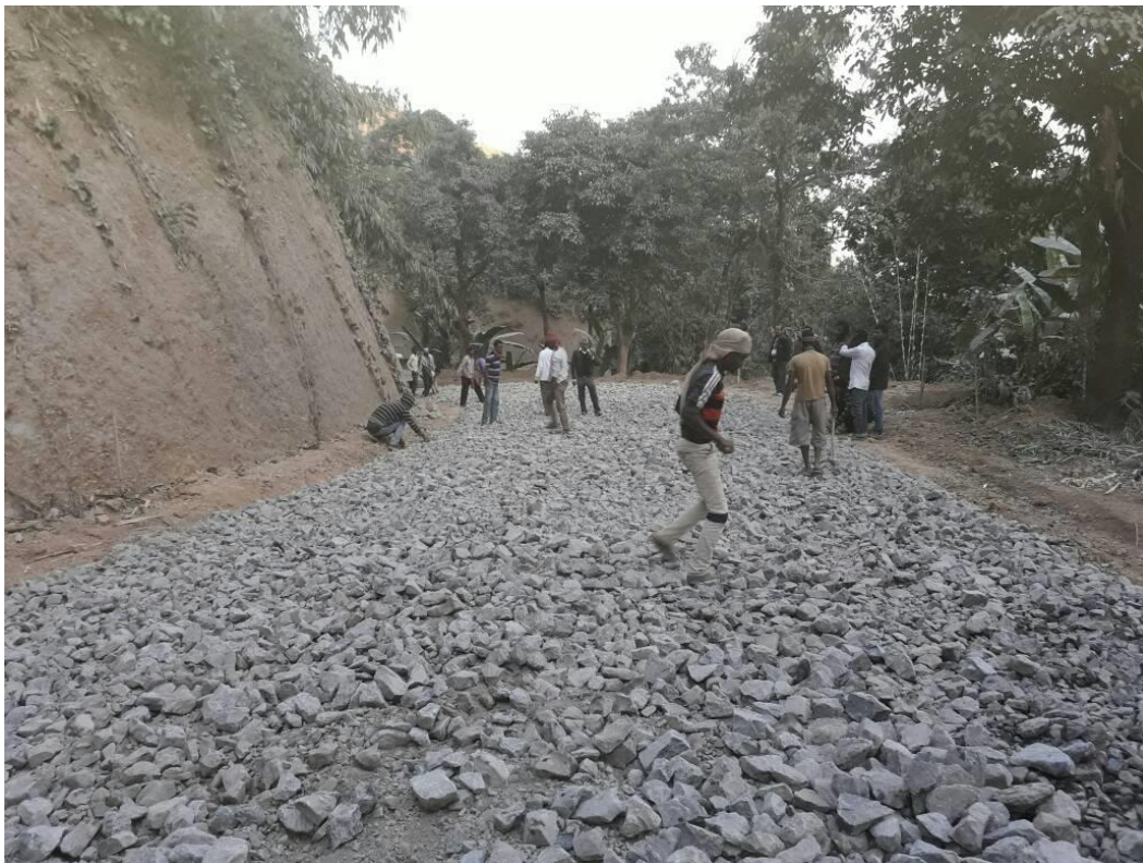
Laying of Granular Sub-Base(GSB) in Part-I
