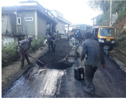
Resurfacing of approach road to Synod Hospital upto Gate. Total Length = 1000.00M
