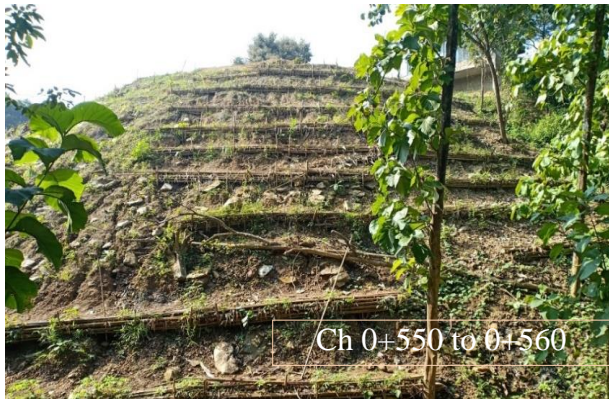
Ch 3+450 Bamboo palisade walls with brush layers at dumping location.
