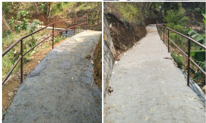
Construction of Cement Concrete Pedestrian Footpath on Approach Road to NSC Presbyterian Church.
