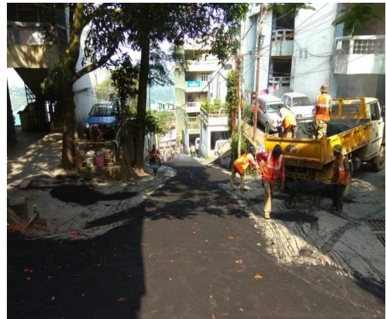
(8) Patch Repair of Zarkawt to Babutlang Approach to Govt. Quater's. Length : 450.00
