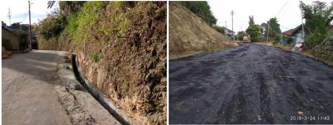
Some resurfacing works within ARSD
