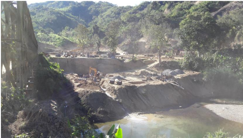
Preparation of test Piles at Tlawng River Bridge Site, Part-II
