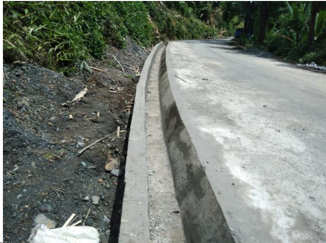
Completed Side Drain in Part-I
