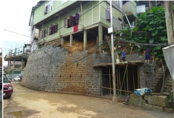
(2) Construction of B/Wall Below Pu Lalthantluanga's House on Armed Veng to Electric Veng Cemetery at Chhinga Veng Length : 18.00
