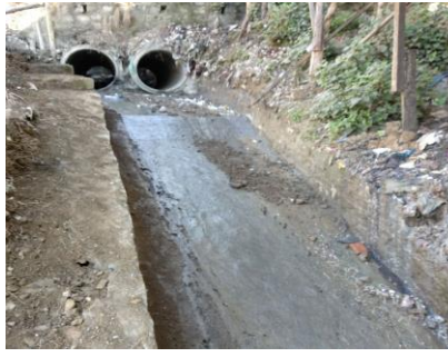
Construction of Link Drain on Down hill side culvert at entrance of Brigade Field approach road. Total Length = 31.00Rm.
