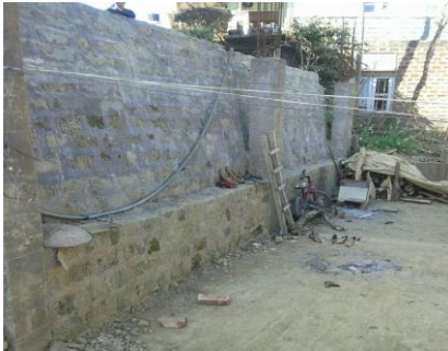
Construction of R/Wall on Durtlang Lower Lane road at Ch: 1.670kmp. Total Length = 10.00M.
