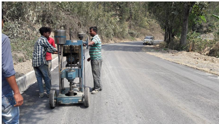
Testing of DBM in Part-I
