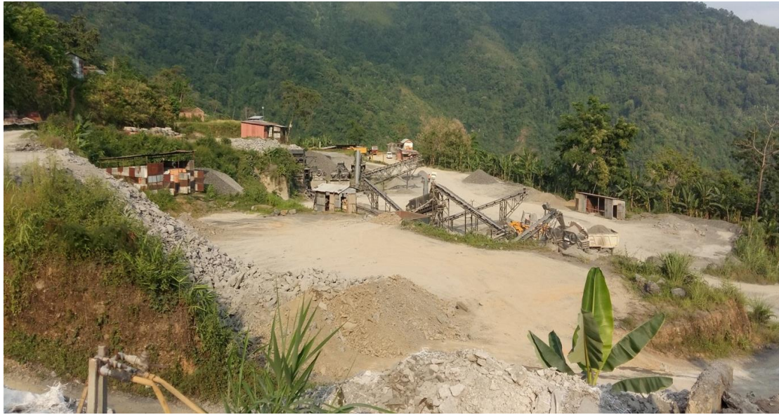
Contractor's Crushing plant
