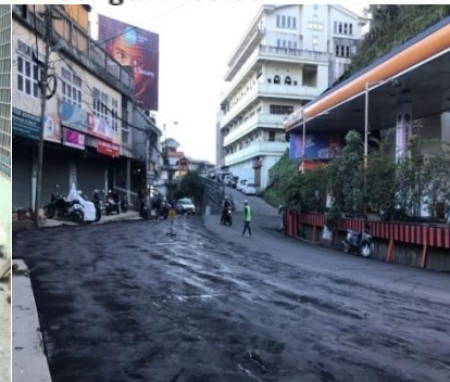
(11) Patch Repair and Seal Coating of Bawngkawn to Chanmari via Ramhlun Length : 3500.00
