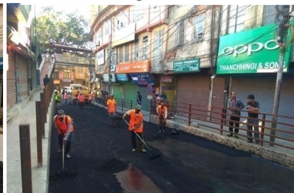
(6) Patch Repair and Sela Coating of Bazar Bungkawm to Millenium Centre Length : 420.00
