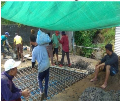
(9) Re-Construction of Collapsed RCC Slab Armed Veng South to Bethlehem Vengthlang. Length : 1.00
