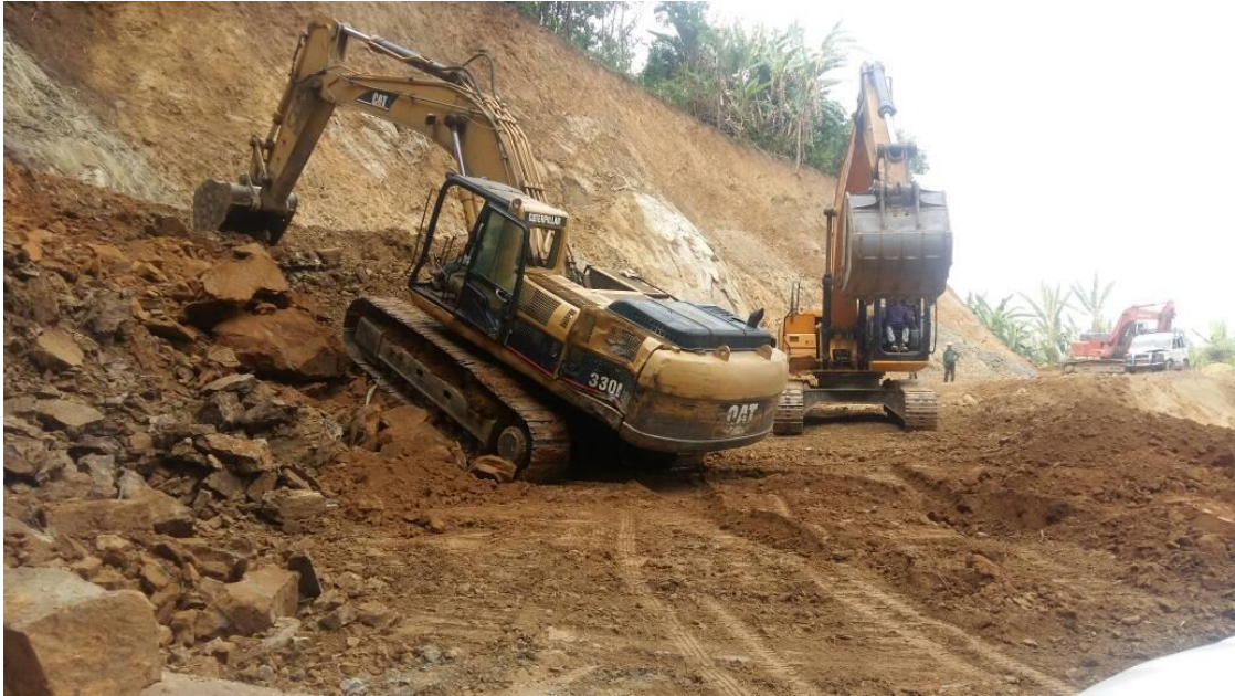
On-going excavation in Part-II
