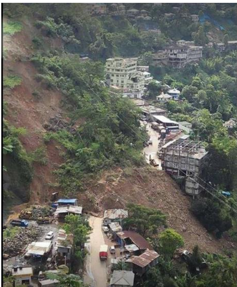
Landslide on the road
