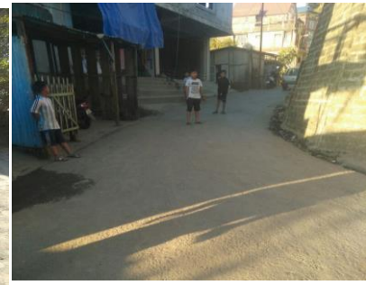
Resurfacing of Thingkhim to Galilee veng at Zemabawk Total Length = 680.00 M
