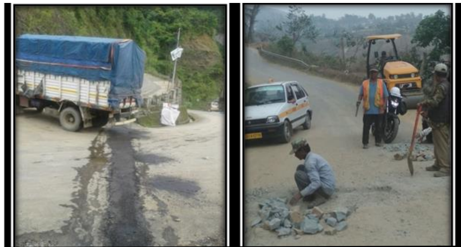
Resurfacing works within Aizawl Road South Division. (Repair of Bad Patches and Potholes on Aizawl Bypass Road).
