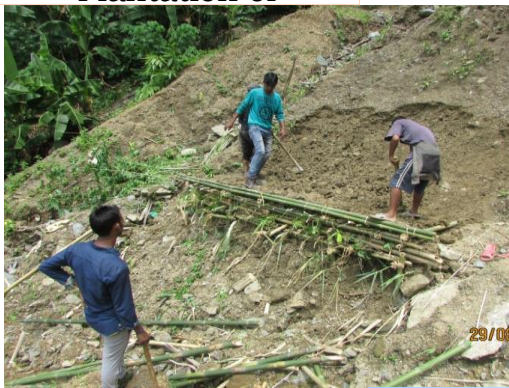
CH 7+950 Construction of Bamboo Crip Work & Plantation of
