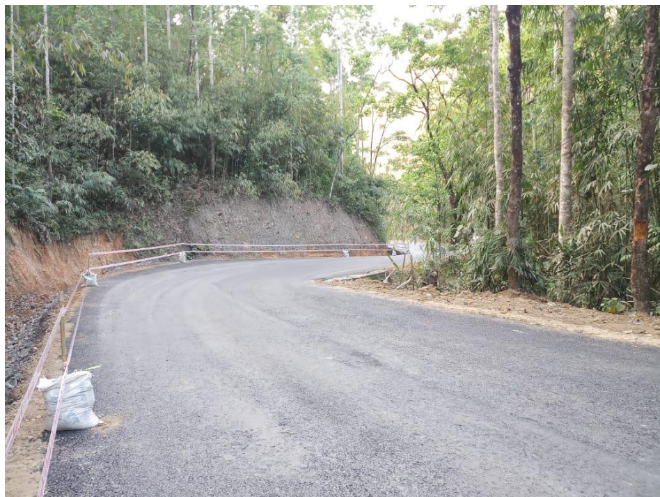
Completed Dense Bituminous Macadam(DBM) at Ch.13+800 Kmp, Part-I
