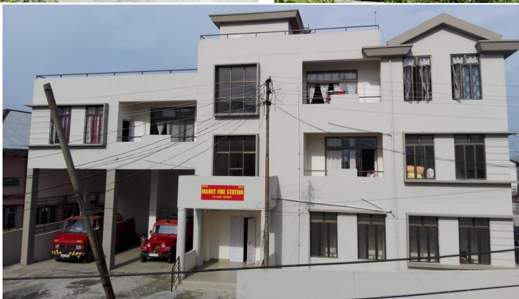
Name of work : Construction of Fire Station Building at Mamit Sanction No : No.D.11014/4/2010-HME Dt.29.01.2015 Sanction Amount : Rs 180.00 lakh Funding source : 13 th Finance Commission (TFC) Date of completion : Dt.20.04.2017 The building was handed over to the Fire & Emergency Service Department on Dt. 25.01.2018
