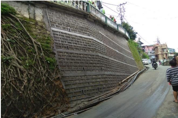
(1) Re Construction of R/Wall on Approach Road to Chief Minister Bungalow from Zarkawt. Length : 14.50
