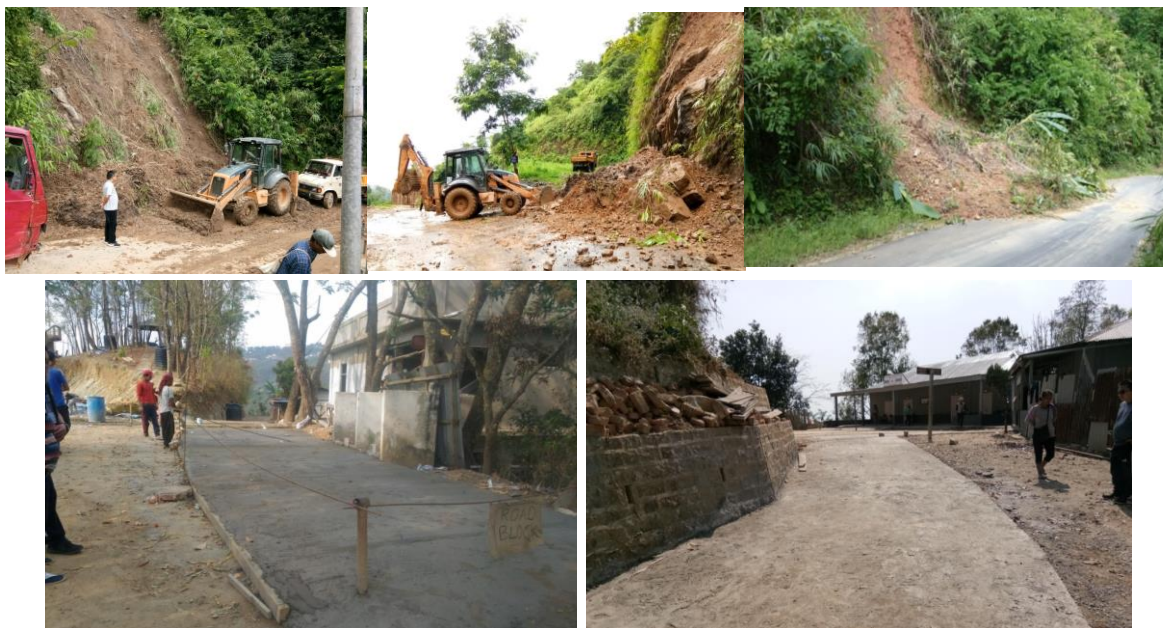
Cement Concrete Pavement of Approach Road to Lawipu Middle School
