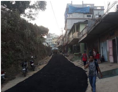
Metalling and Black Topping of Thuampui Internal Road (Lalthanga Road), Total Length = 100.00Rm
