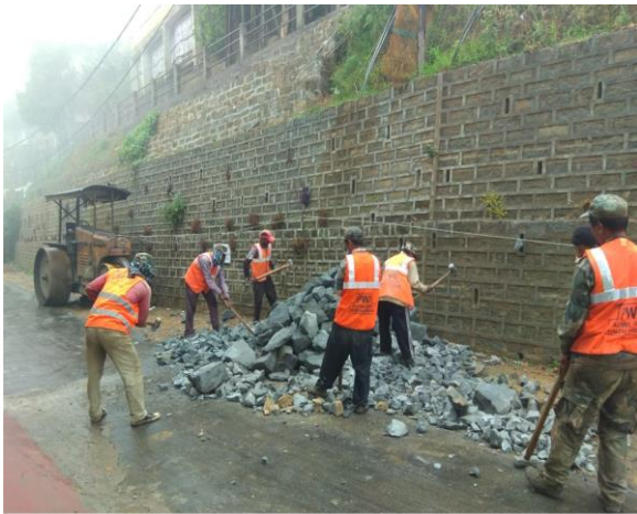
(7) Patch Repair of Approach Road to S.E NHC-II Office PWD at Ramhlun Venglai. Length : 431.00
