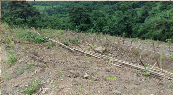
CH 5+650 (DUMPING AREA) RHS --- Bio- Engineering Demonstration for Slope Protection (Bamboo Crip
