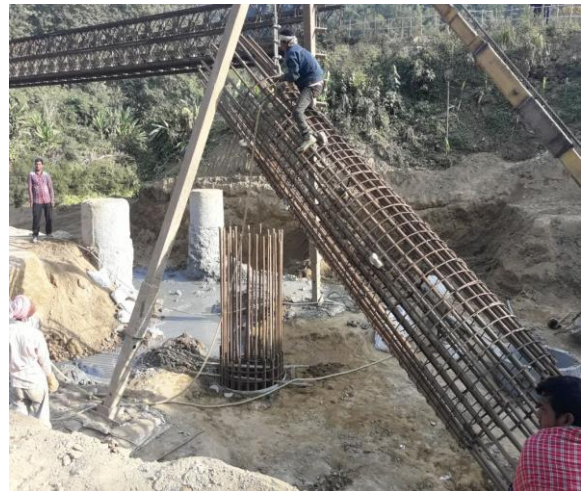
Preparation of test Piles at Tlawng River Bridge Site, Part-II
