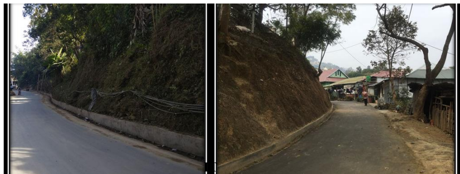
Patch Repair of ITI Ring Road (near Presbyterian Church)
