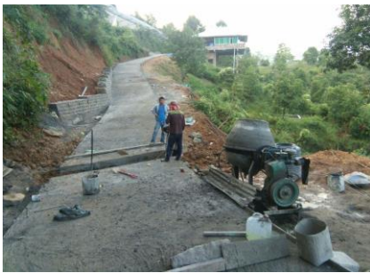
Concrete Pavement for approach road to Bawngkawn 'S' Cemetery at Durtlang Ramthar Total Length = 600.00M.
