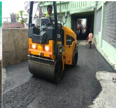
(10) Re-Surfacing of Chhinga Veng Internal Road Length : 750.00
