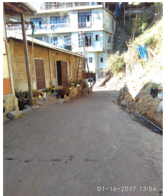
Repair of Bad Stretches and Seal Coating of Approach Road to CID complex and YMA Road at Bungkaxen
