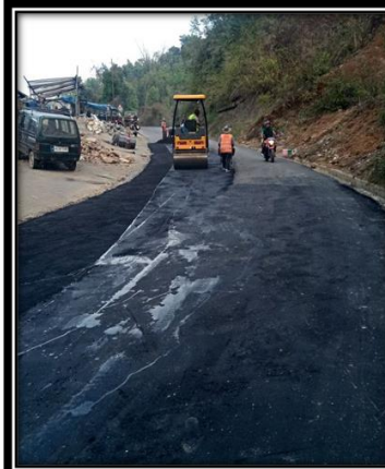
Repair of potholes with full sealcoat on Aizawl Bypass Road, Ch 2.00-4.00 km \phi (L=2 km, Rs 30 Lakhs, R&B).
