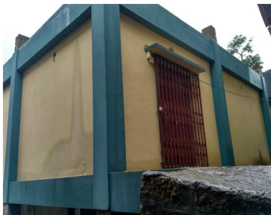
Construction of Warehouse for EVM and VVPAT at Lawngtlai
