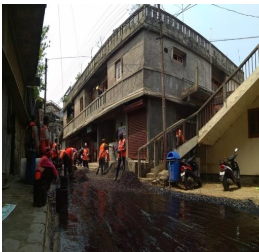
(1) Laying of Paver Block Dawrpui Cemetry Internal Road (Upper Lan). Length : 225.00
