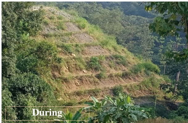
Ch 3+450 Bamboo palisade walls with brush layers at dumping location.
