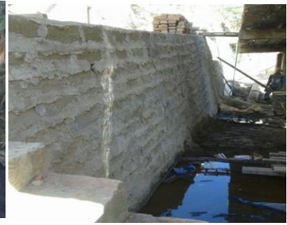
Reconstruction of R/Wall on Chite road at tCh: 0.150kmp near Pastor Biakvumawia's house. Total Length = 22.00 M.
