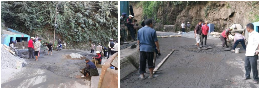
Construction of Concrete Pavement on Khatla Ring Road in front of Nursery Tuikhur at Nursery Veng.
