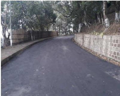
Approach road to ATC with internal roads and main Building Courtyard. TotalLength = 1.717 km,
