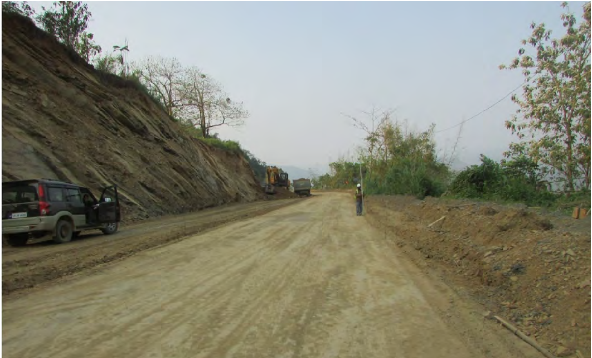
Sub grade Top Layer Km3+990 to 4+130 (C-C Road)
