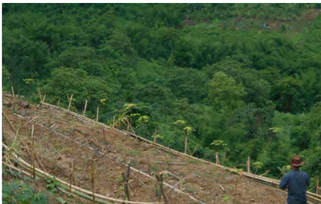
Turfing and Grass Sodds Km 7+950(Dumping) (C-C Road) & Bamboo Crib Wall Km 8+050 (C-C Road)
