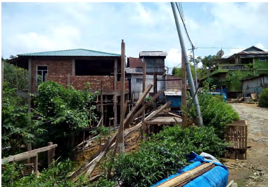
Shifting of Structure for widening of road at Buarpui Village, Part-II.
