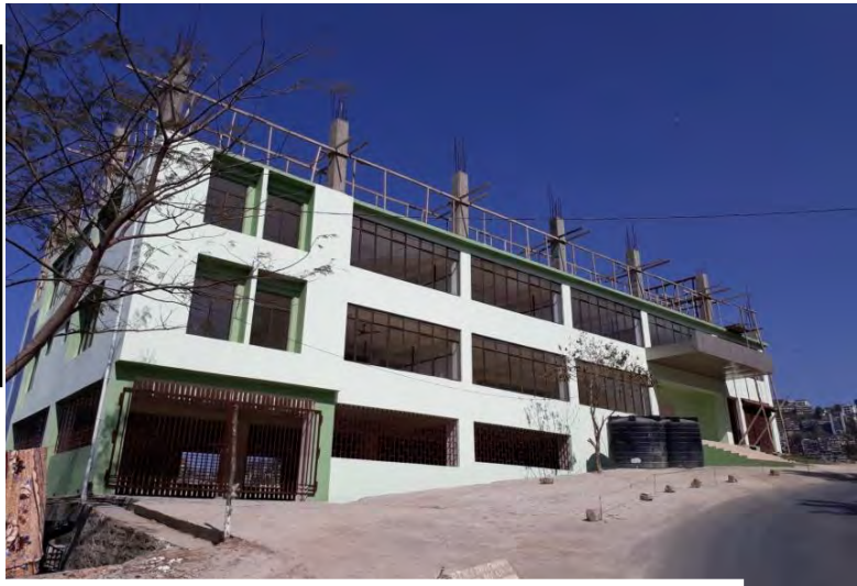
PIC: DIRECTORATE OF TAXATION BUILDING PHASE-I & PHASE-II AT NEW SECRETARIAT COMPLEX, AIZAWL
