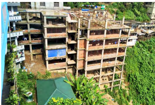
Mission Veng Bazar under construction
