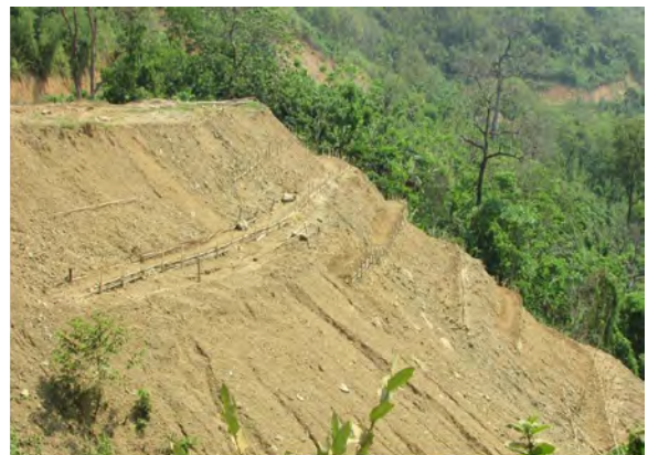
Turfing and Grass Sodds Km 7+950(Dumping) (C-C Road) & Bamboo Crib Wall Km 8+050 (C-C Road)
