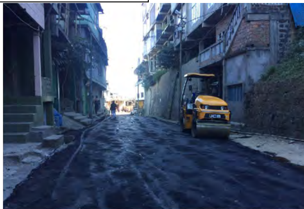
Repair of Bad Stretches and seal coating of full width of Treasury Sq. to Sikulpui Kawn via Upper Republic Rd
