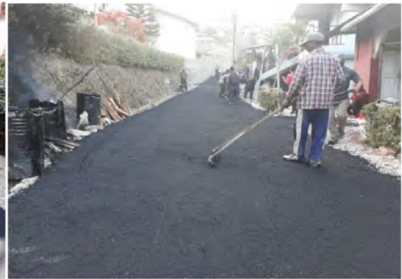
Approach Road to Chhuahlam Tuikhur at Durtlang
