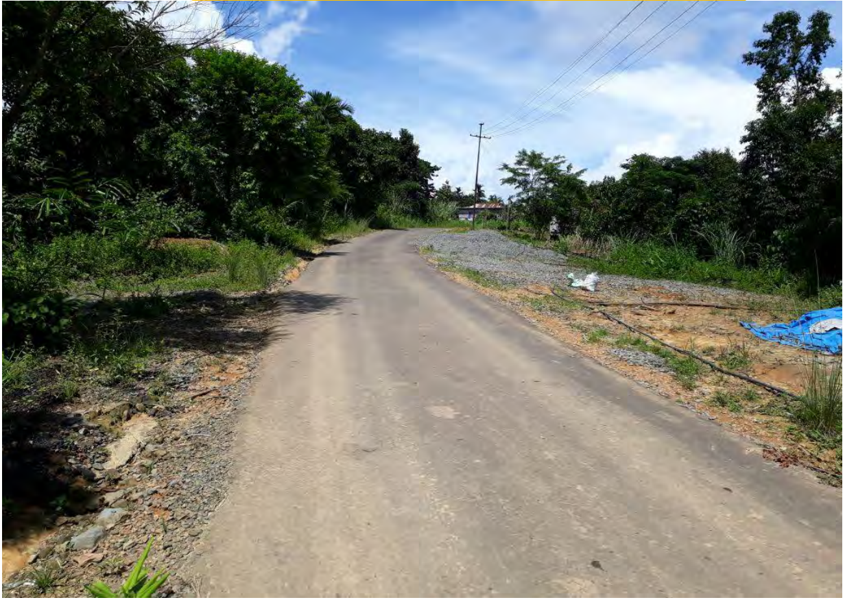
Phairuang to Thenhlum road at 68.500 kmp ( After repairing)
