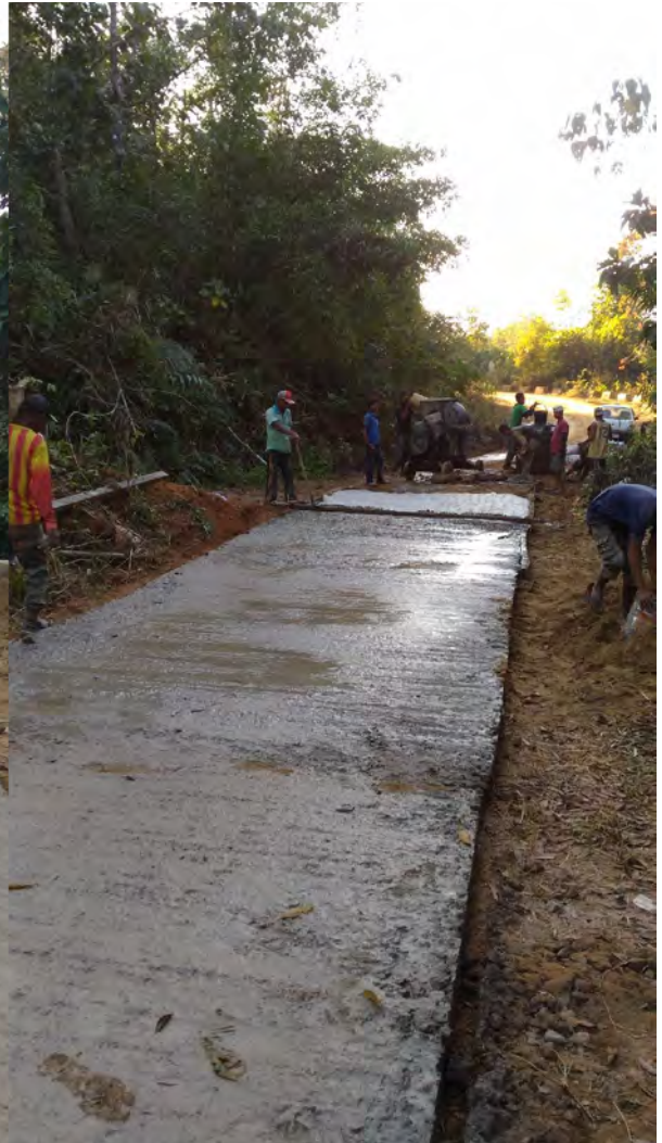
MAUZAM - PUANKHAI ROAD (CELL FILLED CONCRETE PAVEMENT) CHAINAGE AT 2.950 KMP
