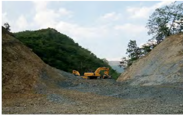
Excavation in progress Km 21+080 (C-Z Road)
