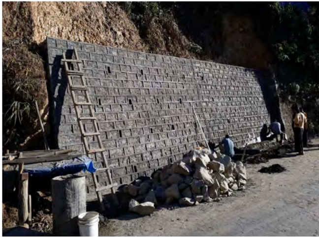
Constn. of Protection Work at Nursery Junction on Khatla Ring Road & Re-Constn. of R/Wall in front of Dinthar Govt. Middle School-II at Dinthar on MHNL Sec-III
