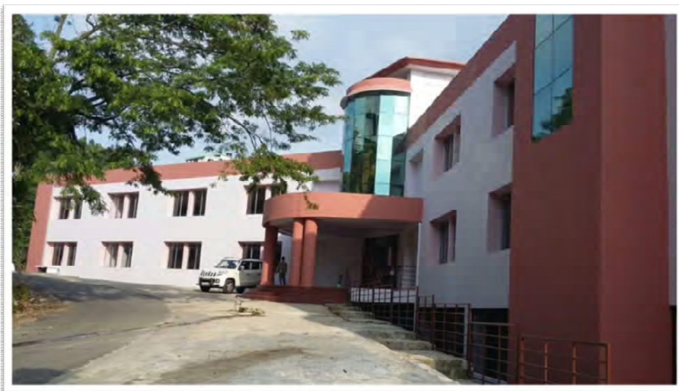
PIC: DIRECTORATE OF HOSPITAL AND MEDICAL EDUCATION BUILDING AT NEW SECRETARIAT COMPLEX, AIZAWL
