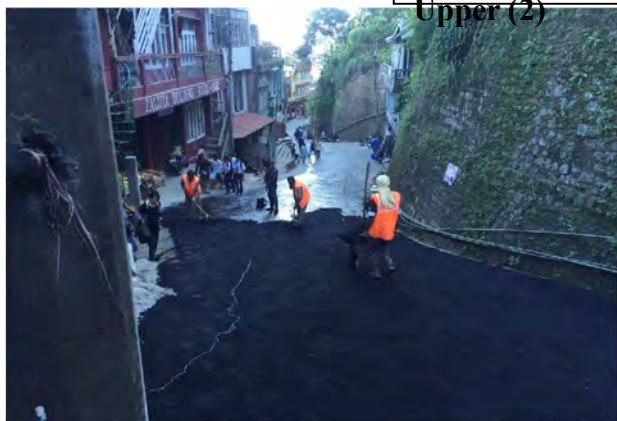
Repair of Bad Stretches and seal coating of full width of Treasury Sq. to Sikulpui Kawn via Upper Republic Rd
