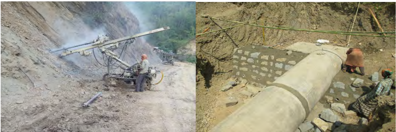
Drilling of hard rock for blasting in progress in Part-II & Construction of Hume pipe in progress at Ch. 7+168, Part-I.
