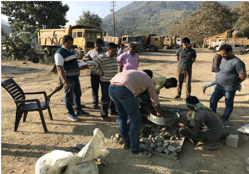
Checking WBM Gradations.
