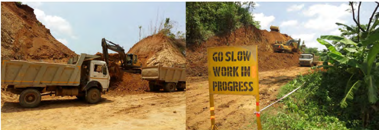
CHAINAGE : 3+600 to 3+660 (Work is in Progress) (T-K Road) & Work in Progress at Chainage 4+140 to 4+210. (T-K Road)
