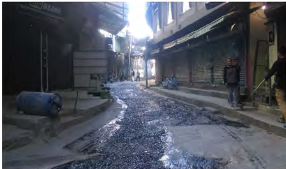
MAINTENANCE OF AIZAWL CITY ROAD UNDER ARND 2016-2017 P/R OF NEW MARKET INTERNAL ROAD
