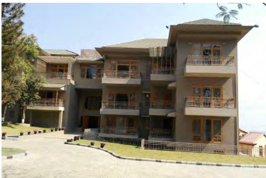
Main Building (Completed)
