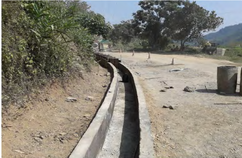
Construction of Side Drain in progress at Ch. 12+600, Part-I.
