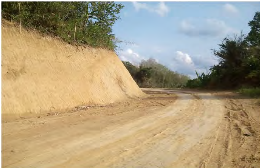
Finished Formation Cutting at Ch. 12+900, Part-II.
