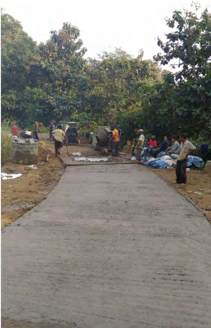
TLABUNG - DIBLIBAGH ROAD (CELL FILLED CONCRETE PAVEMENT) CHAINAGE AT 3.150 KMP
