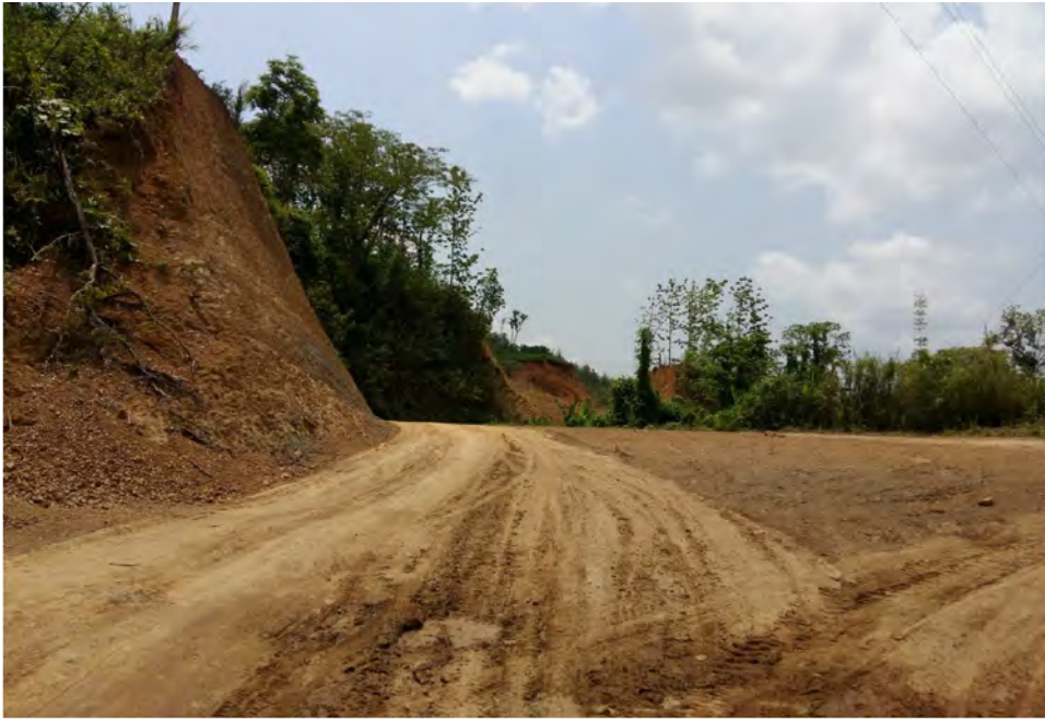
CHAINAGE : 3+530 to 3+580 (Completed Up to Existing Road Level) (T-K Road)
