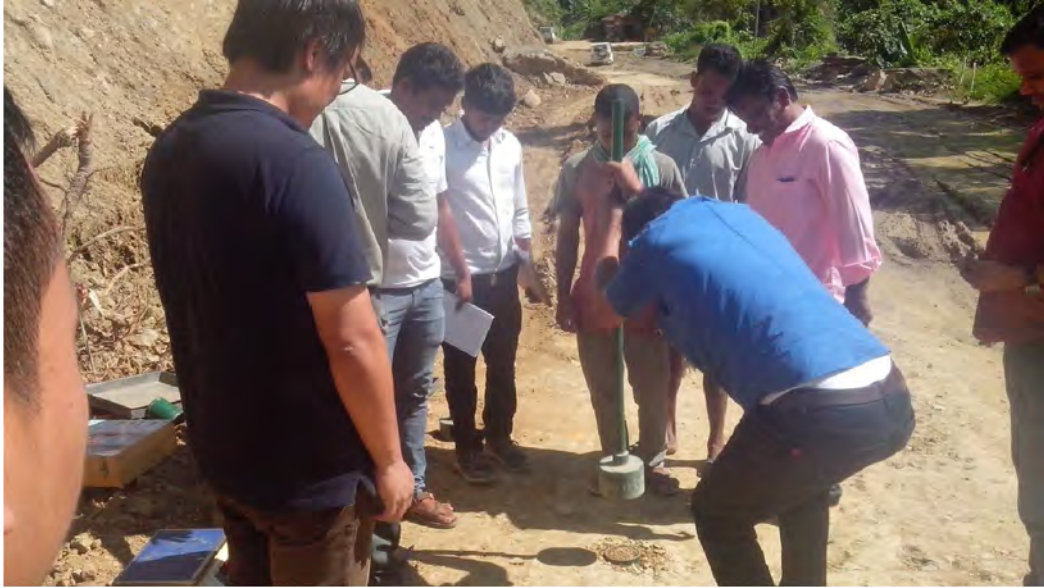
Checking of existing sub-grade density.
