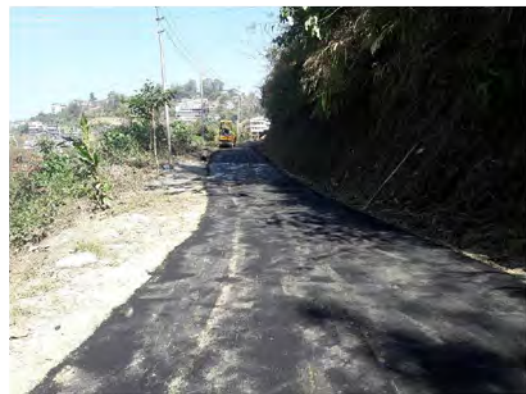
Pavement of PWD Labour Camp & Work Site at New Secretariat Complex
