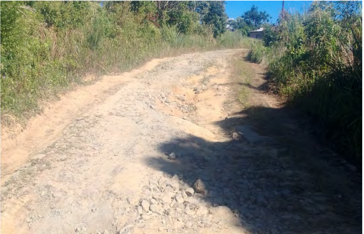
Phairuang to Thenhlum road at 68.500Kmp (Before Repair)
