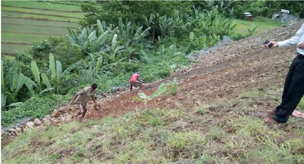
Turfing of Dumping Yard in Progress at Ch 12+500 Kmp Part I.
