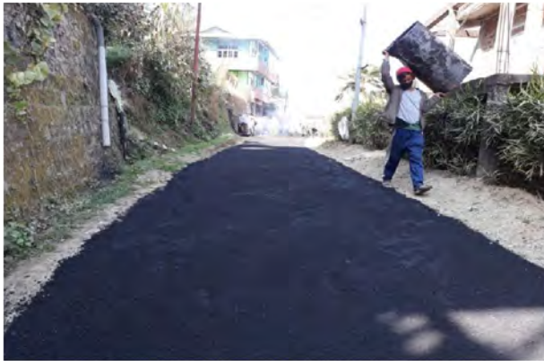
Approach Road to Durtlang Lower Lane
