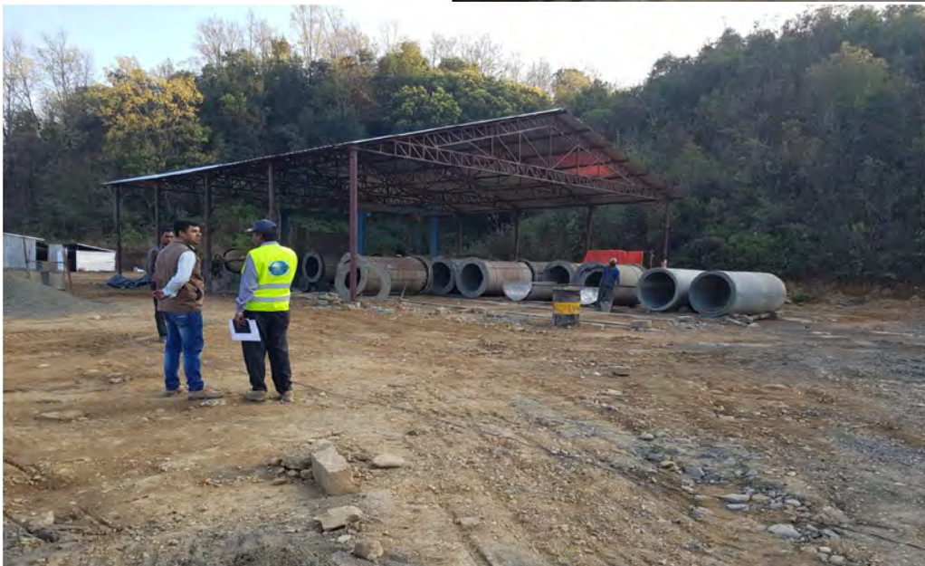
Hume Pipe Manufacturing Plant (C-Z Road)
