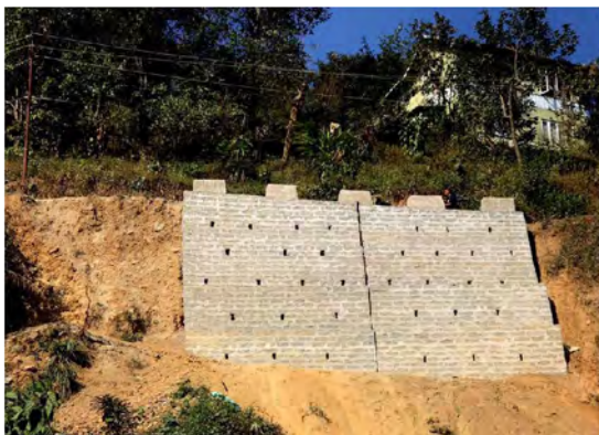
Constn of R/W on Bethlehem Vengthlang to Armed Veng road near Bethlehem Tuikhur
