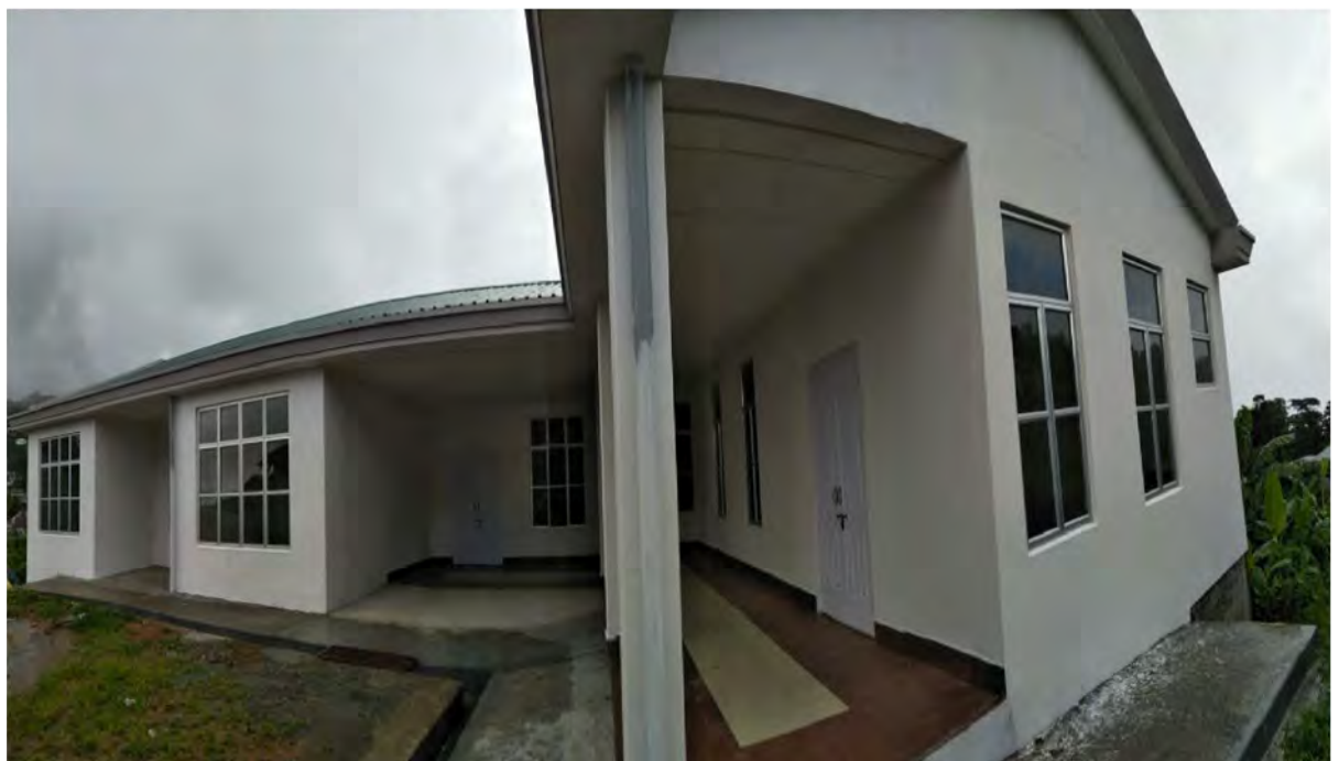
Construction of PHC Building at Bunglemun
