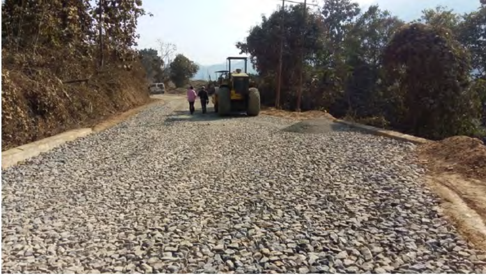
Ch: 12+320kmp Part I WBM Grading-I.
