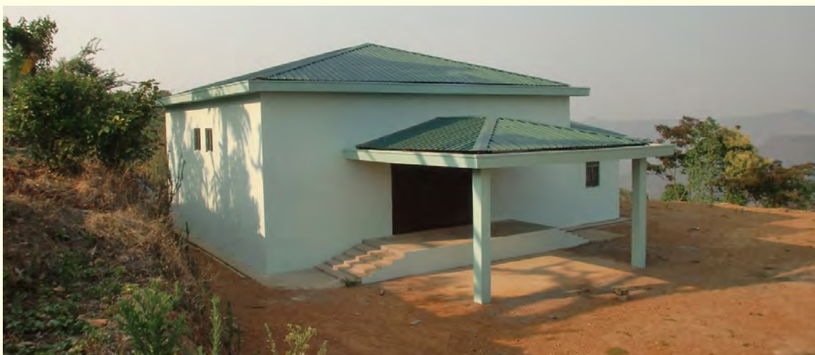
Construction of Storage Godown at Biate
