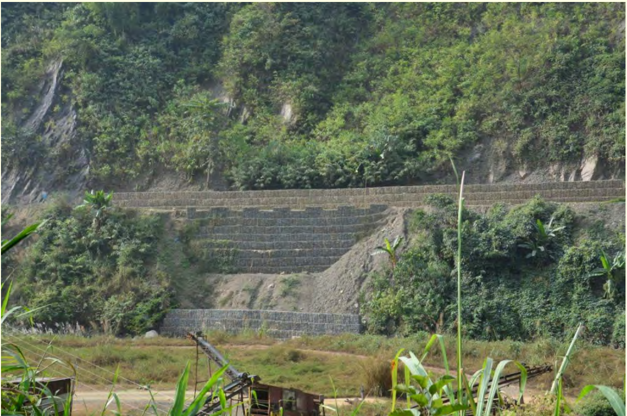
Gabion Walls near River Tuitlawk.
