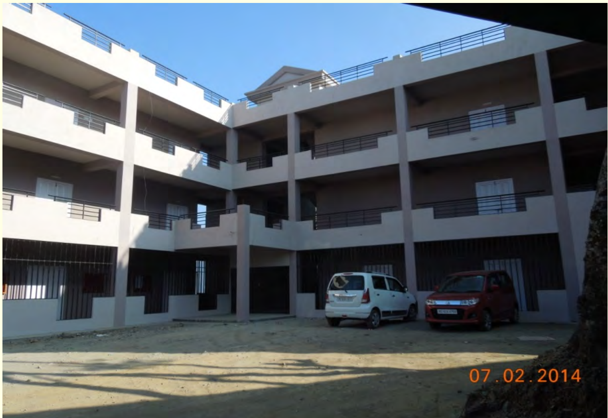
Construction of Govt. J. Buana College at Lunglei
