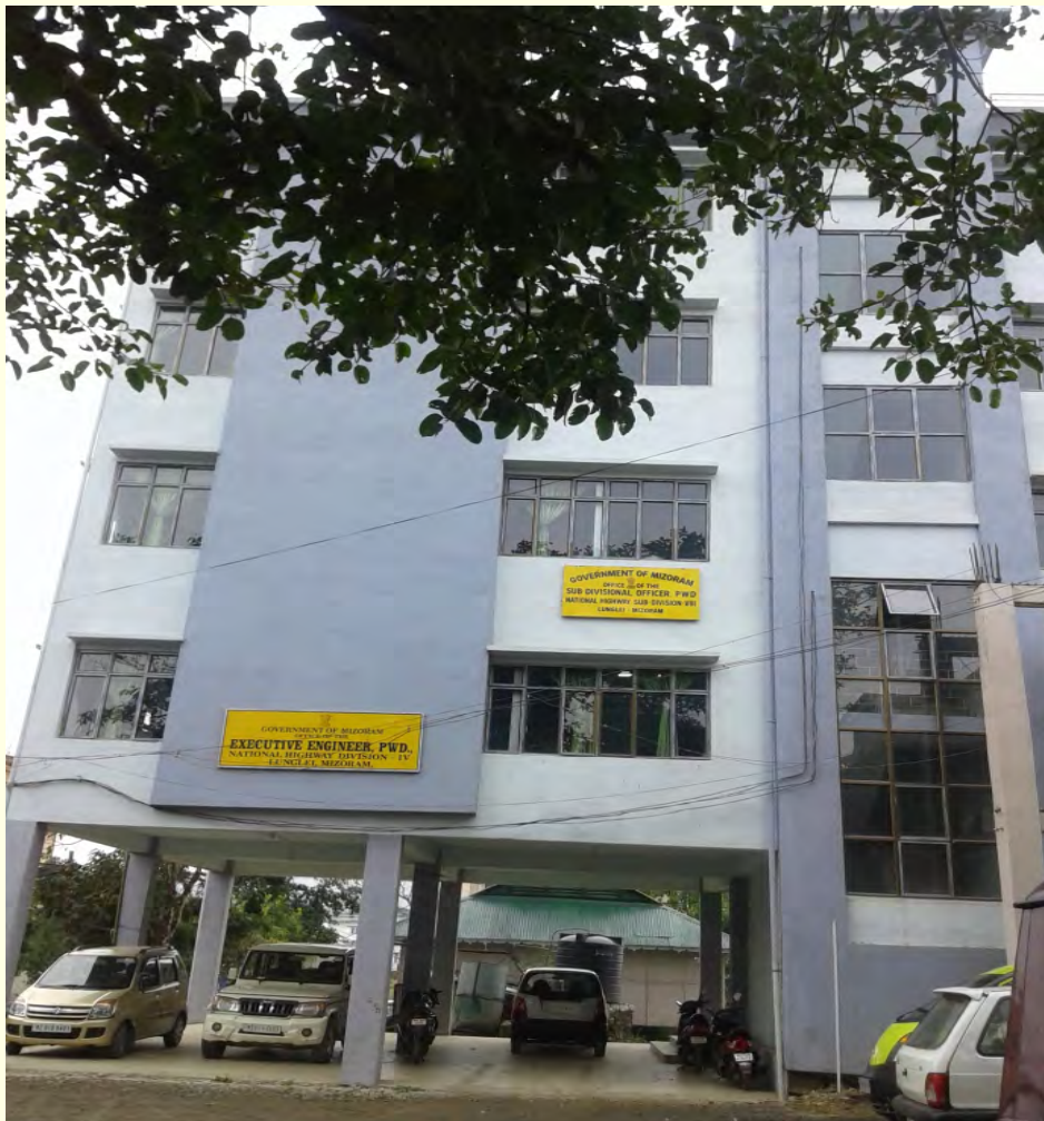
Construction of National Highway Division Office at Lunglei
