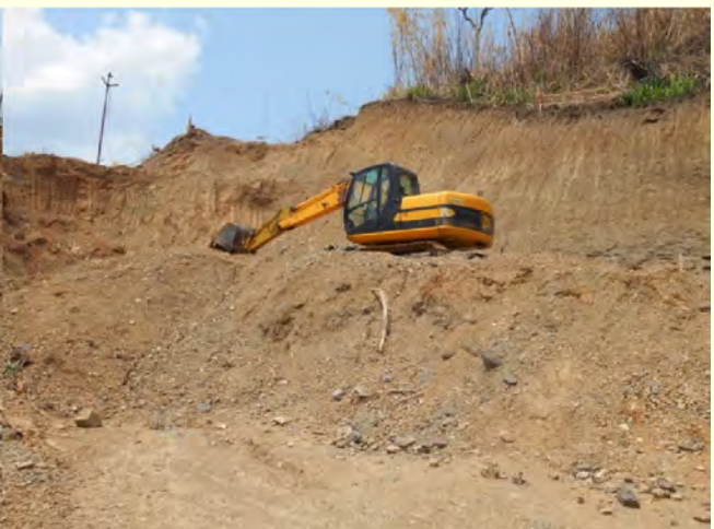
Formation Cutting @ Km 10+300 C-C Road (C-C = Chhungkhum-Chawngte)
