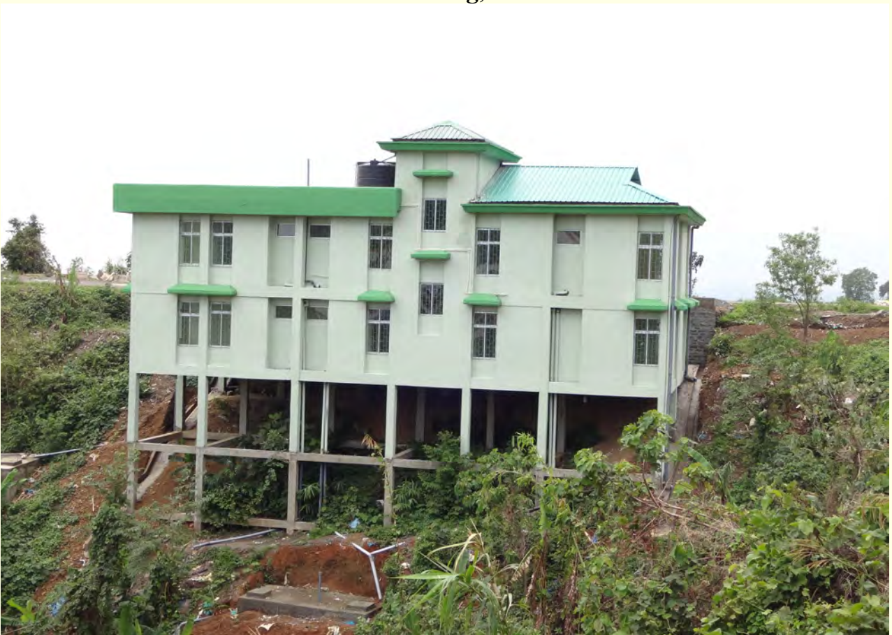
Polytechnic Thingdawl (Administrative Block)
