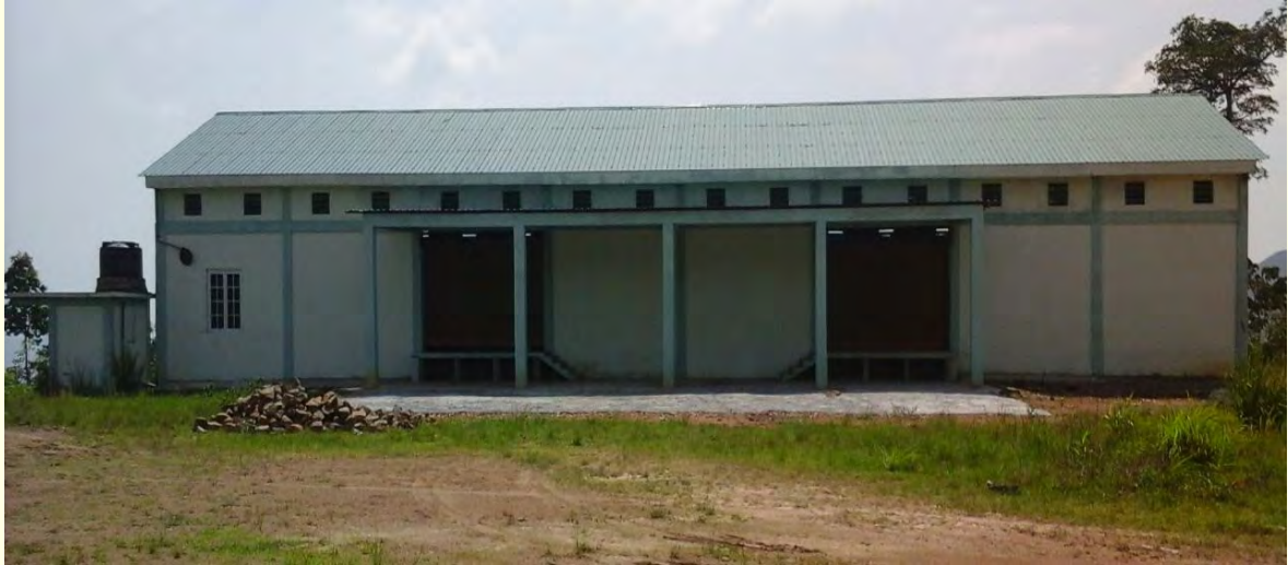
Construction of Storage Godown at Saitual
