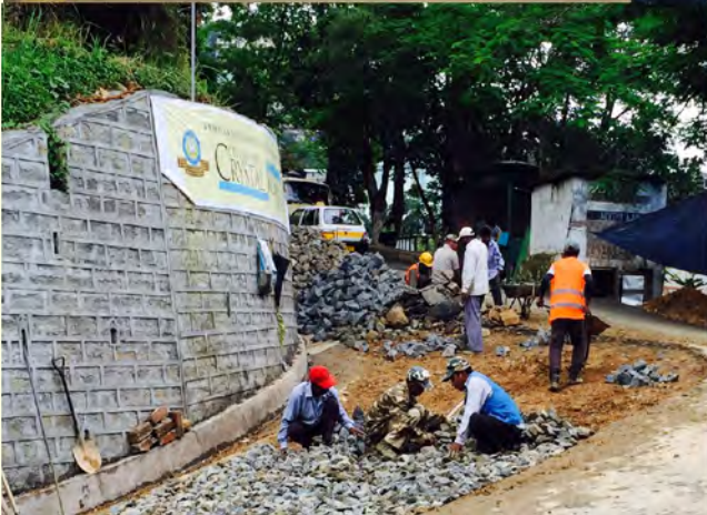
Improvement of works at ITI Junction (1. Grading & Levelling, 2. WBM, 3. Sub Grade Preparation, 4. Pre-mix Carpetting)
