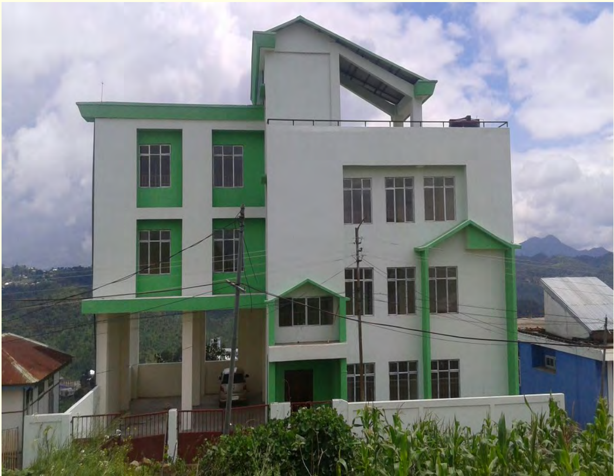
Construction of Fire Station at Champhai
