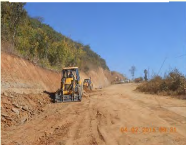
View showing completed formation @ Km 12+100 C – Z Road
