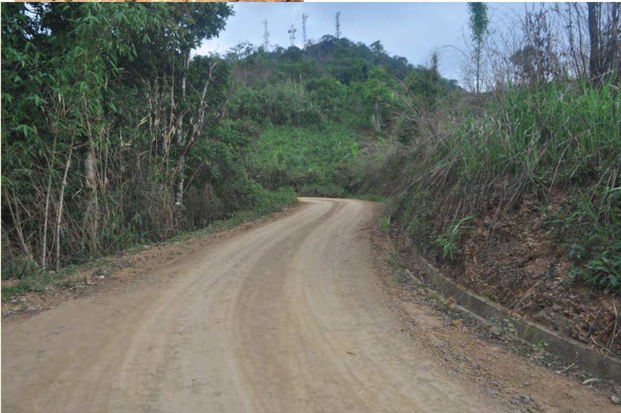
Construction of Thingfal-Mamte Road under PMGSY (Soil Stabilised based with Polymer)
