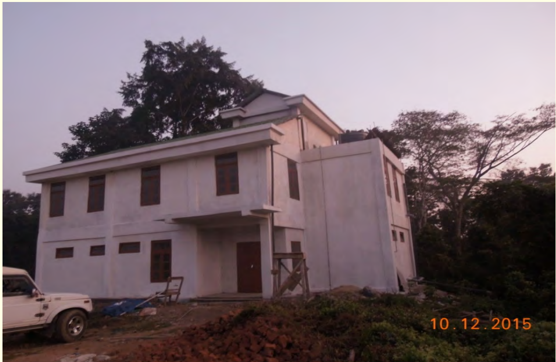
Construction of Police Station of Borapansury
