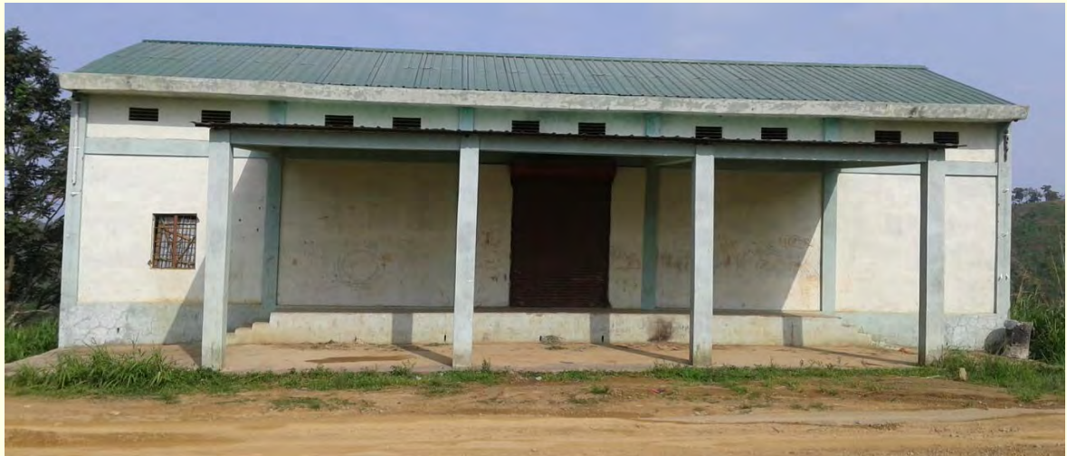
Construction of Storage Godown at Sakawrdai
