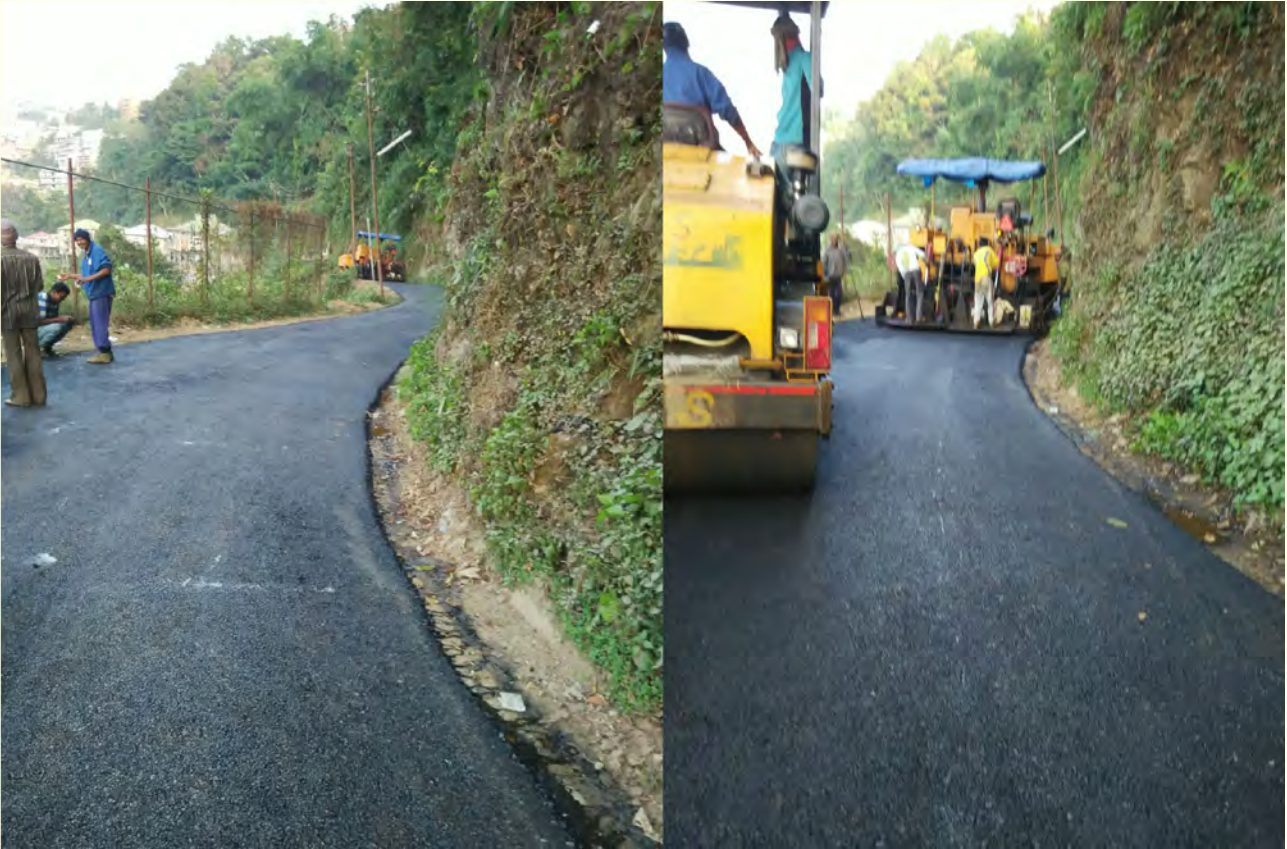
Strengthening & Improvement of Aizawl - Reiek - W. Lungdar Road under CRF
