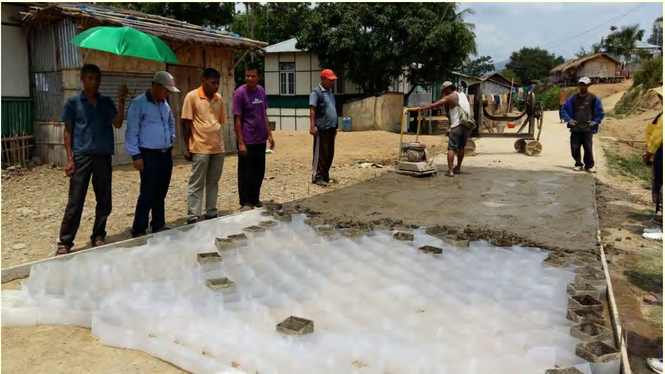
EE, Mamit inspecting Cell-Filled Concrete Pavement of W. Phaileng-Damparengpui Road.
