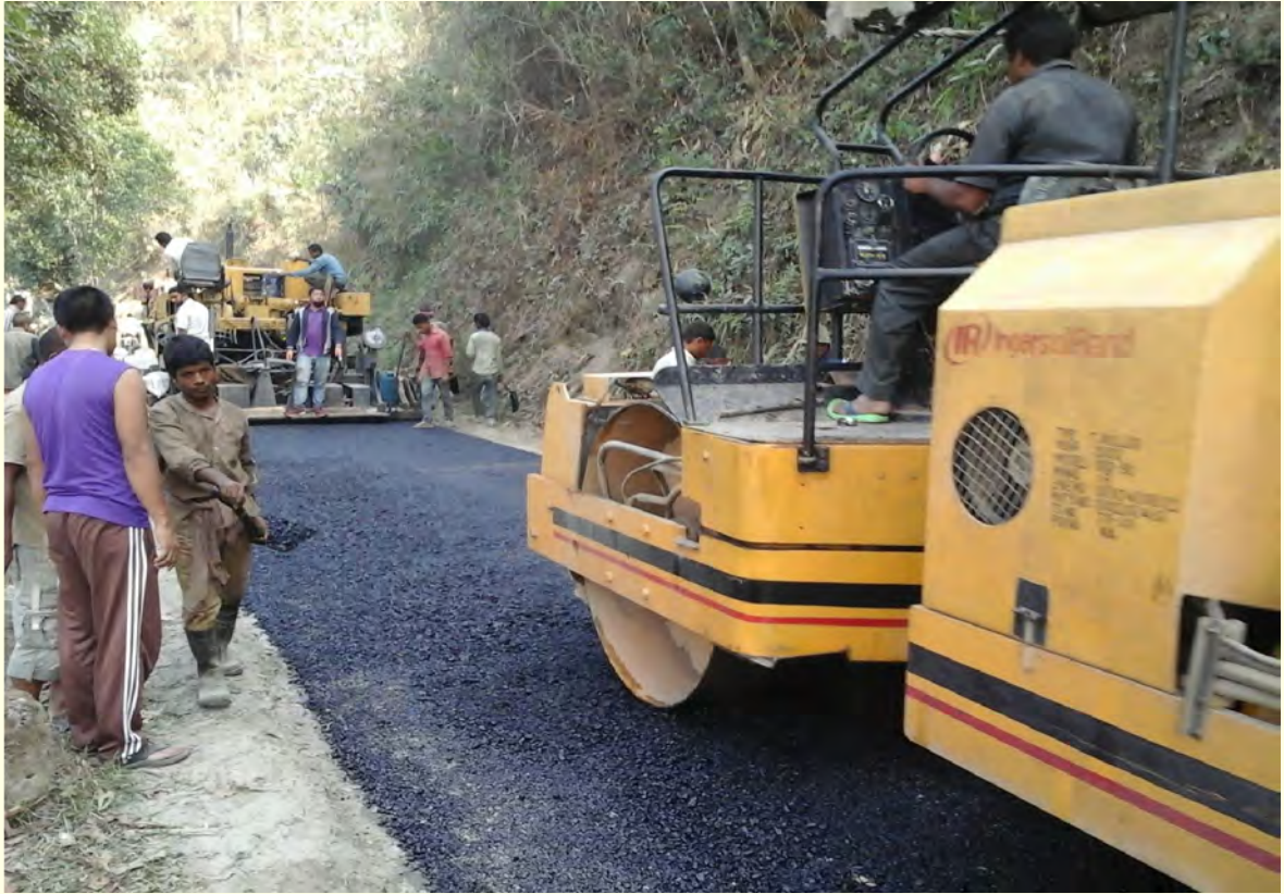
Pavement of W. Phaileng-Marpara Road under NABARD
