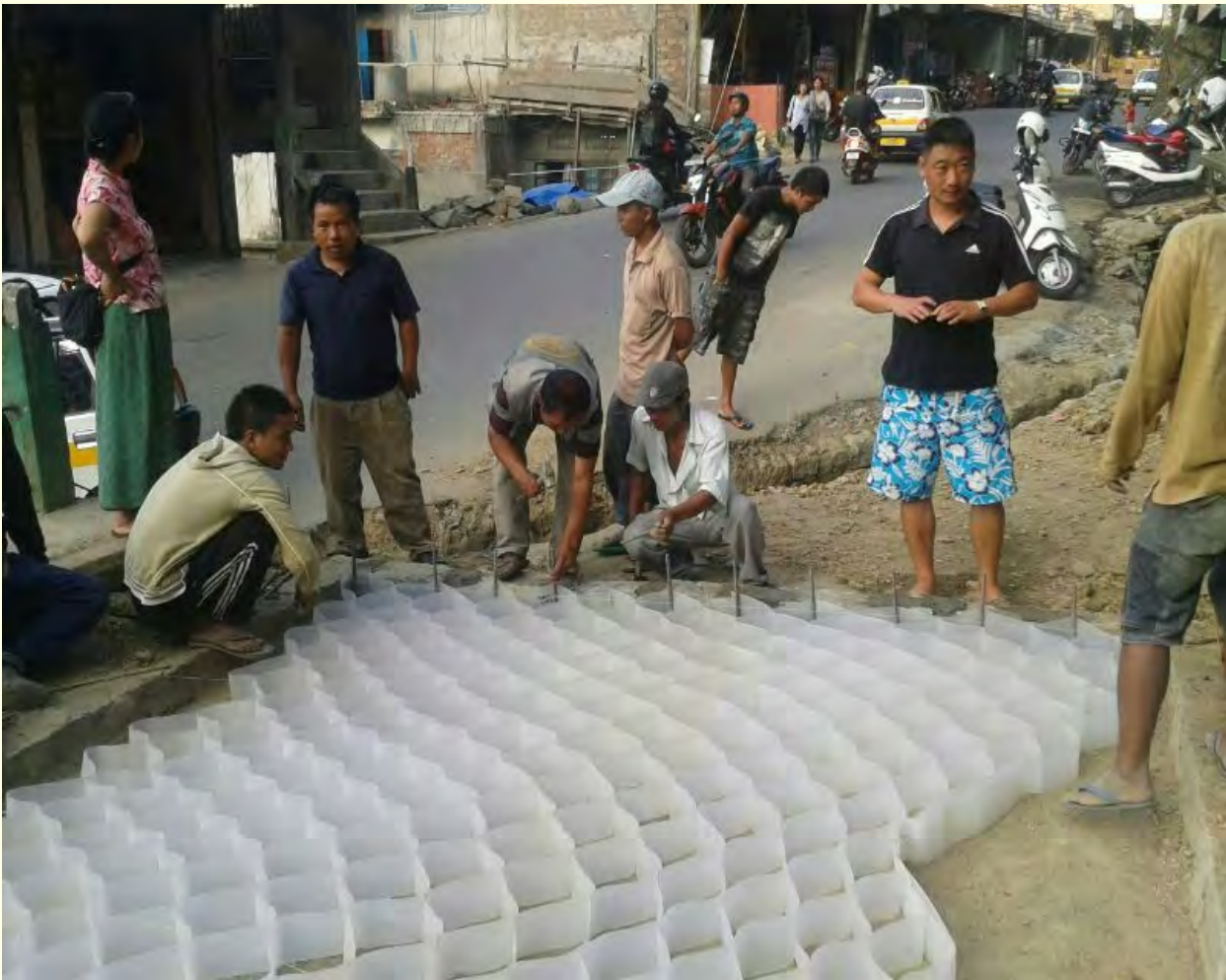
Trial Works PMGSY : Reinforced Cement Concrete Pavement, Vaivakawn to Zotlang Road
