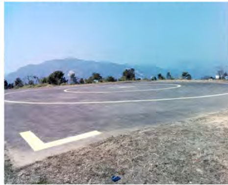
CONSTRUCTION OF HELIPAD AT SERCHHIP UNDER NLCPR
