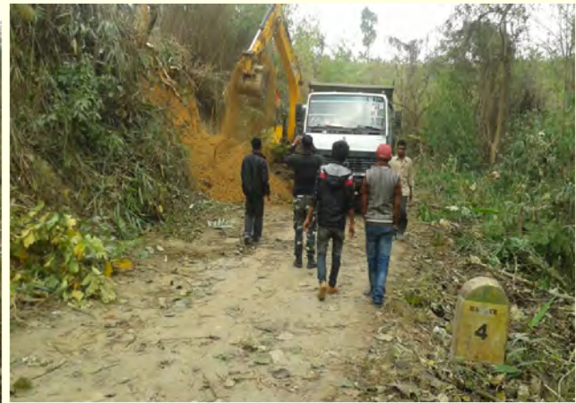
Hill Cutting at Km 1+800, C – C Road
