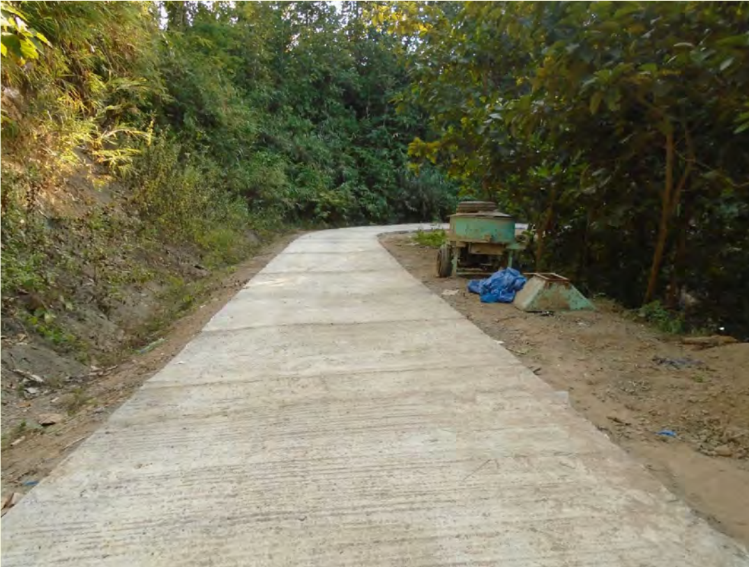
CELL-FILLED CONCRETE ROAD OF PMGSY : Mauzam – Puankhai Road (L=11.120 kms) of Chawngte Area under Tlabung Division
