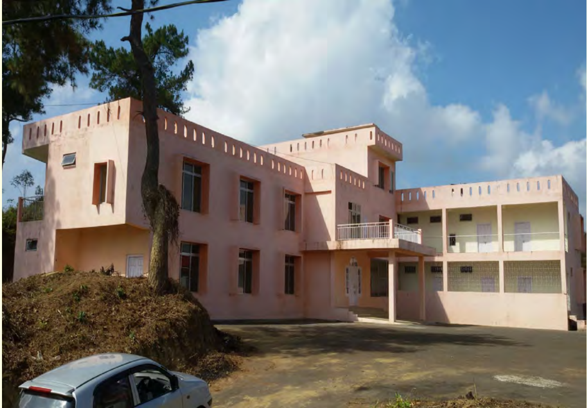
Construction of Tourist Lodge at Serchhip
