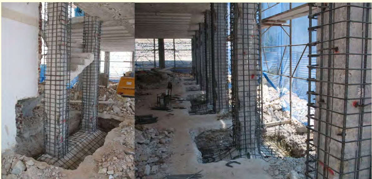
Retrofitting of Printing & Stationery Buildings
