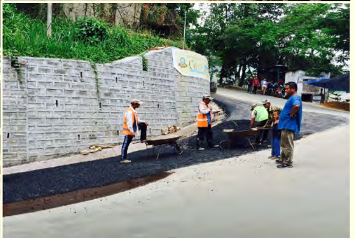
Improvement of works at ITI Junction (1. Grading & Levelling, 2. WBM, 3. Sub Grade Preparation, 4. Pre-mix Carpetting)
