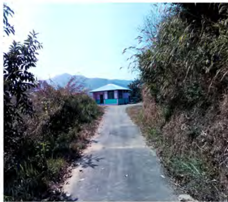
CONSTRUCTION OF HELIPAD ( APPROACH ROAD & WAITING SHED) AT SERCHHIP UNDER NLCPR
