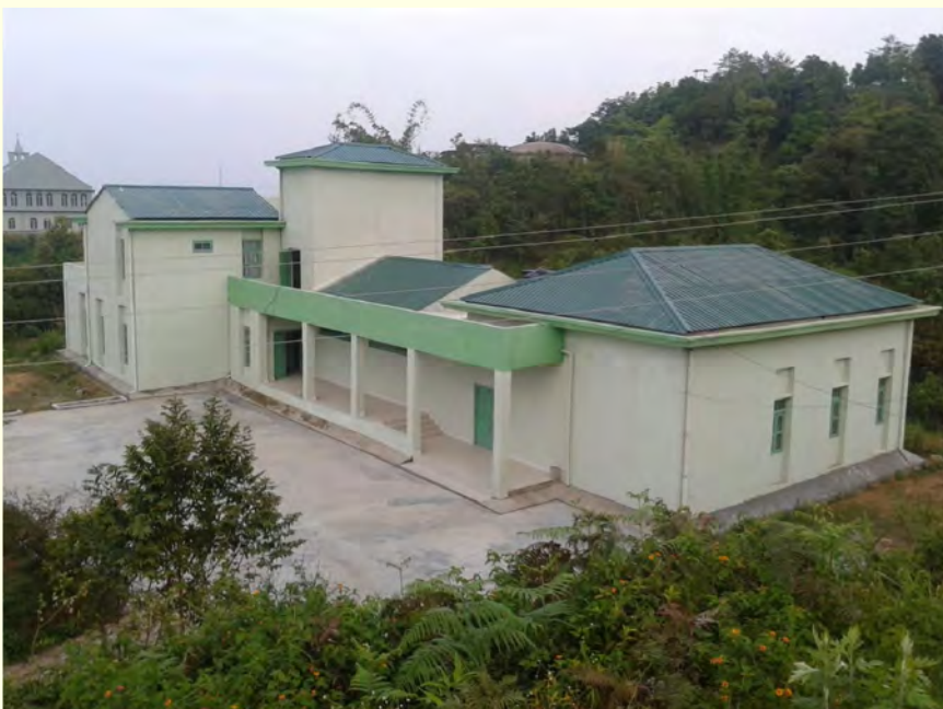
Construction of Auditorium cum Library at Suakphunga's site at Hliappui
