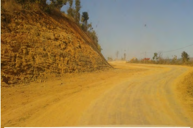
Finished View of Finish View of Formation @ Km 12 + 500, C-Z Road
